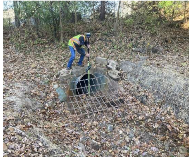
Photo 1 Direction: Facing Downstream
