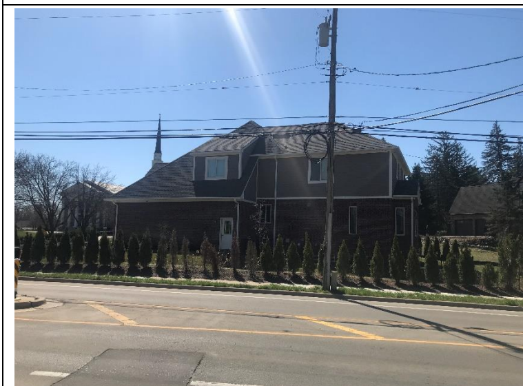
Photo 11. South adjoining residential
