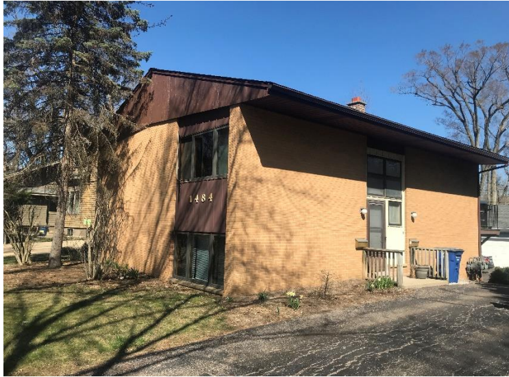
Photo 1. Exterior of 1484 West Liberty near the southern Subject Property Boundary
