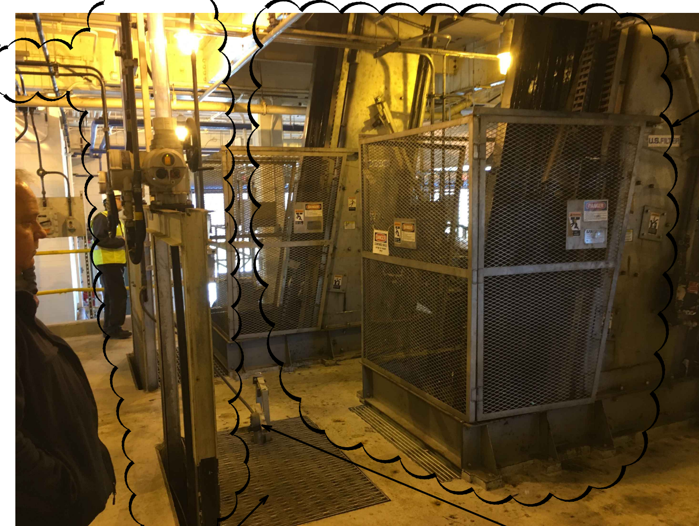
PHOTO 2 - NORTH CHANNEL SCREENS FRONT
