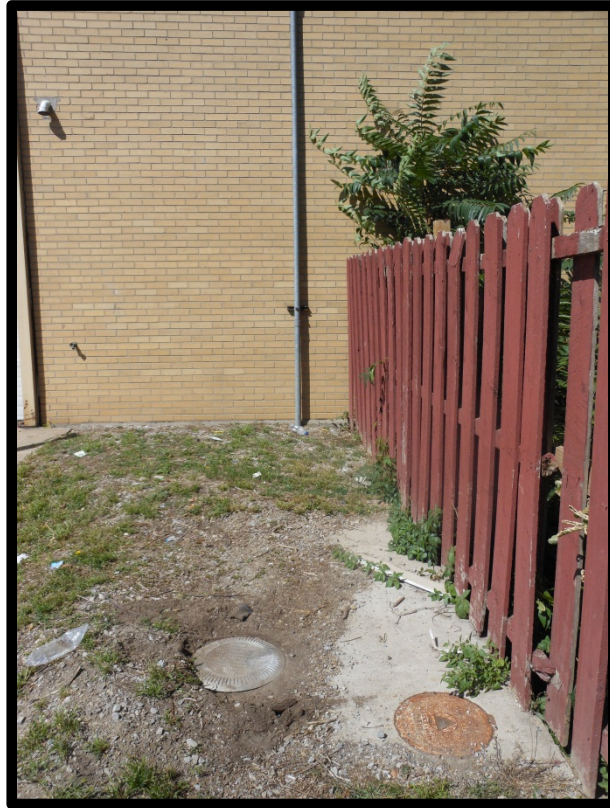
Location of waste oil UST and monitoring well east of maintenance garage
