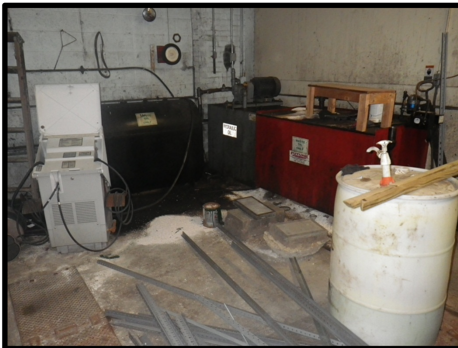
Waste oil, hydraulic oil, and waste anti-freeze tanks located in the maintenance garage
