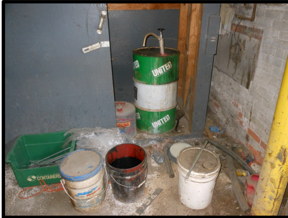
Miscellaneous buckets and drums in the south end of the maintenance garage
