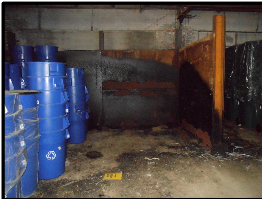
Asphalt storage area in the south end of the maintenance garage
