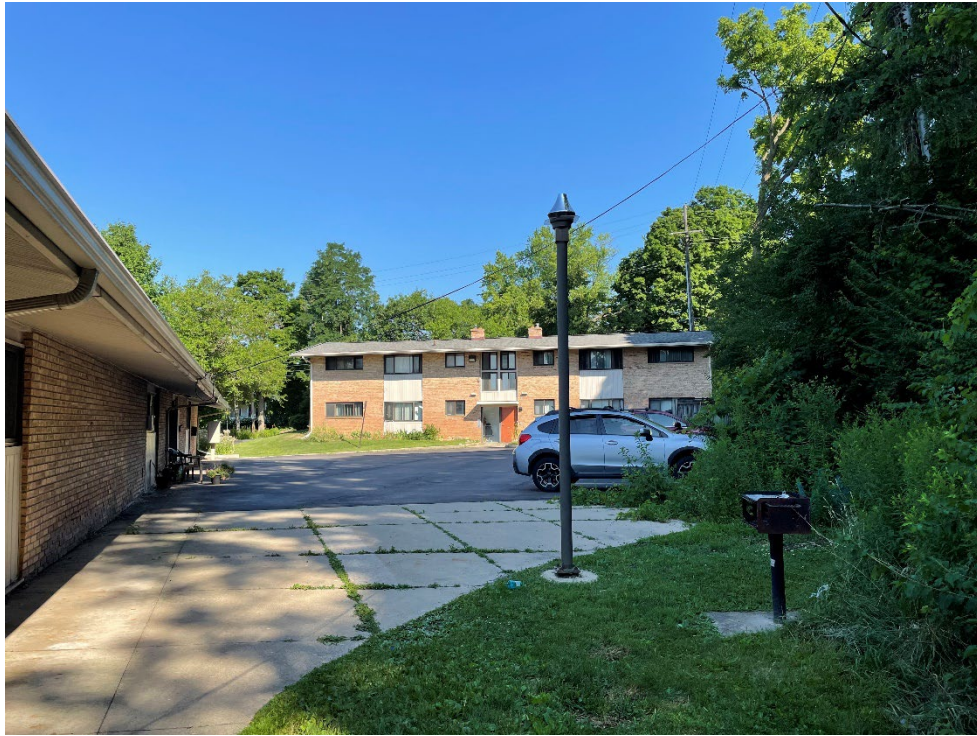
Photograph 7: View looking across the north parking area.
