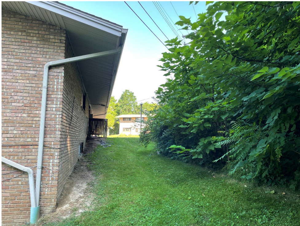
Photograph 8: View looking northwest along the 1506 north building elevation (adjoining heavy vegetation).
