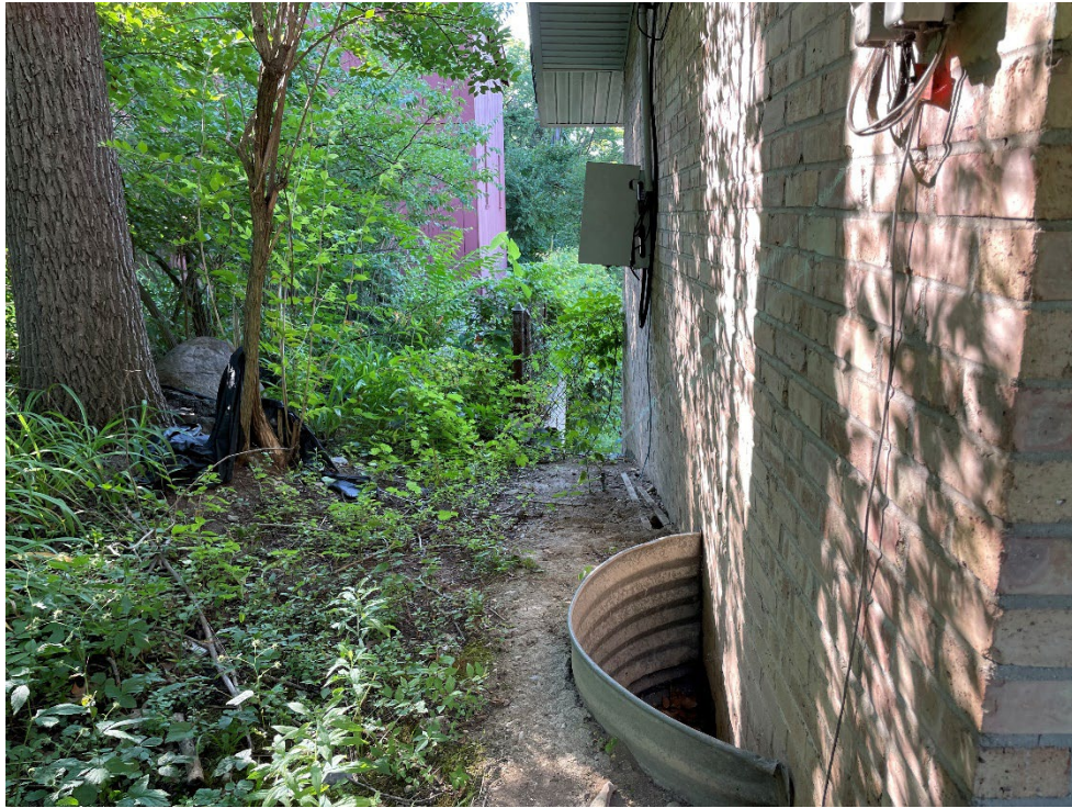
Photograph 3: Side elevation (northeast) of building 1504 (adjoining barn in background).
