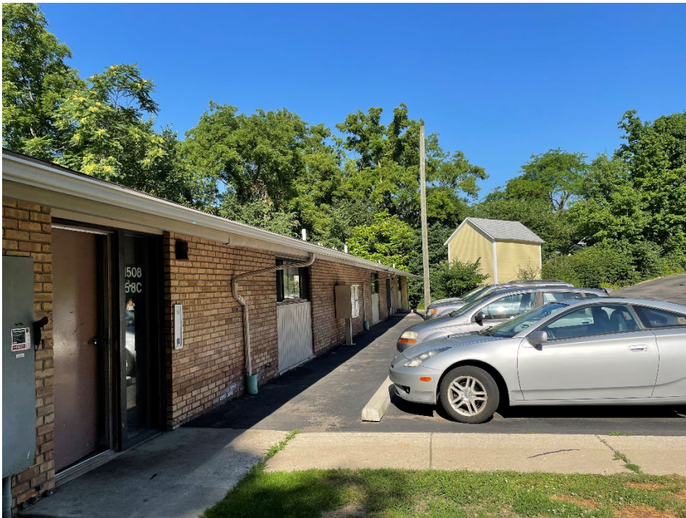
Photograph 12: View of the north building elevation of 1508.
