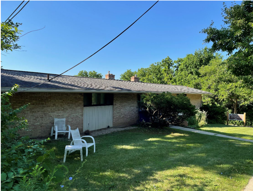
Photograph 2: View of north building (1504) fronting Broadway.
