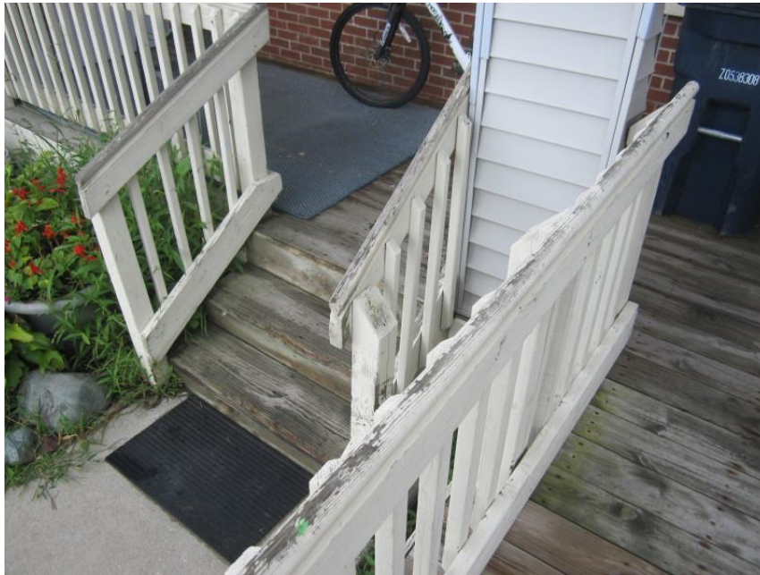
PHOTOGRAPH NO. 7: TYPICAL VIEW OF DECK COMPONENTS
