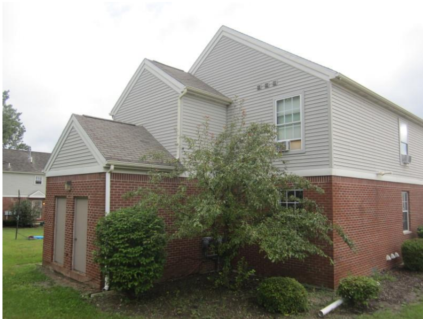
PHOTOGRAPH NO. 2: TYPICAL VIEW OF REAR OF TENANT BUILDING
