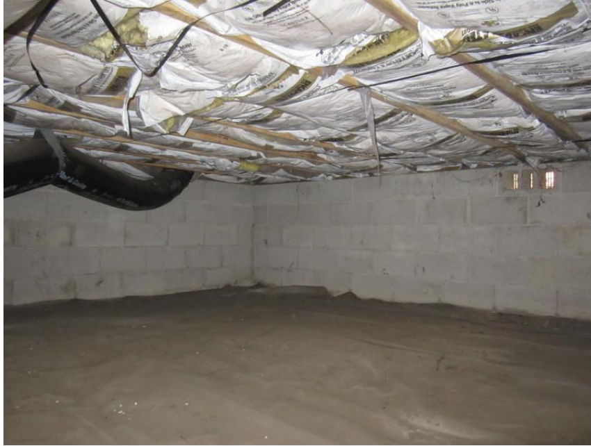
PHOTOGRAPH NO. 13: TYPICAL VIEW OF CRAWL SPACE
