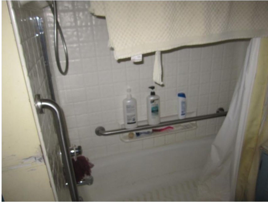
PHOTOGRAPH NO. 11: ADA UNIT BATHROOM
