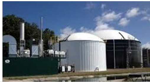
South Campus Digester, Michigan State University
