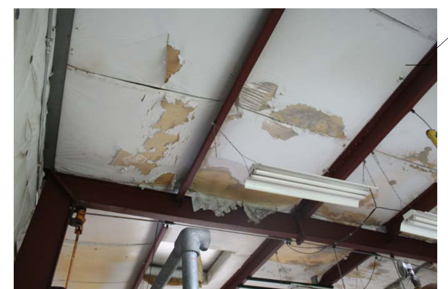
WELL HOUSE 25 - INTERIOR ROOF
