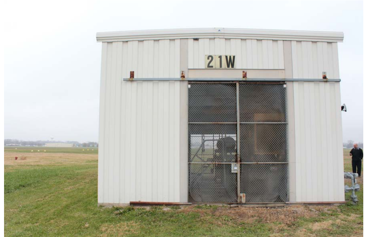
EXISTING WELL HOUSE 21W EXTERIOR
