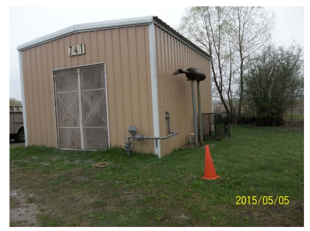
EXISTING WELL HOUSE 741 EXTERIOR
