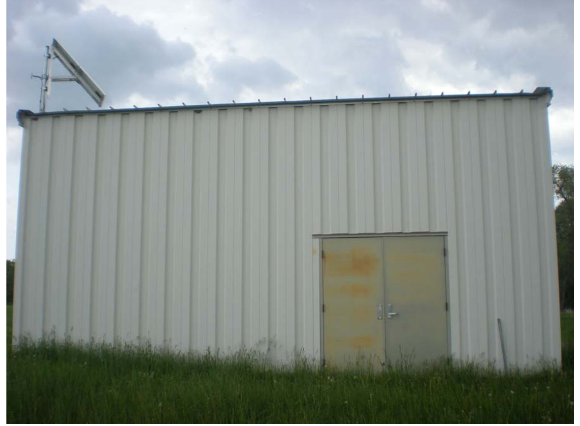
EXISTING WELL HOUSE 21W EXTERIOR
