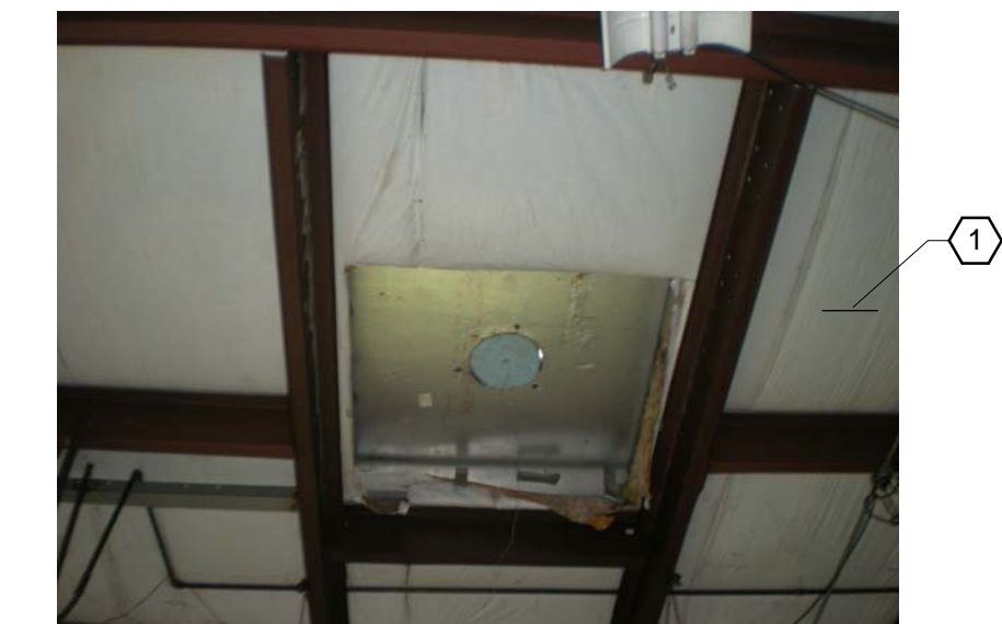
WELL HOUSE 21W - INTERIOR ROOF
