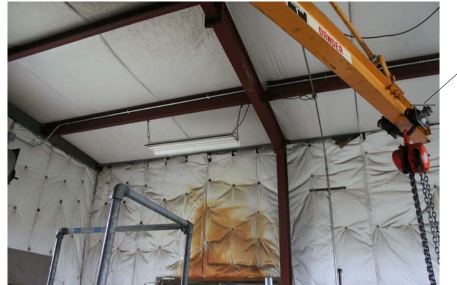
WELL HOUSE 21W - INTERIOR ROOF
