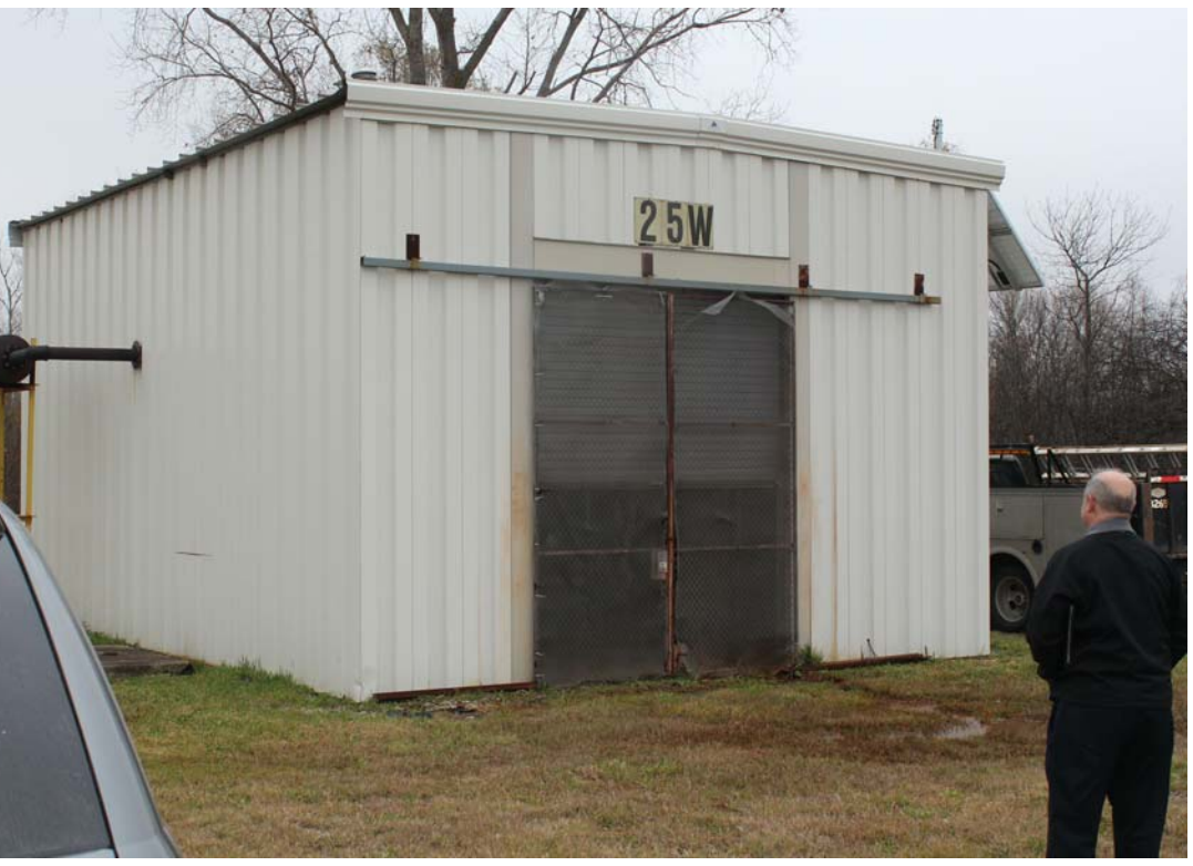
EXISTING WELL HOUSE 25W EXTERIOR
