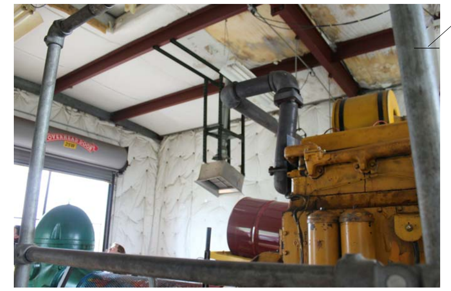
WELL HOUSE 25 - INTERIOR ROOF
