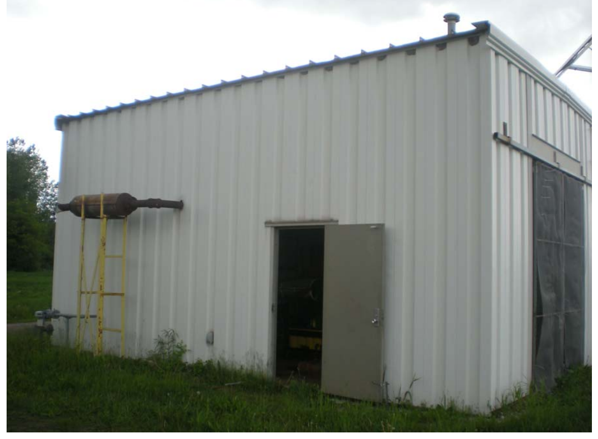
EXISTING WELL HOUSE 21W EXTERIOR
