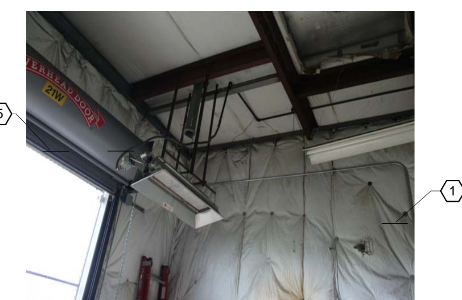
WELL HOUSE 21W - INTERIOR ROOF
