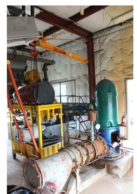
WELL HOUSE 25 INTERIOR
