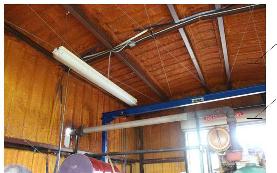
WELL HOUSE 741 - INTERIOR ROOF
