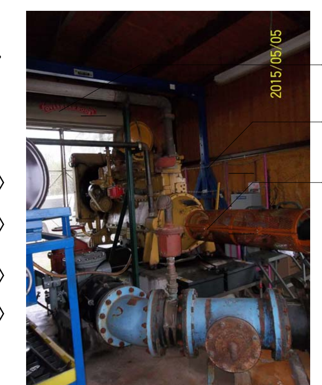
WELL HOUSE 741 INTERIOR
