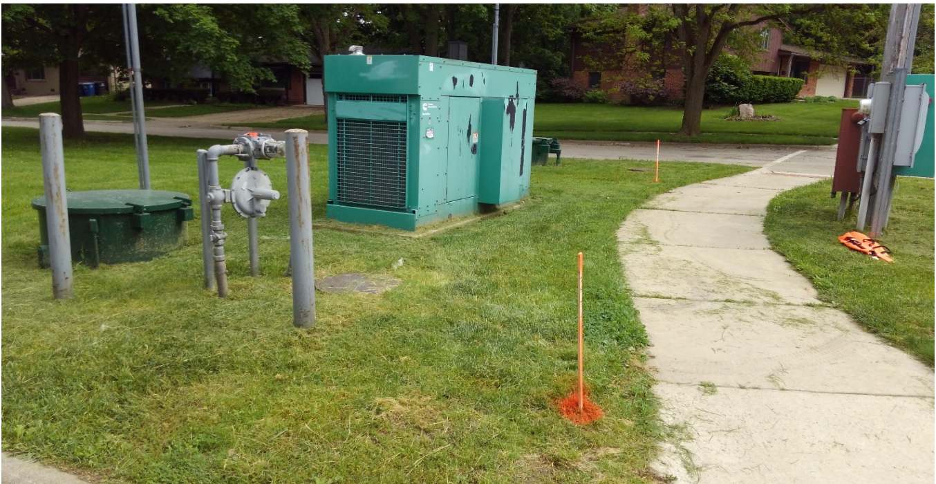
Photo No. 2 - Facing Southeast Towards Boring's B-2 and B-3
