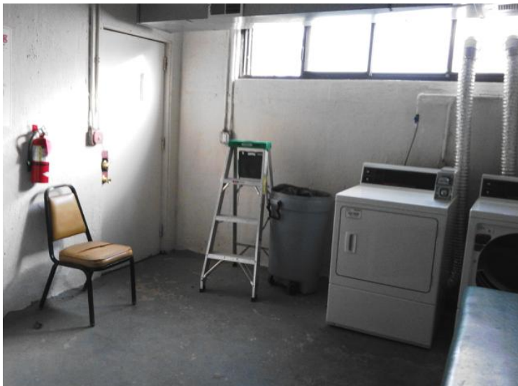
Photo 15. View of laundry room in the basement of 1506 Broadway Street.
