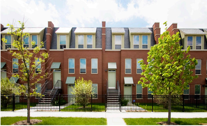
View of 8-Unit Building
