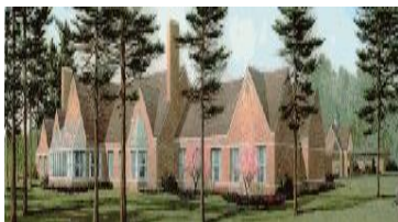
Iosco County Medical Care Facility East Tawas, Michigan
