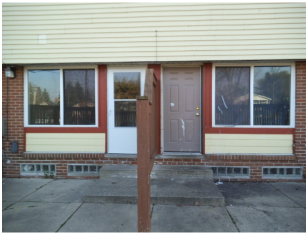
Photo 3: Different door types at complex
