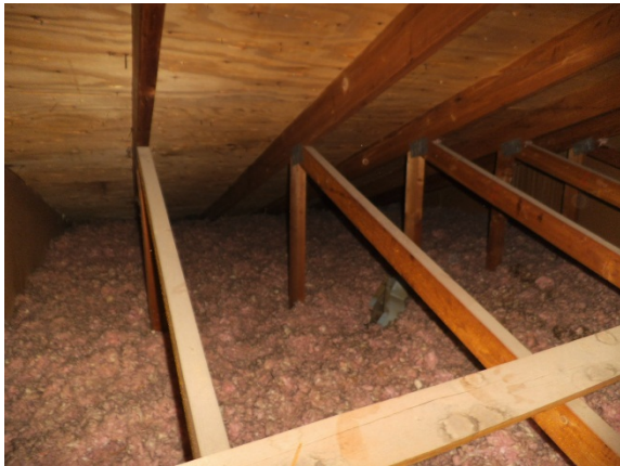
Photo 17: Bathroom Exhaust Fan
