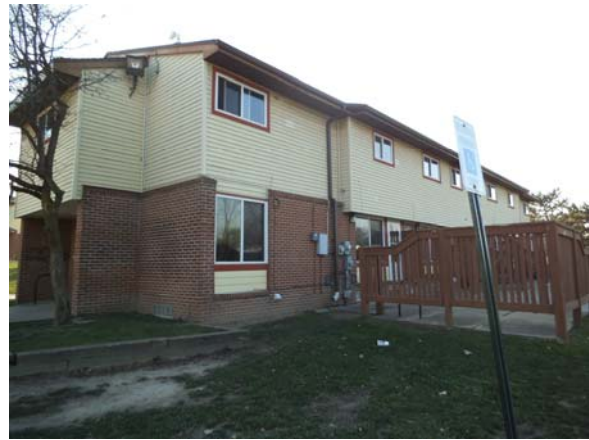
Photo 2: Back exterior of the complex
