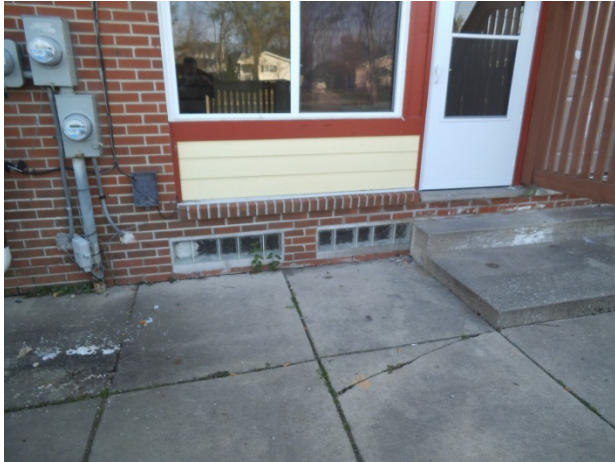
Photo 7: Glass block basement windows
