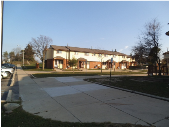
Photo 1: Front exterior of the complex
