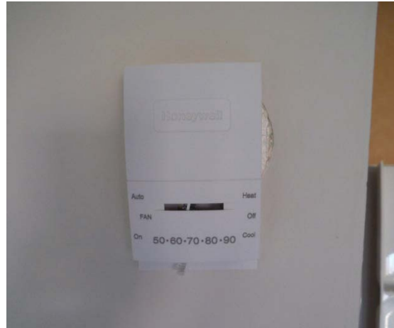
Photo 8: Typical manual thermostat
