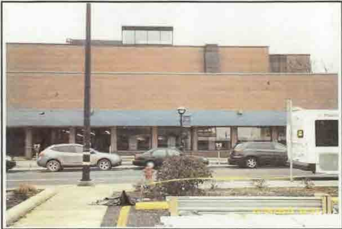
Figure 3.5 View of Ann Arbor Public Library on eastern adjoining parcel.
