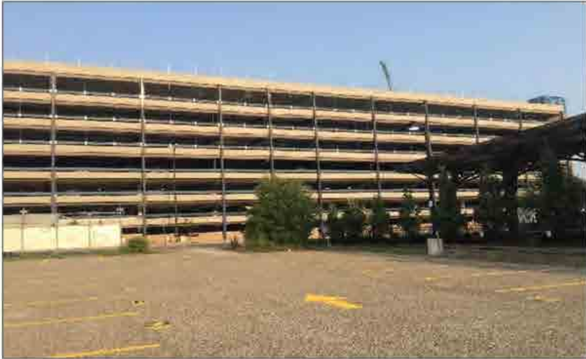
PHOTO NO. 9: View of west-adjointing parking structure.
