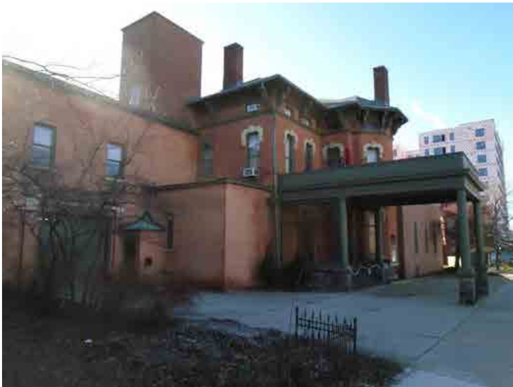
Photo 16: View of the southern adjacent property, Muehlig Funeral Chapel addressed as 403 S. 4 th Ave., looking to the southwest.
