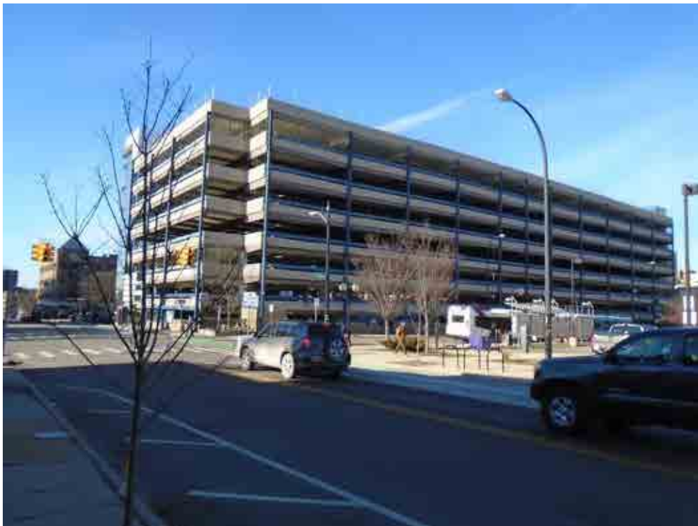
Photo 18: View of the western adjacent property, 4 th and William Parking Structure addressed as 115 E. William Street, looking to the northwest.
