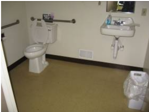
Photo #27: Community center restroom
