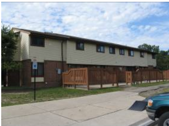
Photo #5: Rear elevation
