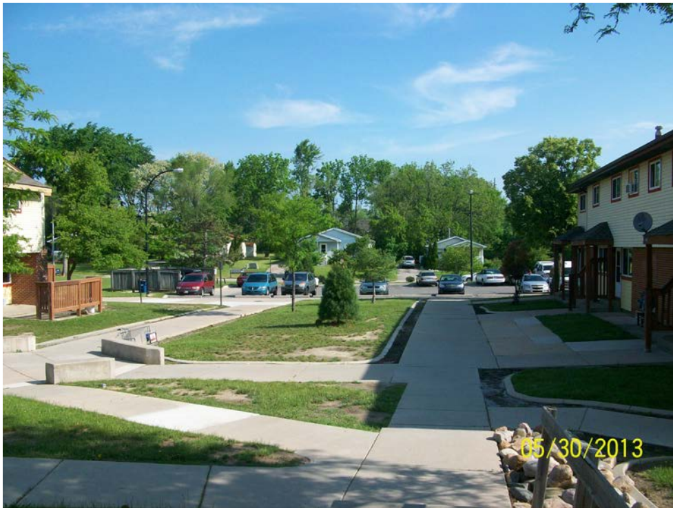
Photograph 4: Central courtyard observed on the Subject Property.
