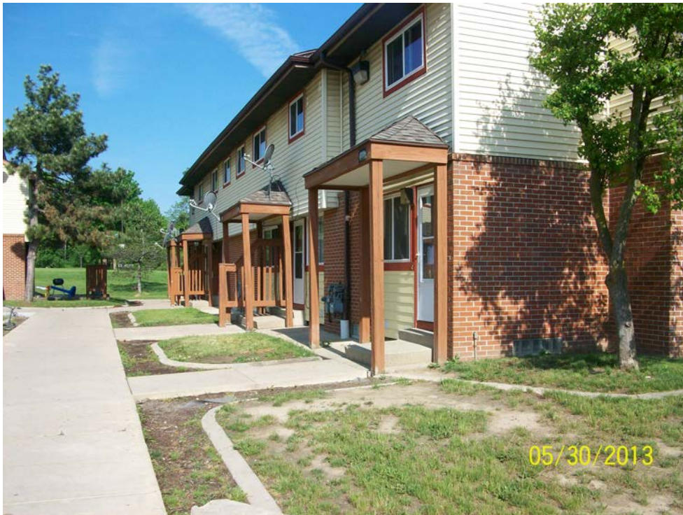
Photograph 2: Typical apartment building observed on the Subject Property.
