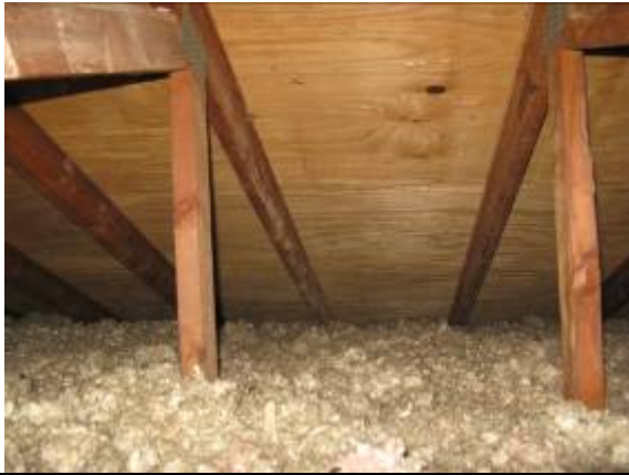
Photo #19: Attic framing
