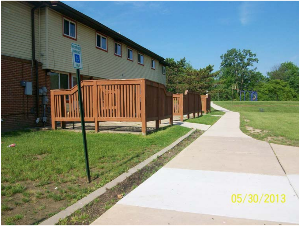
Photograph 3: Typical rear patios with fences observed on the Subject Property.
