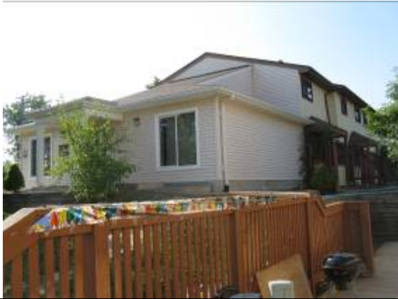
Photo #7: Community center
