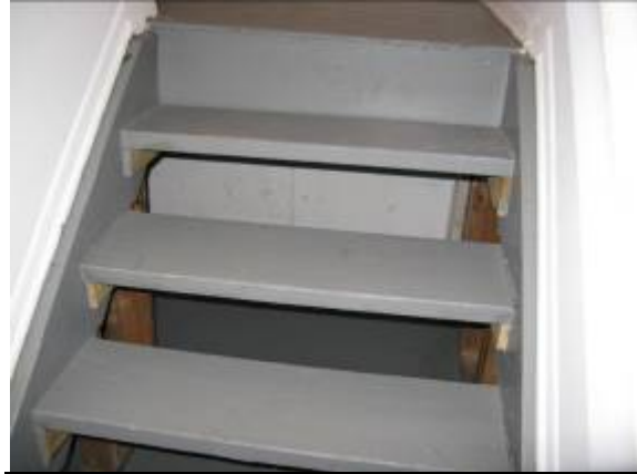
Photo #26: Basement stairs
