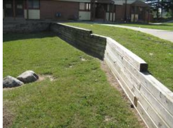
Photo #30: Retaining wall
