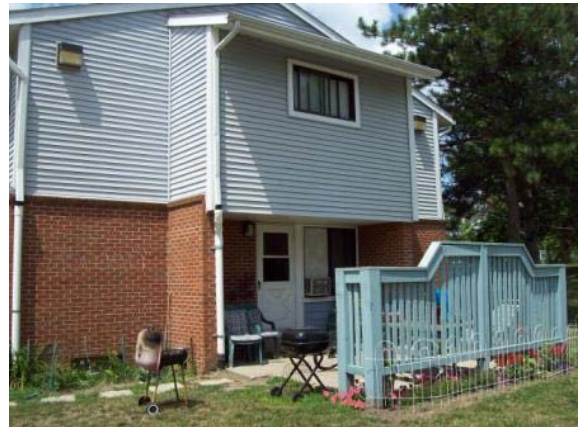
Photo #4: Right side elevation of typical building
