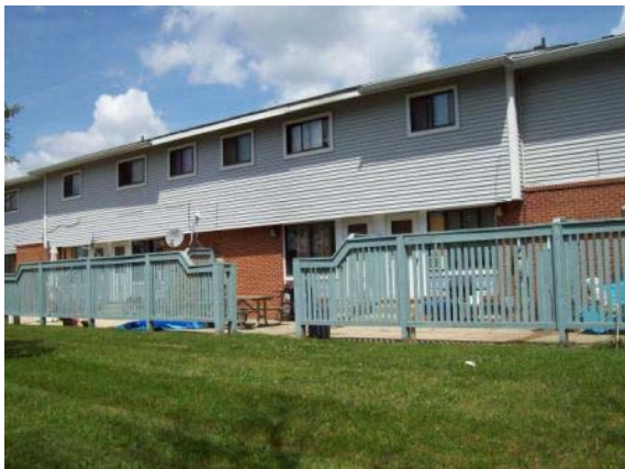
Photo #5: Rear elevation of typical building
