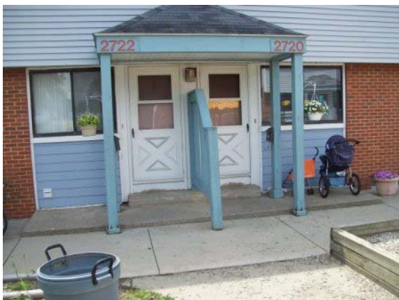
Photo #17: Typical unit entrance and porch structure
