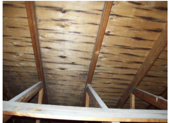
Photo #10: Roof sheathing
