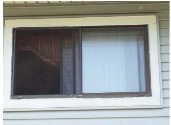
Photo #12: Typical window
