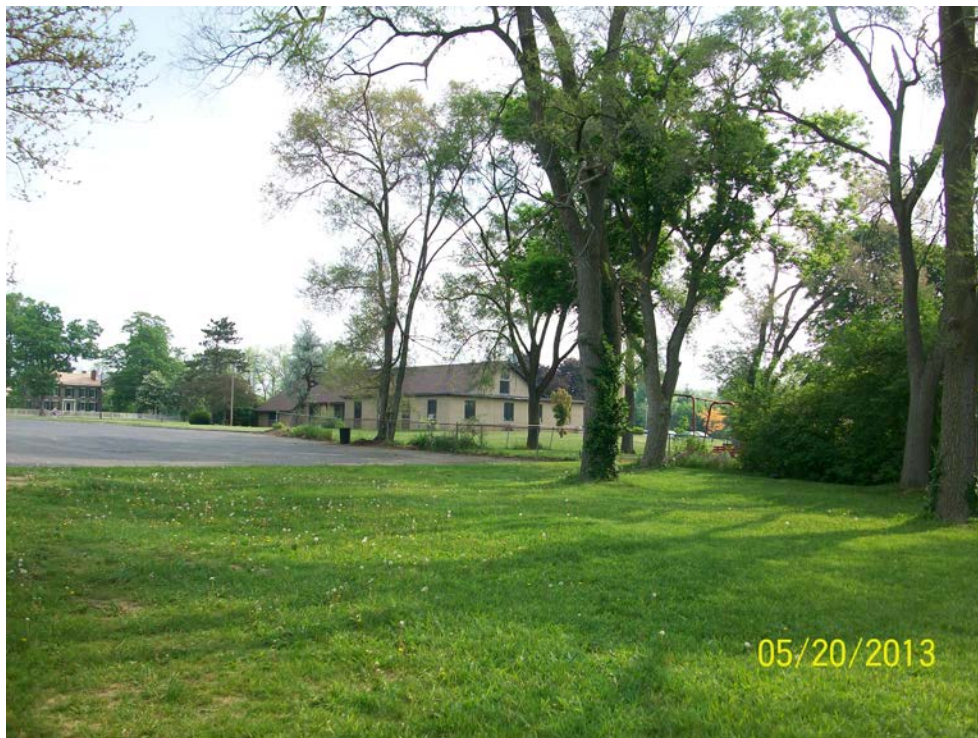
Photograph 14: North adjoining church, view facing northeast.
