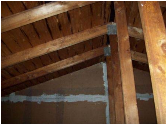
Photo #9: Attic construction
