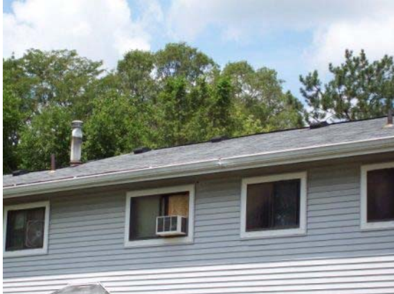
Photo #7: Roof overview
