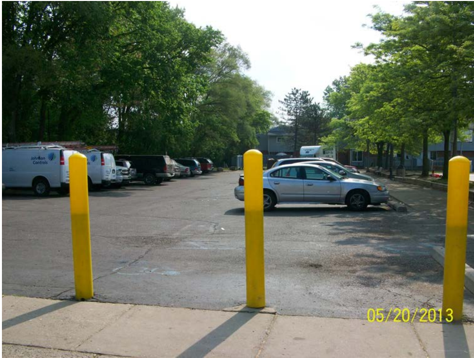
Photograph 5: Asphalt parking lot on the Subject Property.
