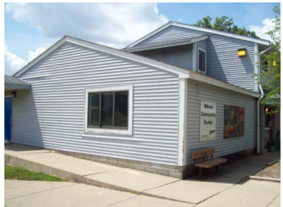
Photo #6: Community center
