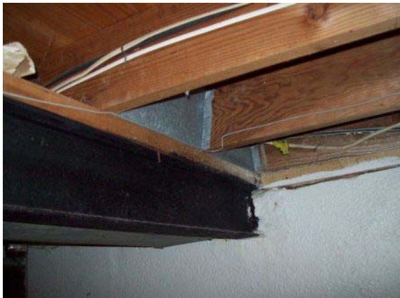
Photo #11: Floor construction and basement wall
