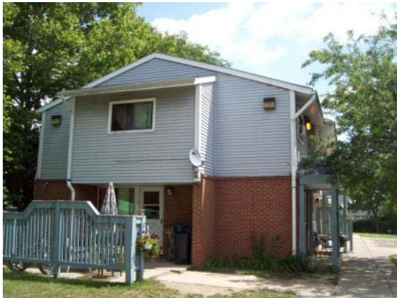
Photo #3: Left side elevation of typical building
