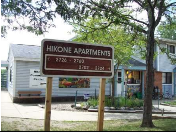
Photo #1: Property signage
