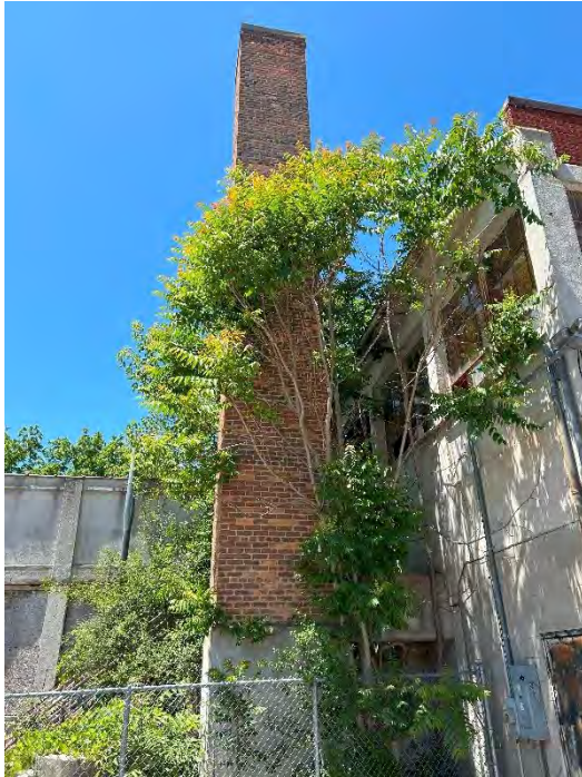
Photo 1: Photo of Chimney, Flue and Existing Building.
