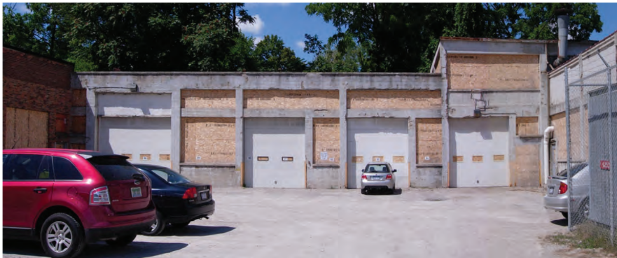
2012 photo of the 1928 addition showing the steel sash covered with OSB board for security.
