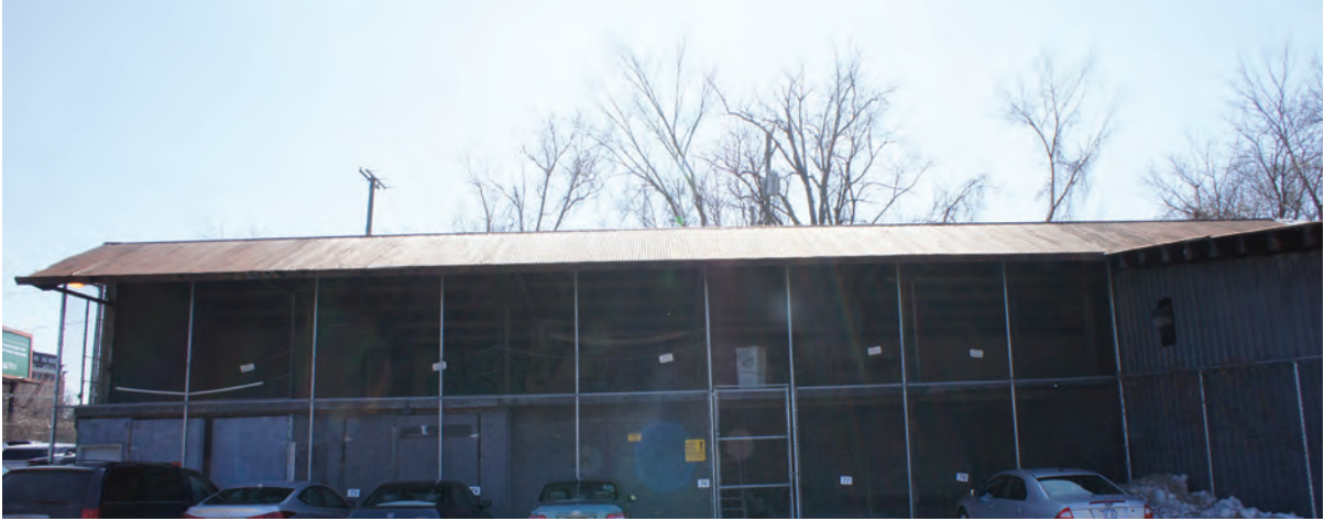
2012 photo of the 1934 CWA Welfare steel shed addition.
