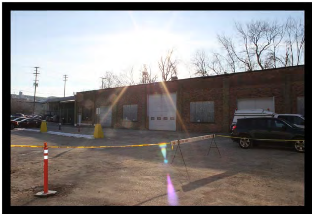
Looking south at the South Garage
