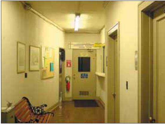
Second floor corridor
