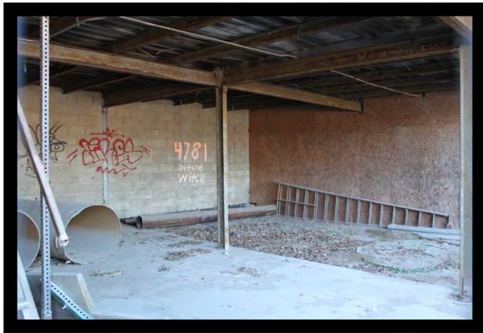
Inside the storage area of the South Garage
