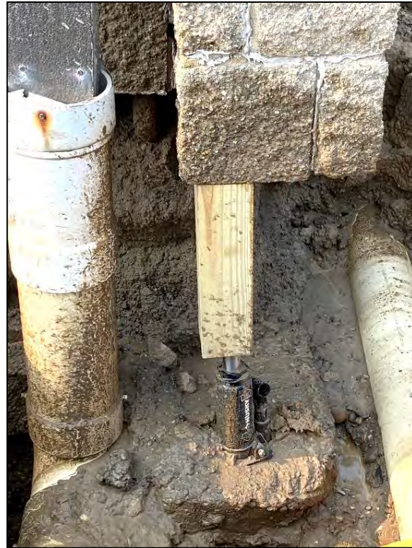
Photo 10: Hydraulic Jack and 4x4 On Concrete Foundation
