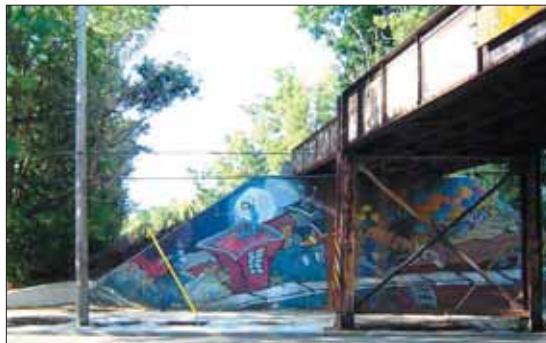
AARR tressle bridge
