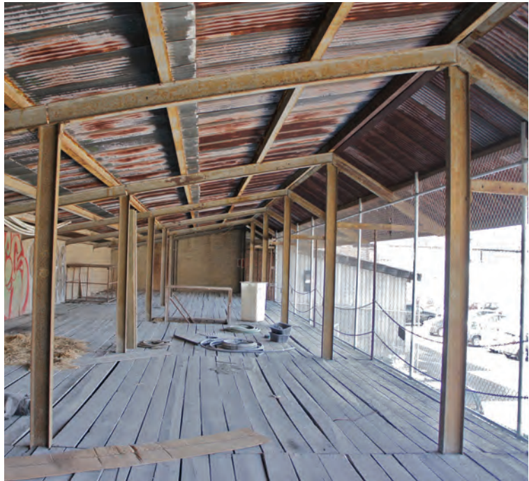
Interior second floor 2013 photo of the 1934 CWA Welfare steel shed addition.
