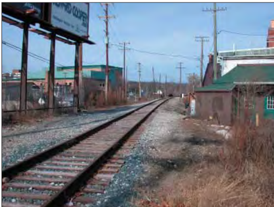
AARR tracks looking North to the embankment
