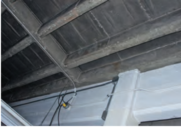
Steel pan formed roof deck. The floor system is similar.
