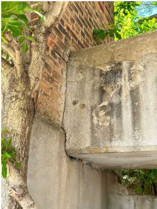
Photo 2: Existing Concrete Flue Bearing on Concrete Base.
