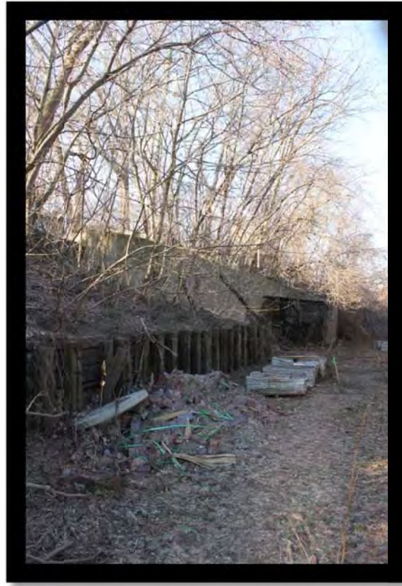
Looking west at the area behind the South Garage
