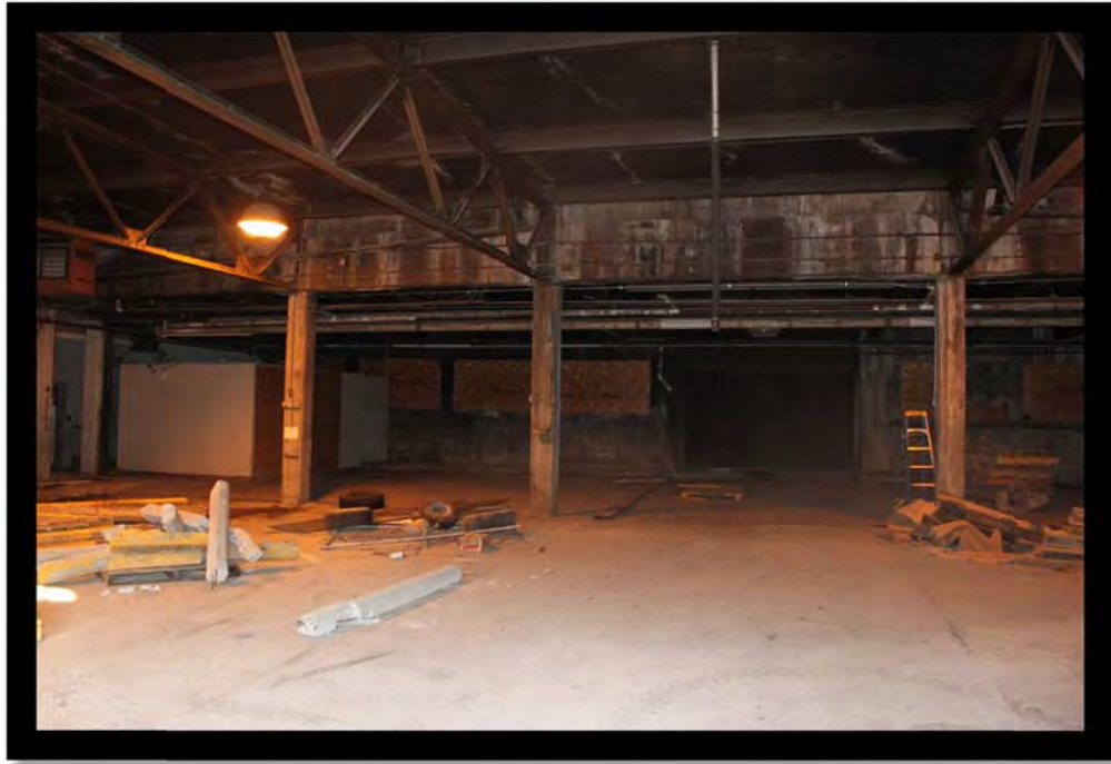
Looking north inside the North Garage
