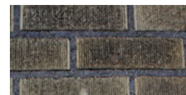
Buff "rug faced" brick on pilasters.
