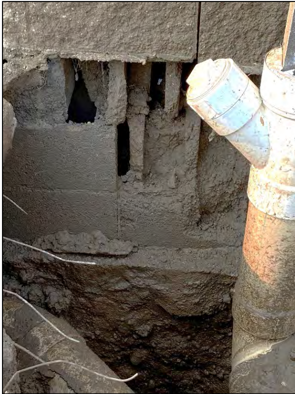
Photo 9: Concrete Foundation Below Plain CMU
