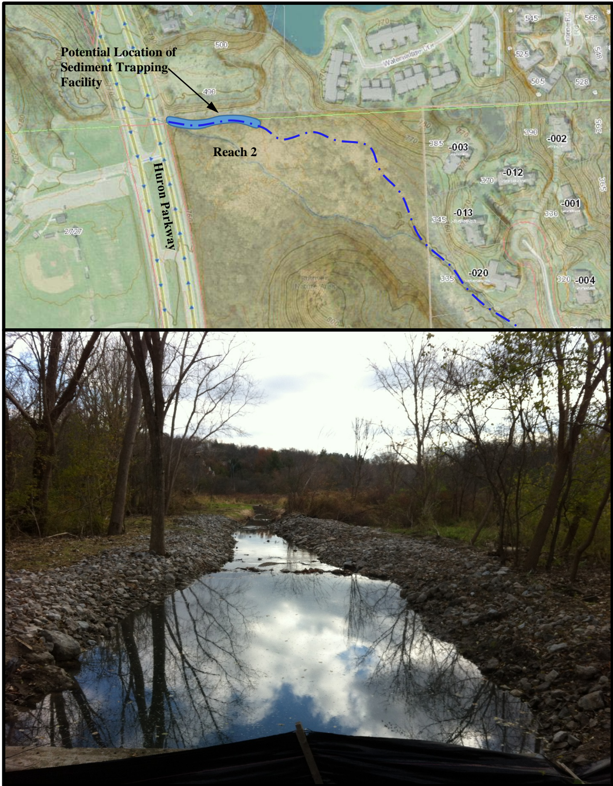
Figure 15. Location of Reach 2 sediment trap-and-removal (top) and photo (bottom) of 2012 sediment removal area.
