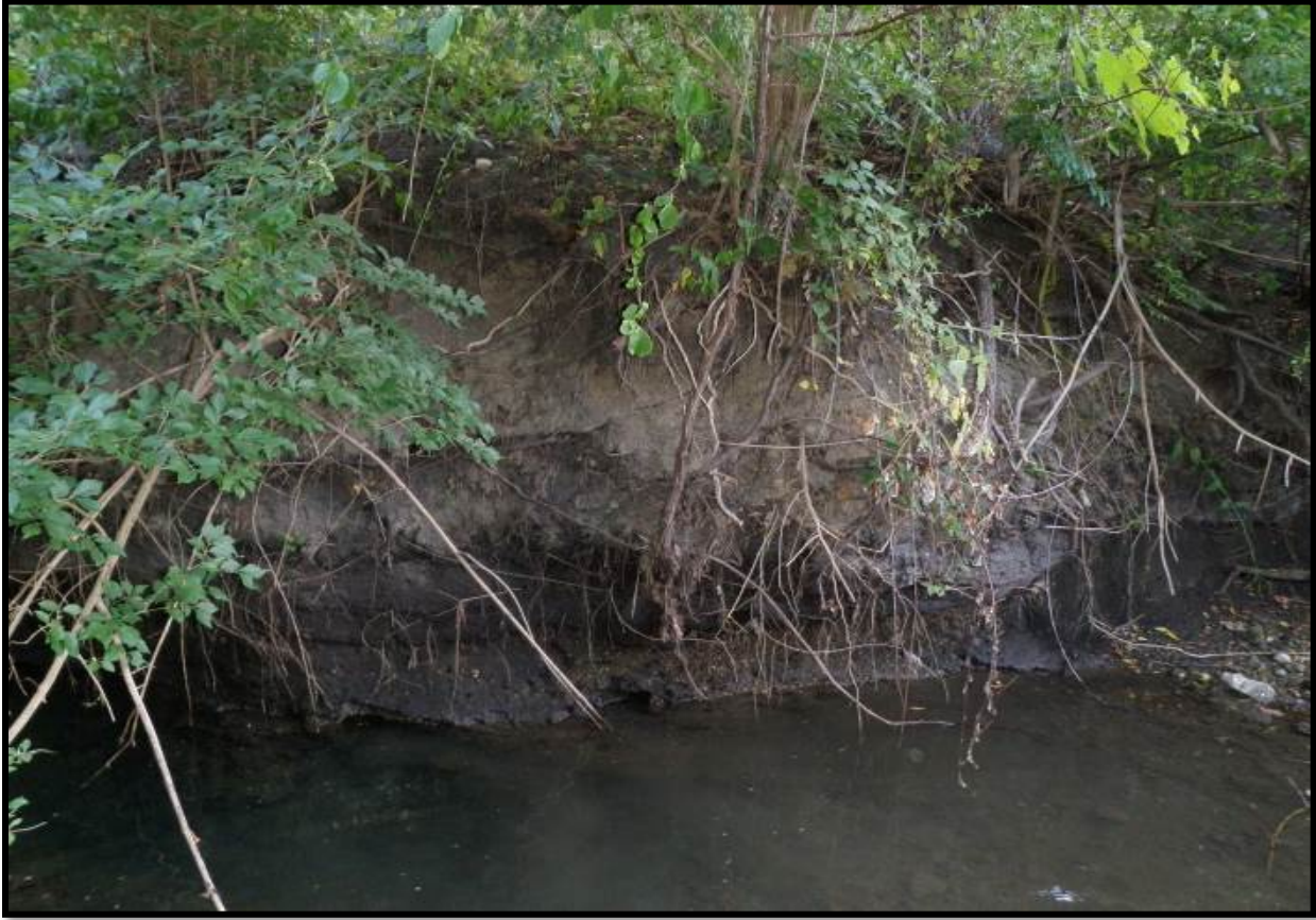
Figure 5. Severe bank erosion in Reach 6.
