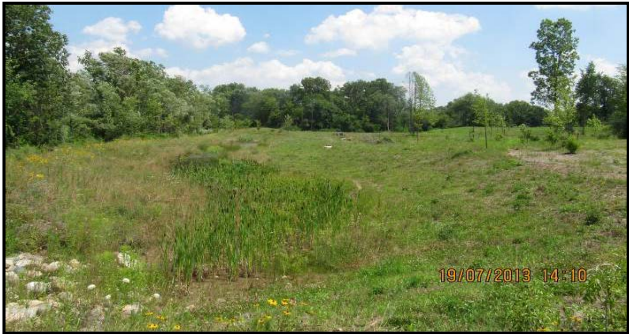
Figure 14-1. County Farm Park sediment forebay (foreground) and stormwater detention basin (background), Ann Arbor, MI.
