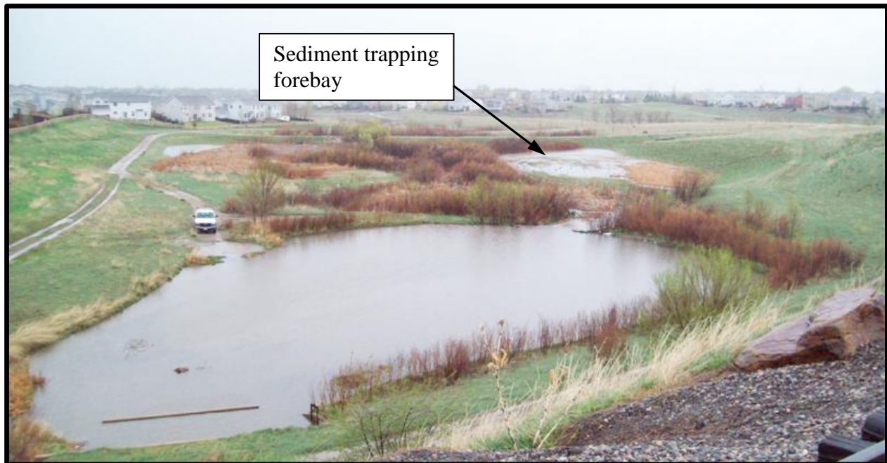
Figure 14-2. Regional Stormwater Detention Basin with Sediment Trapping Forebay, Northglenn, CO.
