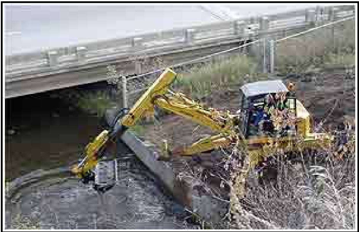
Figure 16. Sediment trap maintenance in Duluth, MN.
