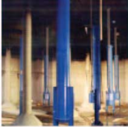
Figure 2.3 - Cannon Mixer Installation
