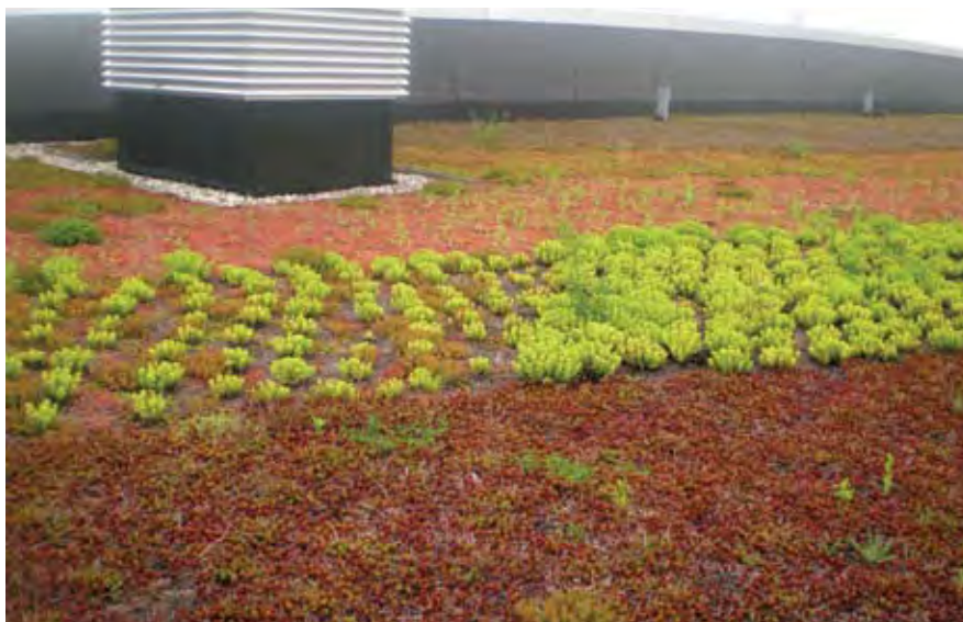
Green roof with sedum at Lawrence Technological University's Taubman Student Services Center
