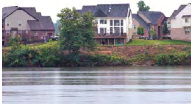
Combination of established and new riparian vegetation Source: Huron River Watershed Council
