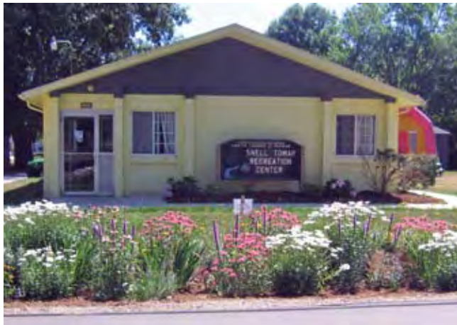
Towar Rain Garden Drains
