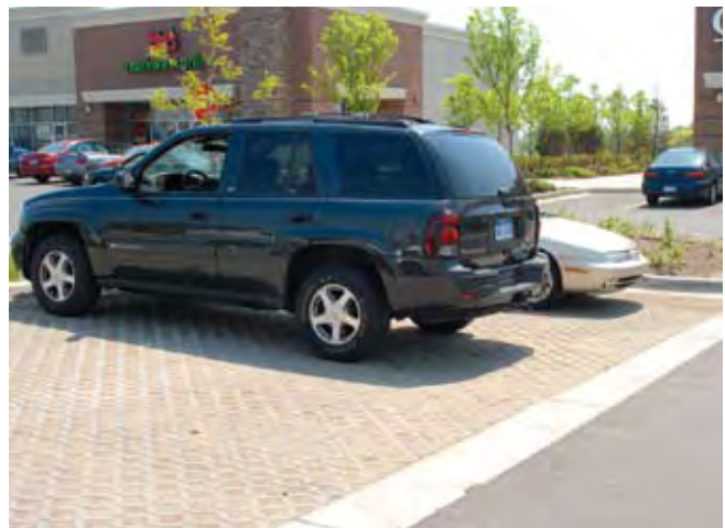
Permeable paver blocks at Fairlane Green shopping center, Allen Park, MI
