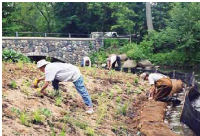
Rouge River streambank stabilization, City of Birmingham, MI
