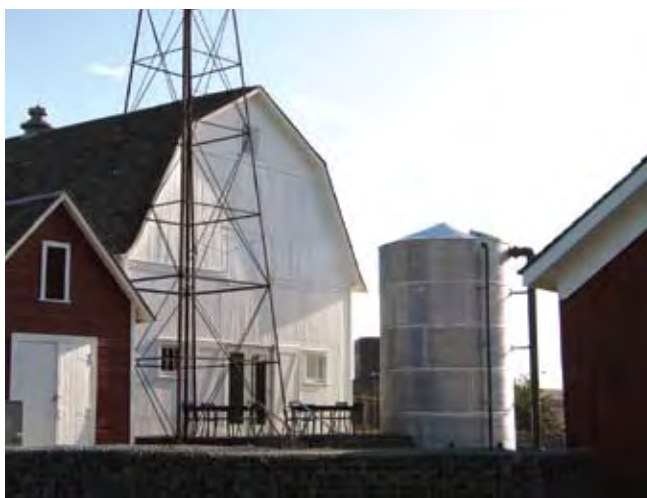
Cistern at Kresge Foundation
