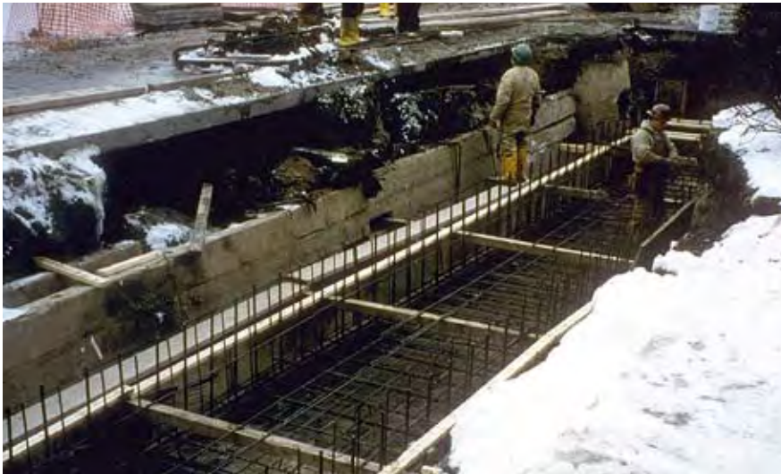
Installation of a sand filter
