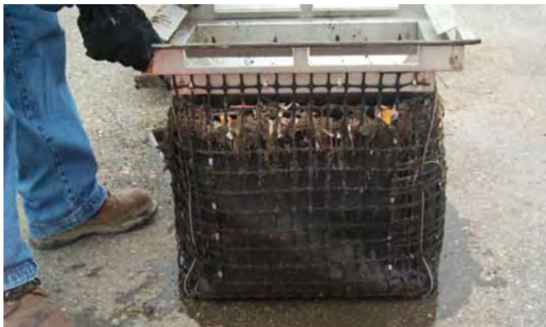
Filtration insert with debris in St. Clair Shores, MI Source: Environmental Consulting & Technology, Inc.
