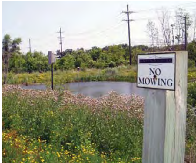
Detention basin with a no mow buffer in West Bloomfield Township, MI
