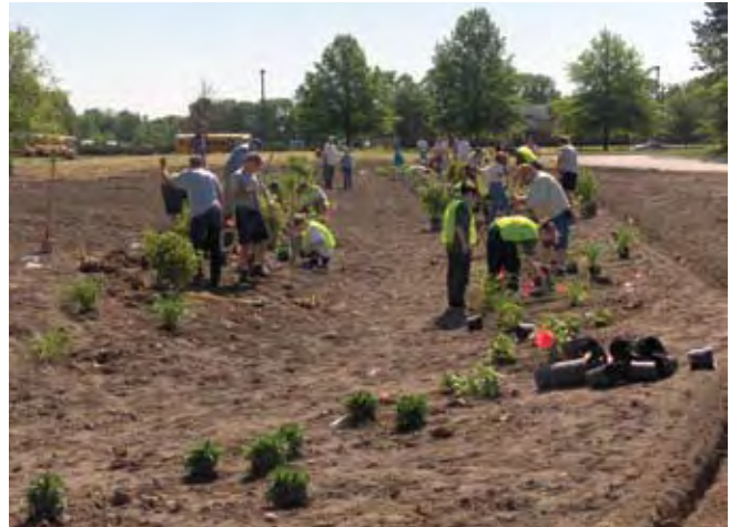
Installing bioswale vegetation at Macomb County Public Works Office.
