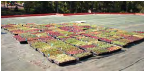
Plugs prior to planting extensive vegetated roof
