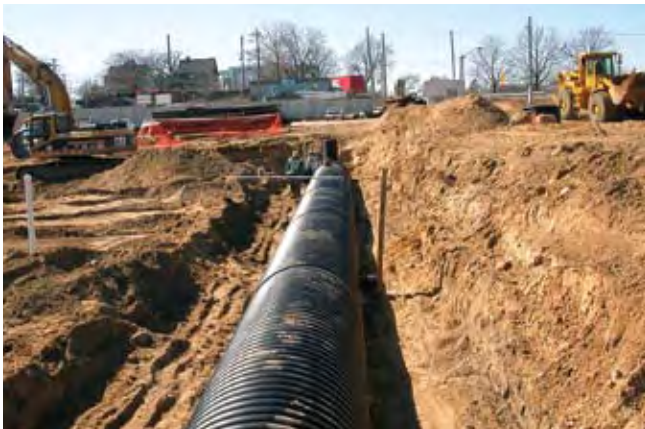
Subsurface infiltration system
