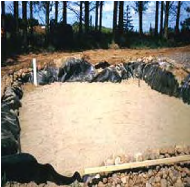
Sand filter under construction
