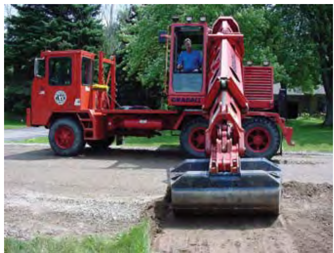
Evaluate roadside ditching operations to retain existing vegetation where possible.
