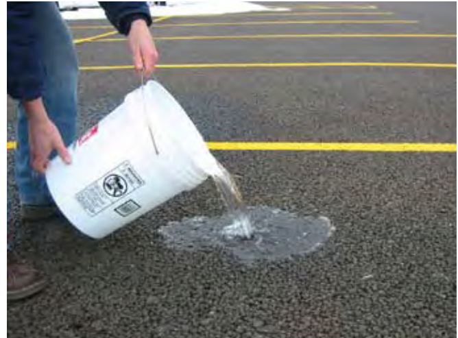
Water on Porous Asphalt Source: Fishbeck, Thompson, Carr & Huber, Inc.
