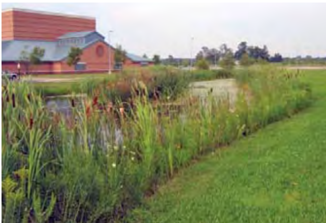
Constructed wetland at Okemos High School Source: Tetra Tech
