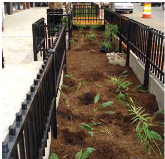
Street view of rain gardens in planter boxes in Lansing, MI.
