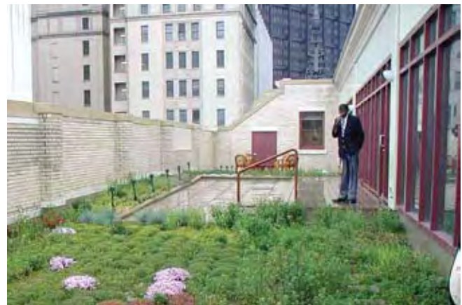
Extensive vegetated roof cover retrofit incorporating a patio for viewing
