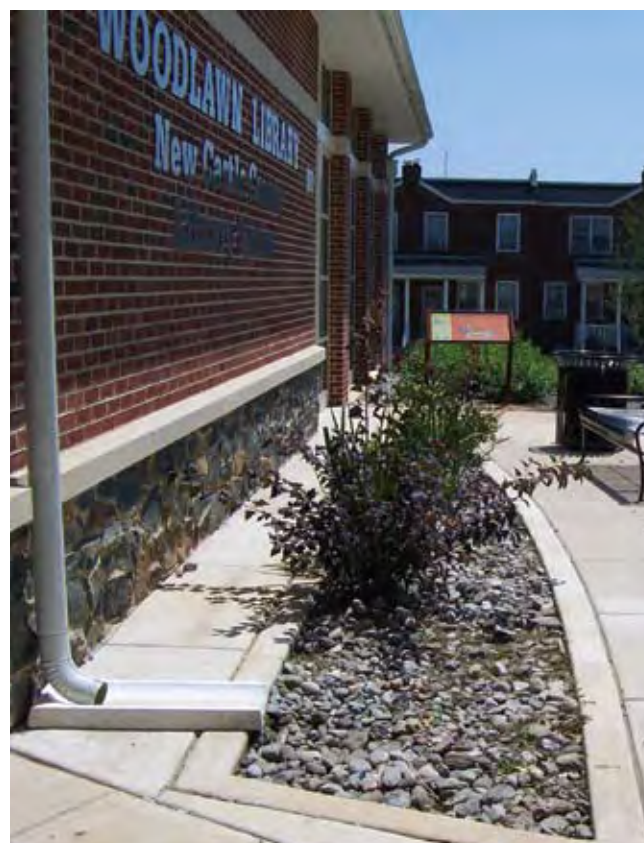
Example of Infiltration Planter Box
