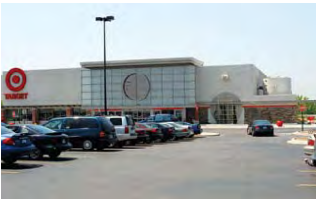
Retail center that incorporated a cistern and rain garden.
