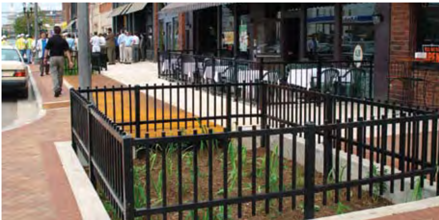
Bioretention in planter box along Michigan Avenue, Lansing, Michigan
