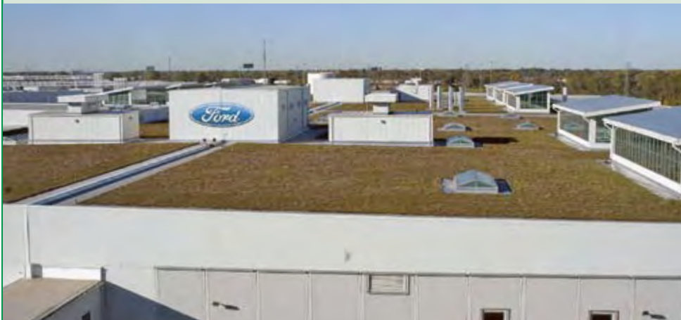
Green roof at the Ford Rouge Plant in Dearborn, MI
