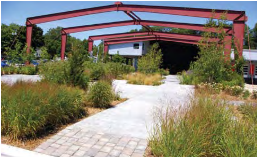
Center for the Arts stormwater disconnection
