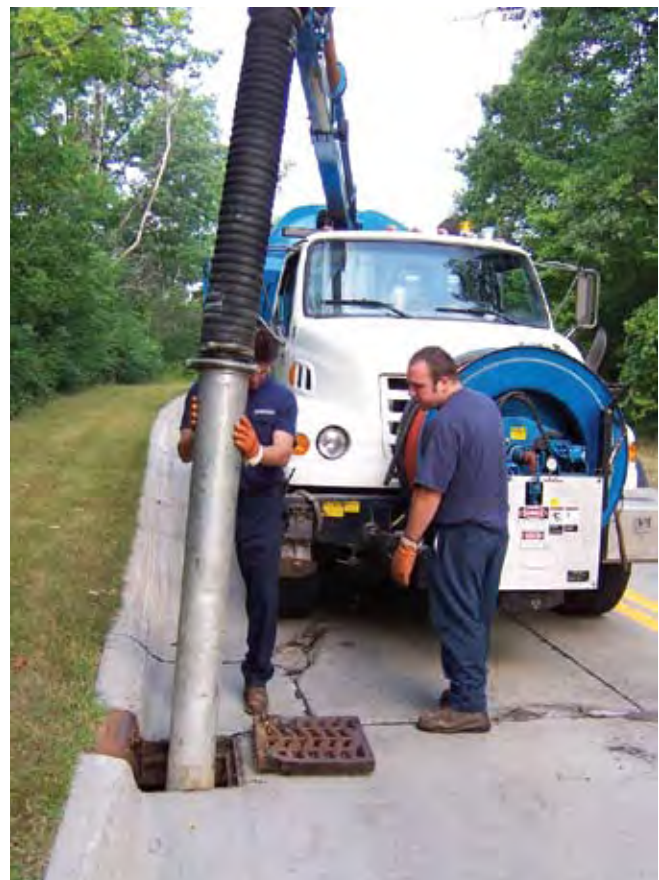
Catch basin cleaning in Bloomfield Township, MI
