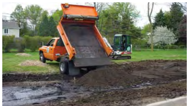
Preparing bed with planting soil
