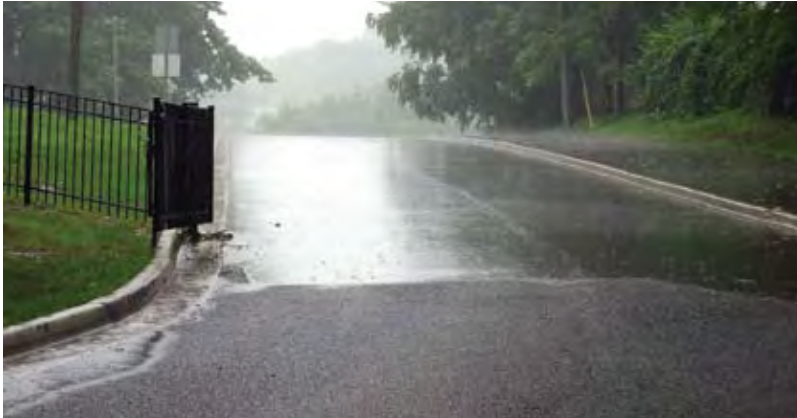
Pervious asphalt at Willard Beach Park
