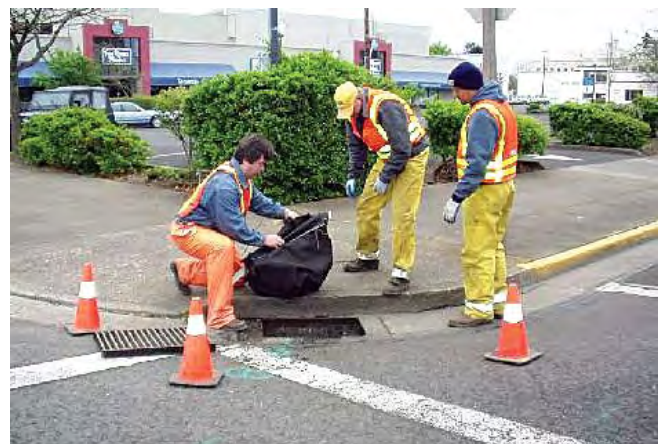
Installing a bag type catch basin insert
