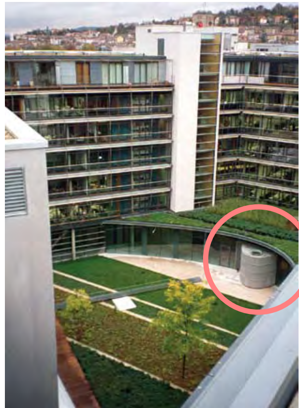
Vertical storage units for vegetated roof plaza maintenance are common in Germany
