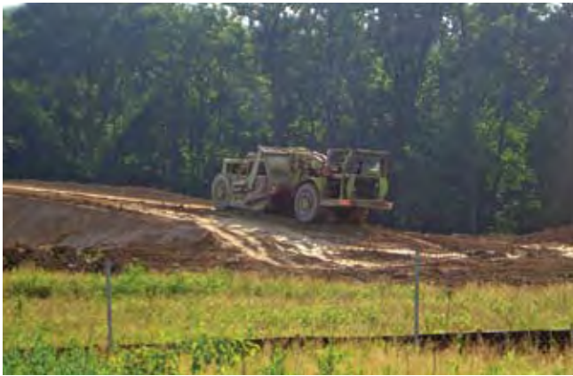
Construction site disturbance showing grading and soil compaction
