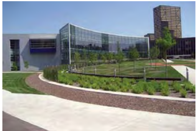
Bioswale at Taubman Center, LTU Campus
