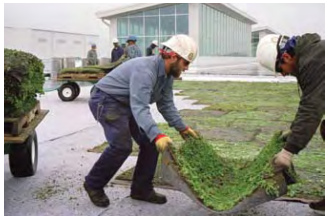
Installation of green roof at the Ford Rouge Plant in Dearborn, MI
