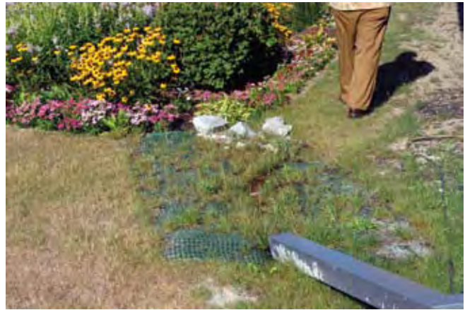
Erosion control matting and rock can be used at surface flow entrances
