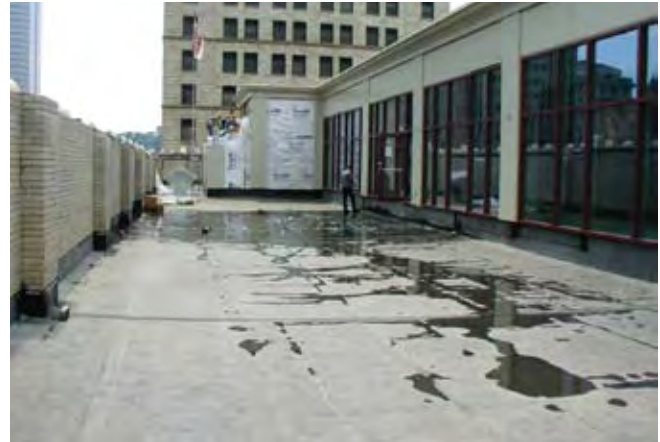
Conventional roof prior to retrofit
