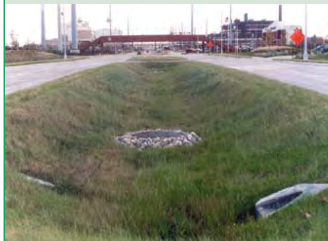
Swale along Miller Road in Dearborn, MI
