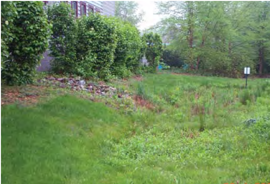
Roofleader directed toward bioretention
