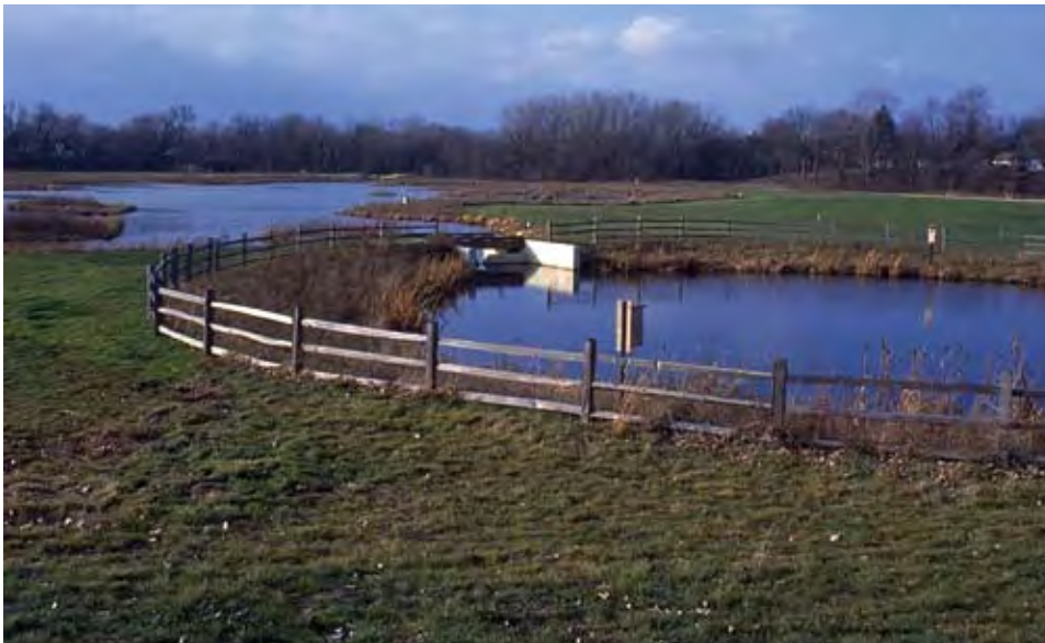
Inkster Valley constructed wetland
