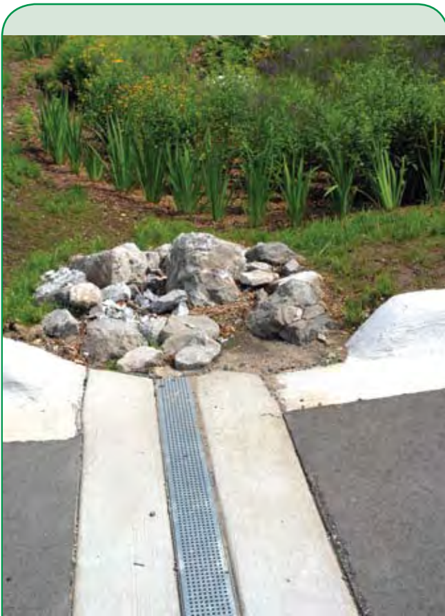
Horizontal grates can be added to a site as one way to separate stormwater from contaminated and non-contaminated areas. This was a measure employed at the Macomb County Public Administration Building to ensure that runoff from the site did not enter the storm drainage system in the older section of the parking lot, which directly drains to the Clinton River.
