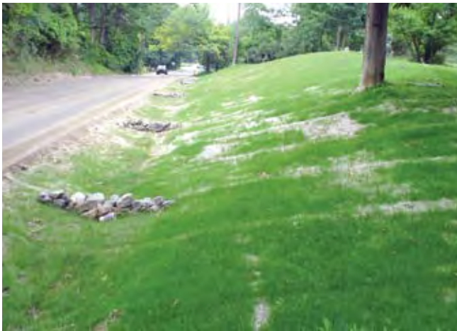
Stone check dams
