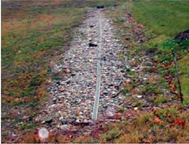
Washtenaw County West Service Center level spreader Source: Insite Design Studio, Inc.
