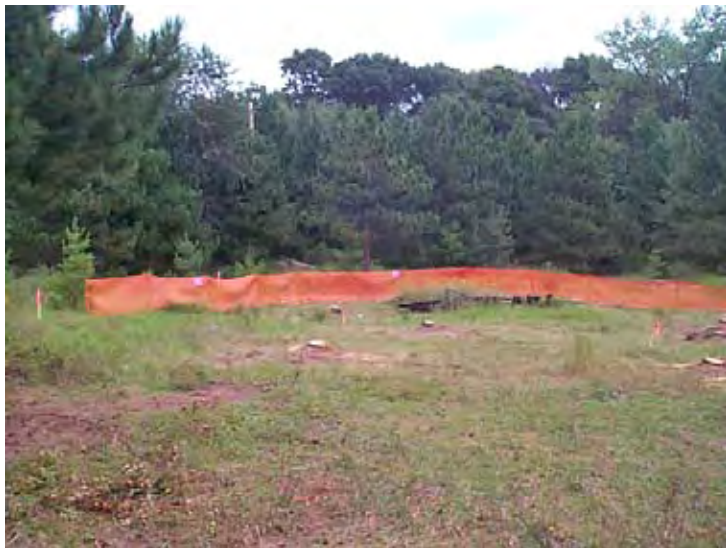
Minimizing disturbance of soil to protect wooded area
