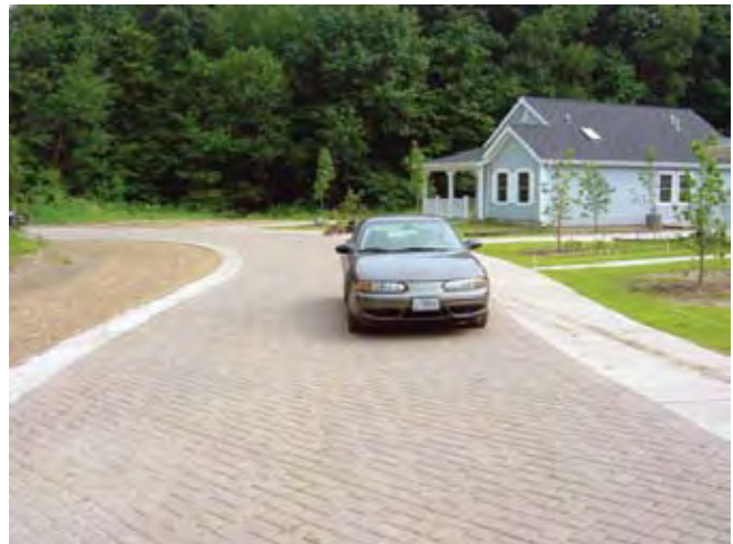
The Pokagonek Edawat Housing Development located in Dowagiac, MI includes the use of 25,000 square feet of interlocking pavers for the primary driving surface.
