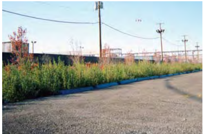
Porous asphalt lot with slow discharge to vegetated swale at Ford Motor Co., Dearborn, MI
