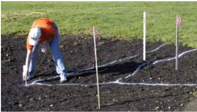
Marking planting area
