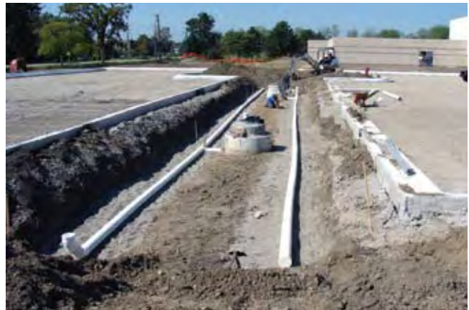
Underdrain in trench
