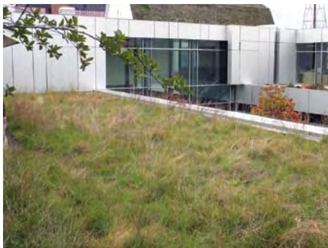
Vegetated roof with meadow grass Source: Conservation Design Forum, Inc.
