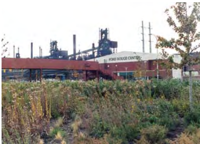
Native vegetation for stormwater infiltration at the Ford Rouge Center
