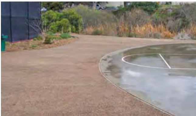
Colored pervious concrete
