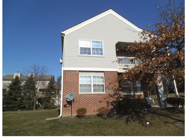
Photo 2: Exterior view of complex from parking lot
