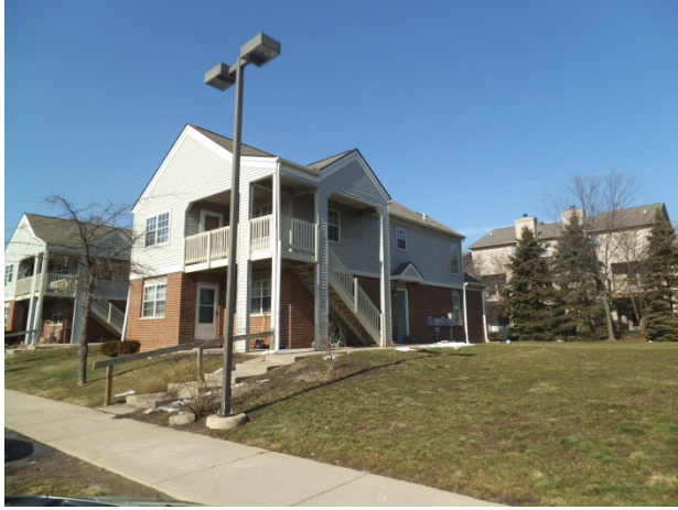
Photo 1: Front exterior of the complex
