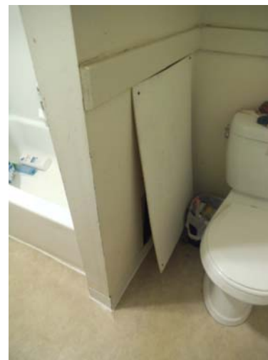
Effects of blower door test @ chase; pulling board off wall (unfastened)
