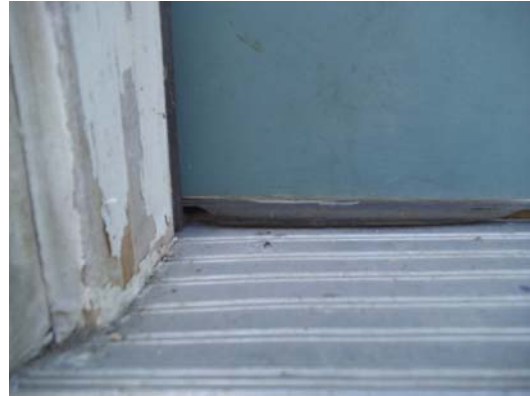
Weather-stripping and seals at threshold
