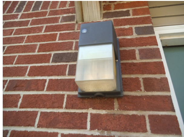
Photo 4: Typical wall-mounted exterior fixture
