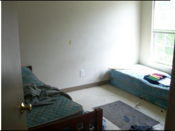
Photo #9: Bedroom 3, Unit 2676 Typical 3 bedroom
