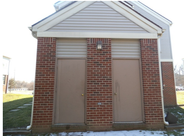
Photo 6: Storage areas behind each building
