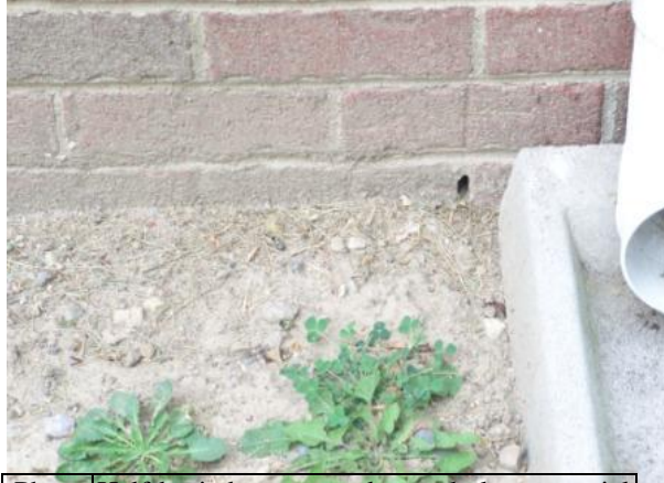
Photo #21: Half-buried unscreened weep holes, potential pest entry point and moisture issue
