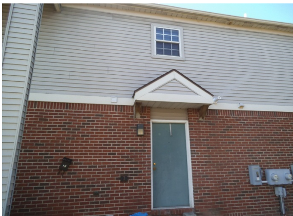
Photo 5: Side entrance on first floor
