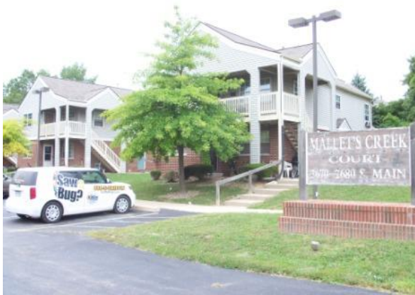
Photo #1: Street elevation
