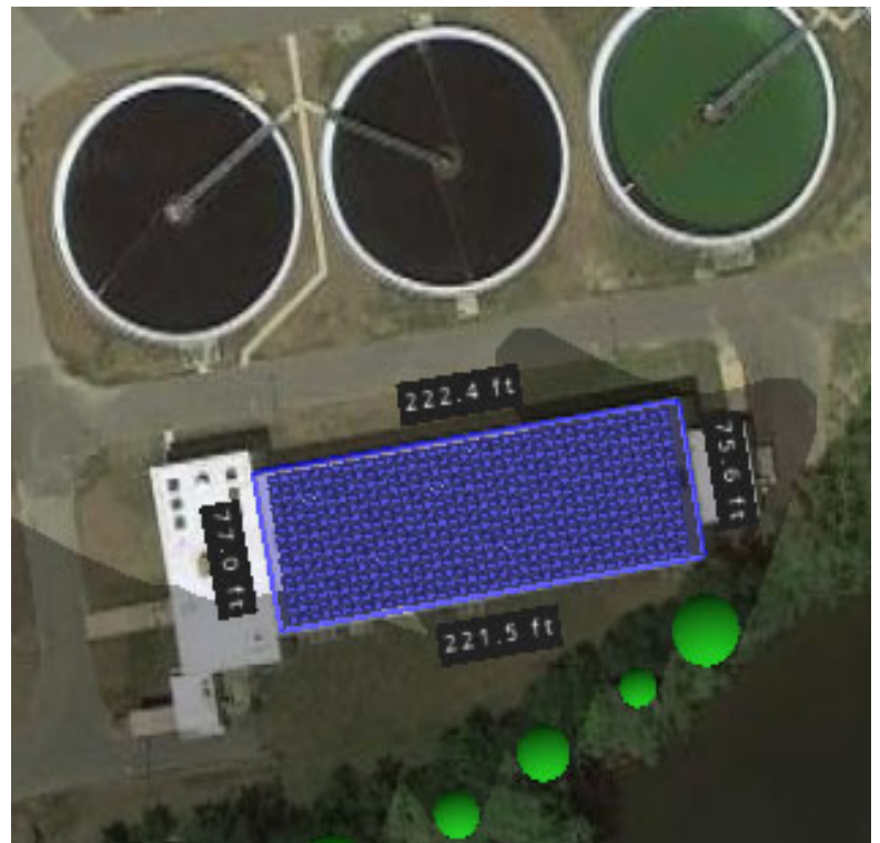
Site 13: Water Treatment Plant (160kw)
