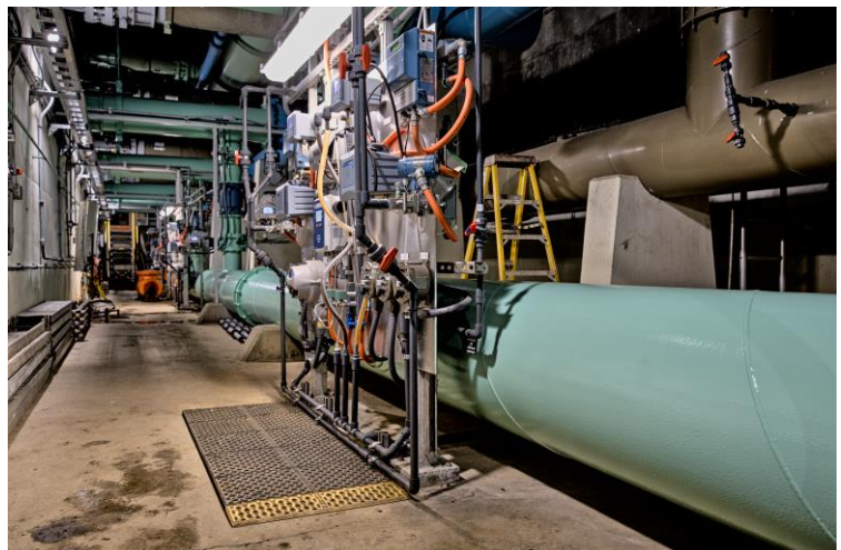
Water Treatment Plant Filter Gallery Rehabilitation Project
