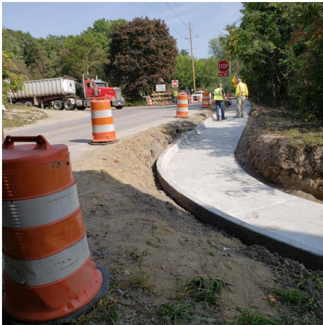
Barton at Boardwalk Sidewalk Installation
