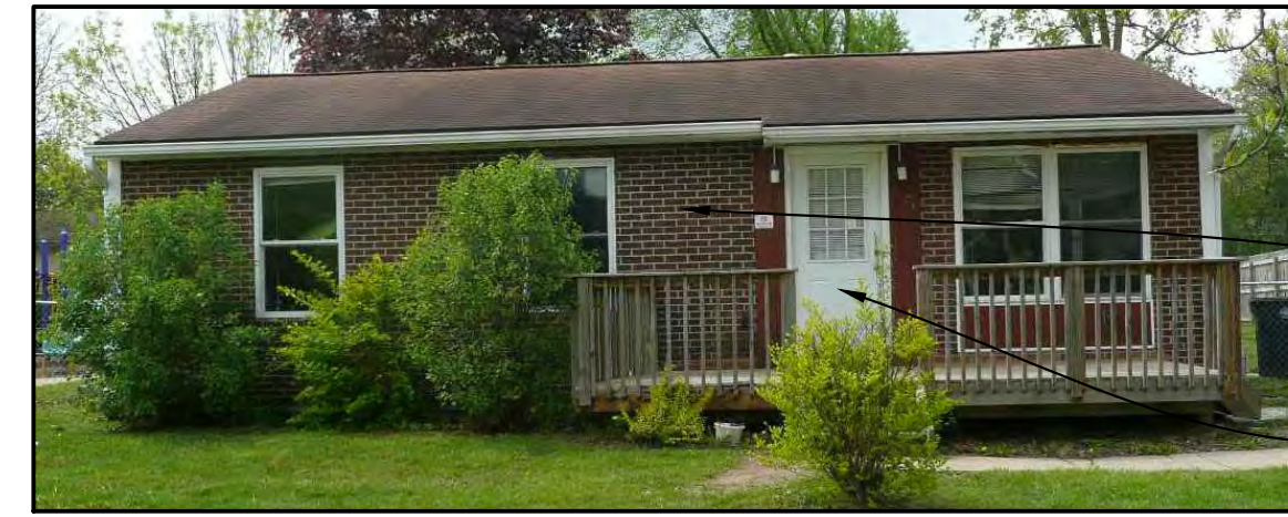
10 North Elevation - Photo A4.1 SCALE: No Scale Teen Center
