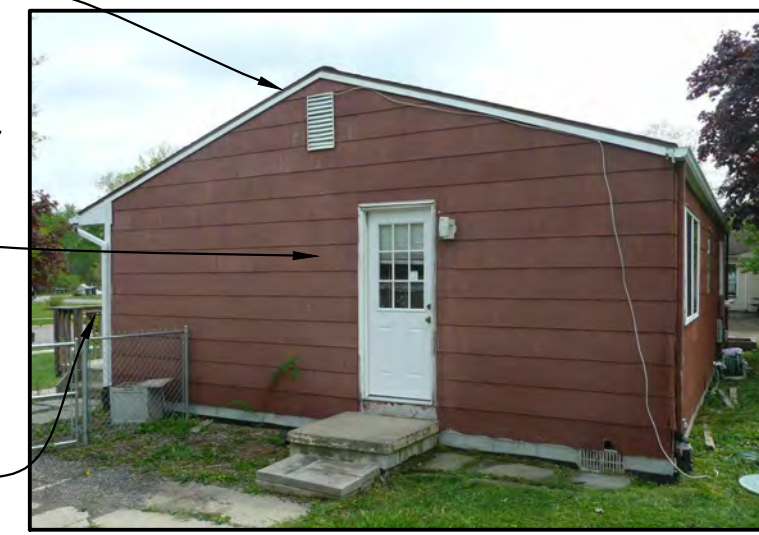
9 West Elevation - Photo A4.1 SCALE: No Scale Teen Center
