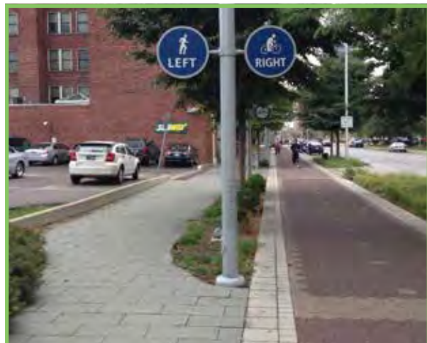
Figure 4-29. A cycle track (two-way protected bicycle lane) paired with a sidewalk along the Indianapolis Cultural Trail
