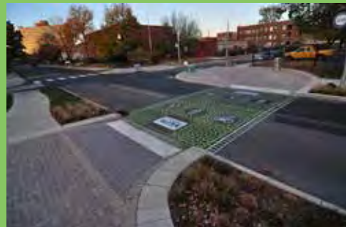
Figure 4-11. Enhanced stop sign intersection along Indianapolis Cultural Trail, featuring high-visibility crosswalks and corner bump-outs
