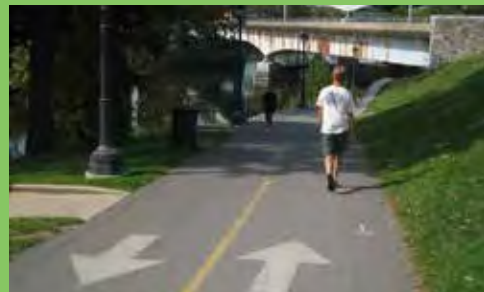
Figure 4-3. Two-lane path striping
