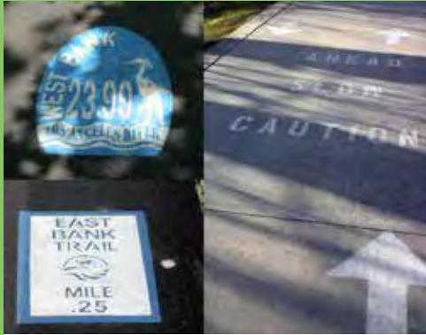
Figure 4-4. Safety, traffic, and mile markers on trail surfaces
