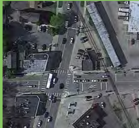
Figure 4-15. Main Street and Madison Street intersection
