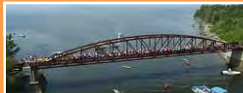
Figure 5-11. Winooski River Bridge
