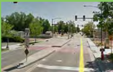
Figure 4-9. Crossing gates installed beyond sidewalk edge to block sidewalk and road, Ft. Collins, CO
