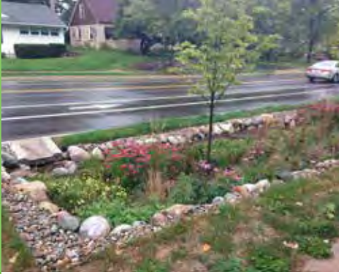
Figure 4-6. Small rain garden at Miller Avenue
