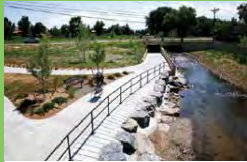
Figure 4-28. This bicycle path along the Left Hand Creek in Boulder, CO was credited with reducing flooding in the surrounding neighborhood
