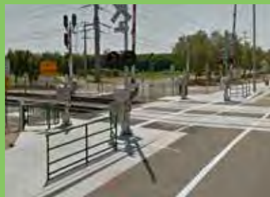
Figure 4-10. Fencing and crossing gates at rail/trail crossing, Irvine, CA
