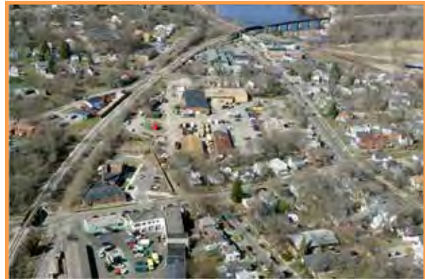
Figure 5-14. Overhead view of the City-owned 721 N. Main Street site; there are a number of potential options to connect this site to the Border-to-Border trail
