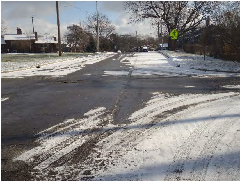
Looking east on Norwood from Fernwood
