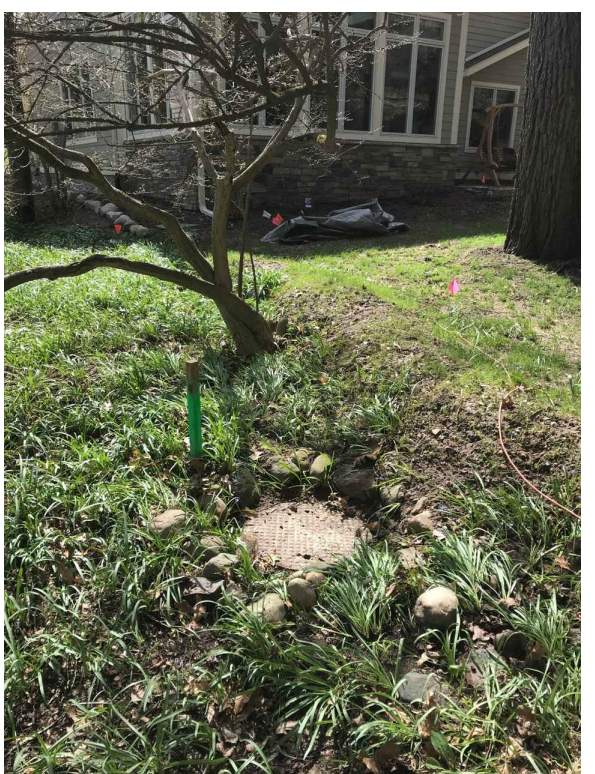
71-70042 • RIM: 829.58 • INVERT ELE: 821.58 • NOT ACCESSIBLE WITH A VEHICLE • PHOTO LOOKING SOUTHEAST
