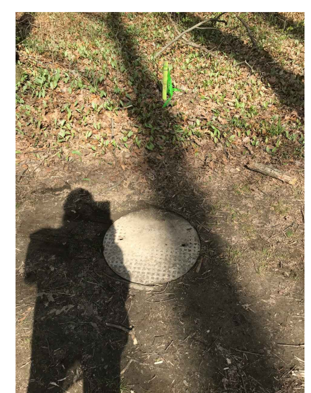
71-70044 RIM: 787.14 INVERT ELE: 781.14 PHOTO LOOKING SOUTHWEST
