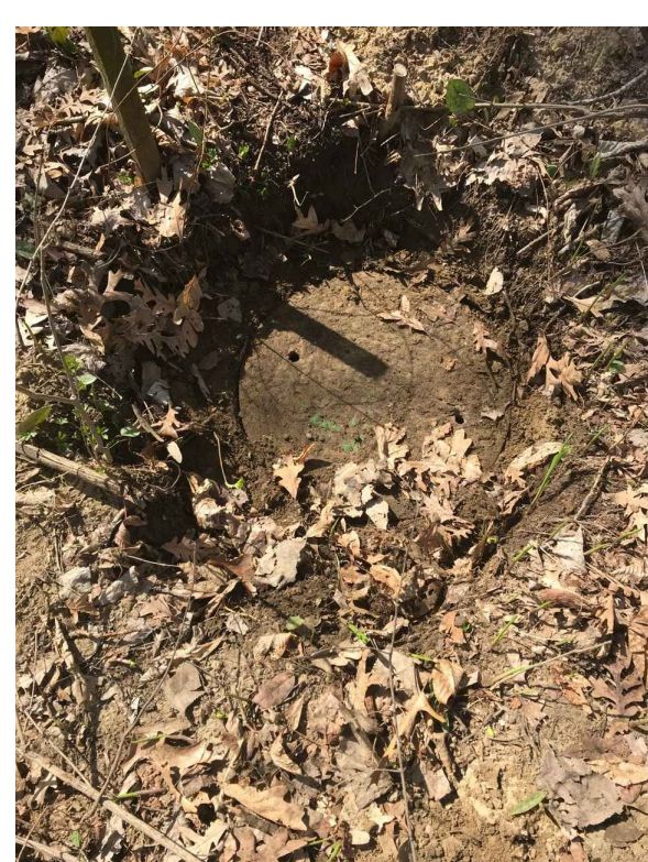
71-70045 MH ADJUST TO GRADE RIM: 789.84 INVERT ELE: 784.84 PHOTO LOOKING NORTHWEST
