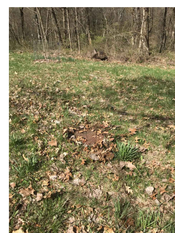
71-70046 RIM: 777.54 INVERT ELE: 772.60 PHOTO LOOKING NORTHWEST
