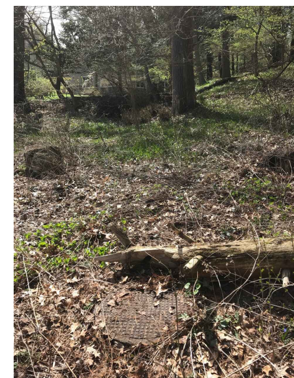
71-70039 • RIM: 823.20 • INVERT ELE: 818.20 • PHOTO LOOKING SOUTH
