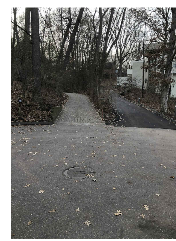
71-70075 • RIM: 775.42 • INVERT ELE: 765.70 • PHOTO LOOKING WEST
