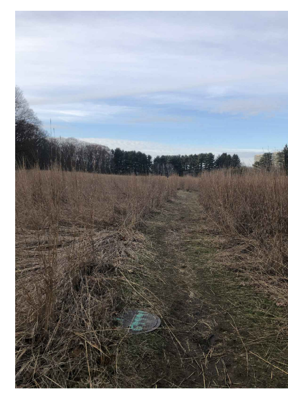
71-69941 • RIM: 771.86 • INVERT ELE: 766.50 • PHOTO LOOKING NORTHWEST
