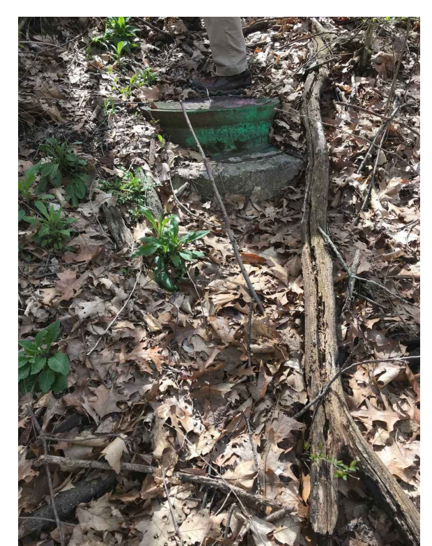
71-69894 RIM: 770.98 INVERT ELE: 775.98 NOT ACCESSIBLE WITH VEHICLE PHOTO LOOKING SOUTHEAST
