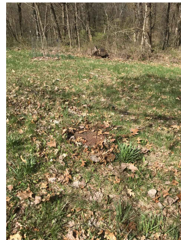
71-70046 • RIM: 777.54 • INVERT ELE: 772.60 • PHOTO LOOKING NORTHWEST
