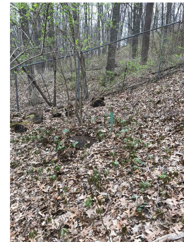
71-69942 • MH IN A FENCED BACK YARD. • REMOVE EX. FENCE & REPLACE WITH NEW SIMILAR FENCE • RIM: 816.34 • INVERT ELE: 807.34 • NOTE 1 • PHOTO LOOKING NORTH
