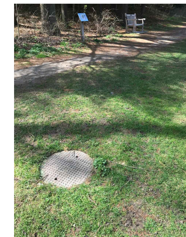
71-70032 • MH LITTLE OFFSET • RIM: 816.76 • INVERT ELE: 811.65 • PHOTO LOOKING WEST
