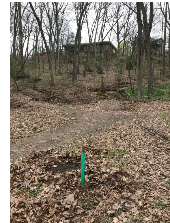
71-70015 • RIM: 807.21 • INVERT ELE: 802.21 • PHOTO LOOKING SOUTHEAST
