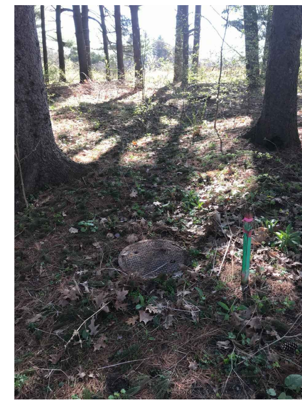
71-69896 • RIM: 775.11 • INVERT ELE: 767.41 • SEE NOTE 1 • PHOTO LOOKING SOUTH
