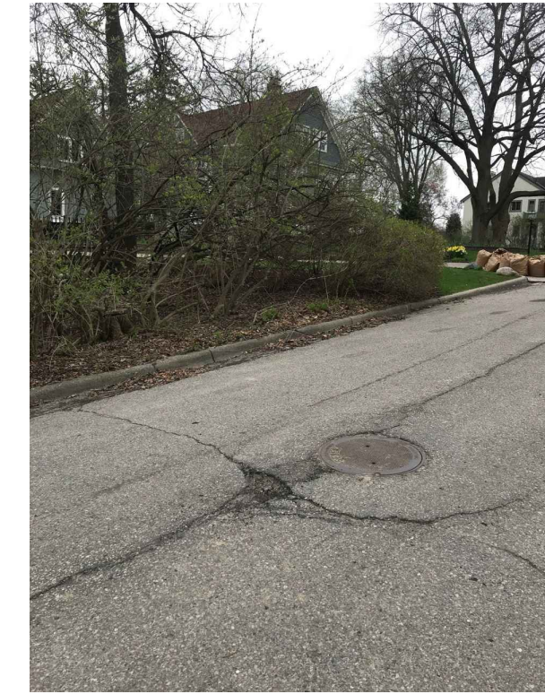
71-69198 • RIM: 921.38 • INVERT ELE: 913.26 • PHOTO LOOKING SOUTH
