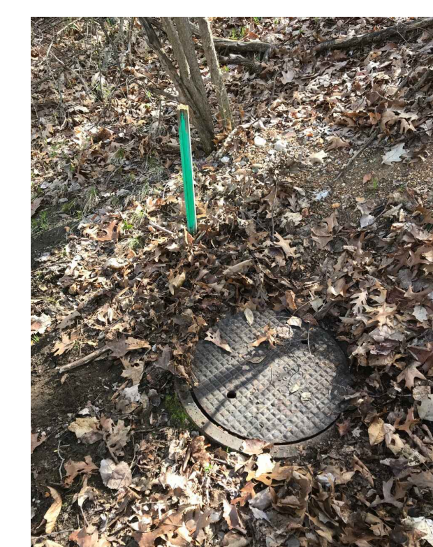
71-69899 RIM: 771.77 INVERT ELE: 778.77 SEE NOTE 1 PHOTO LOOKING SOUTHEAST
