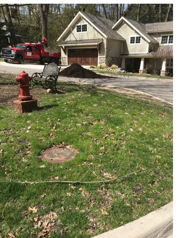
71-70027 • MH BETWEEN HOUSE NO. 28 & 26. • DROP PIPE • RIM: 838.00 • INVERT ELE: 825.97 • PHOTO LOOKING WEST
