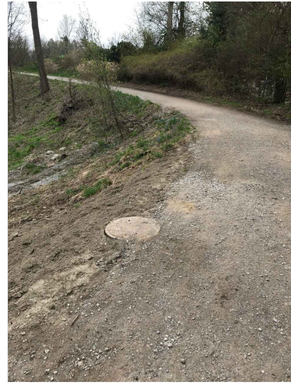
71-70035 • MH AT AN EDGE OF A HILL AND NICHOLAS DR. • RIM: 883.65 • INVERT ELE: 879.65 • PHOTO LOOKING SOUTH
