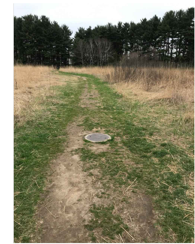
71-69891 • RIM: 772.52 • INVERT ELE: 767.37 • PHOTO LOOKING WEST
