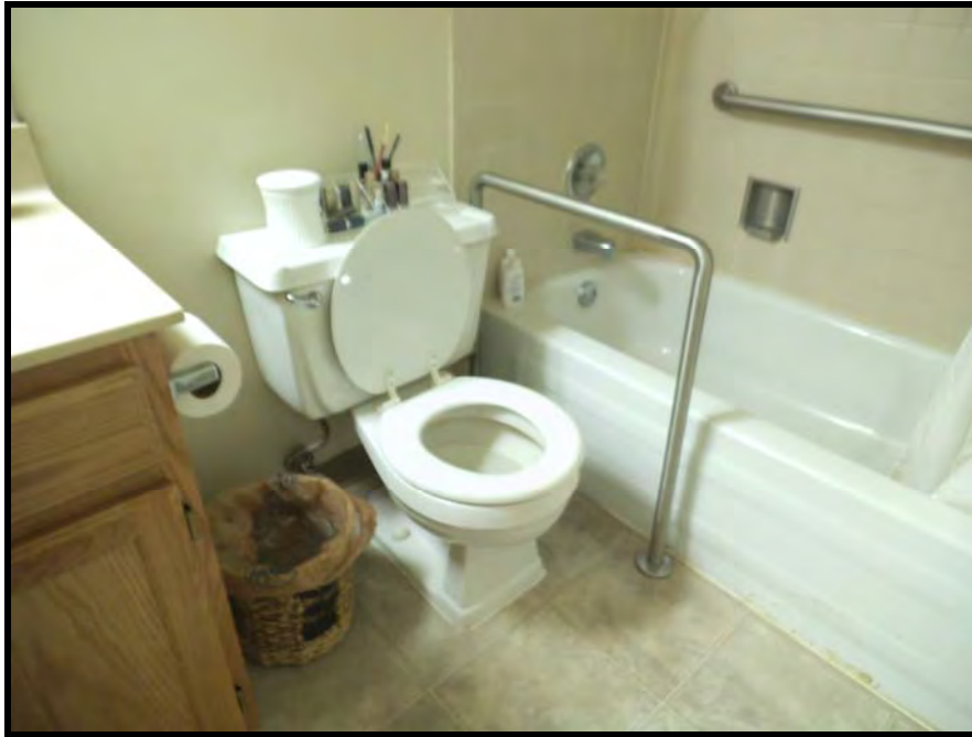
PHOTOGRAPH NO. 15: SUBJECT BUILDING: TYPICAL VIEW OF TENANT UNIT BATHROOM
