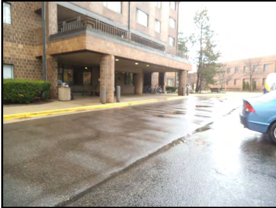
PHOTOGRAPH NO. 1: SUBJECT BUILDING AS VIEWED FACING NORTHWEST
