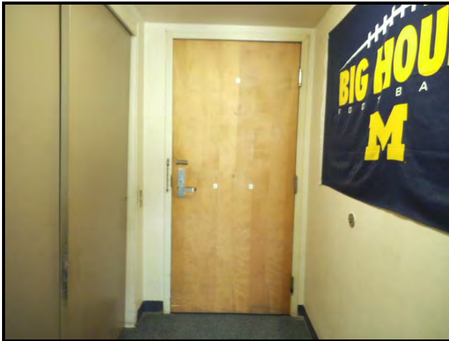
PHOTOGRAPH NO. 12: SUBJECT BUILDING: TYPICAL VIEW OF TENANT UNIT ENTRANCE DOOR
