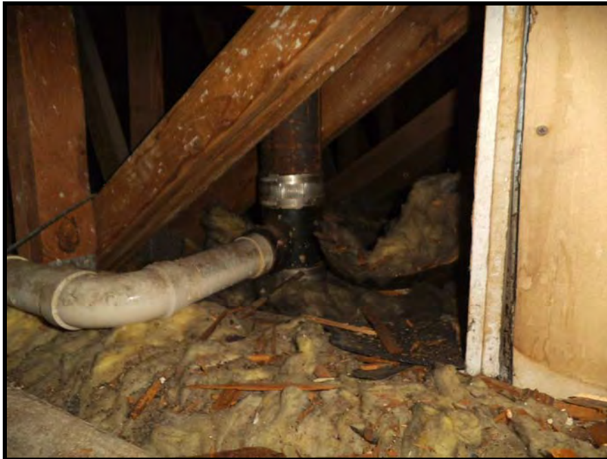
PHOTOGRAPH NO. 22: SUBJECT BUILDING: VIEW OF INSULATION IN ATTIC SPACE
