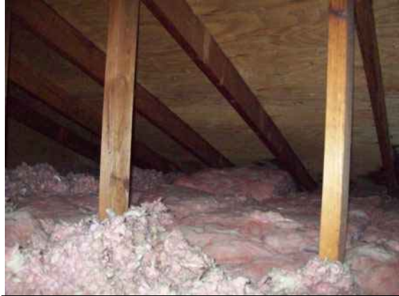
Photo #8: Attic insulation
