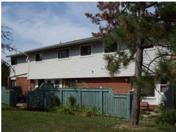
Photo #5: Rear elevation of typical building
