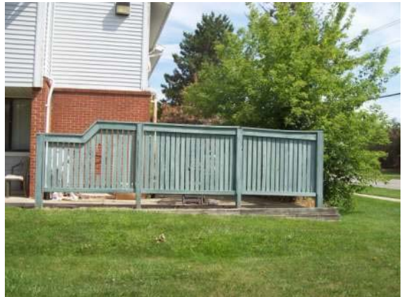
Photo #46: Patio fencing
