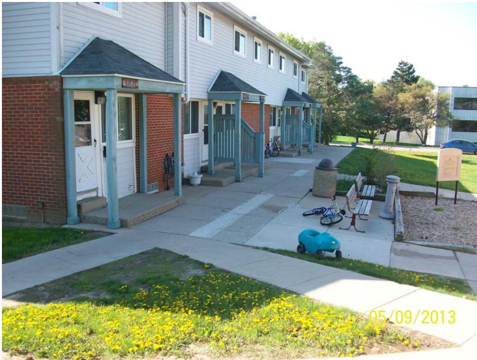
Photograph 5: Typical building front and front doors to the apartment units.
