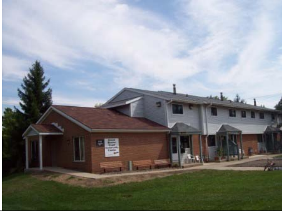
Photo #37: Community Center
