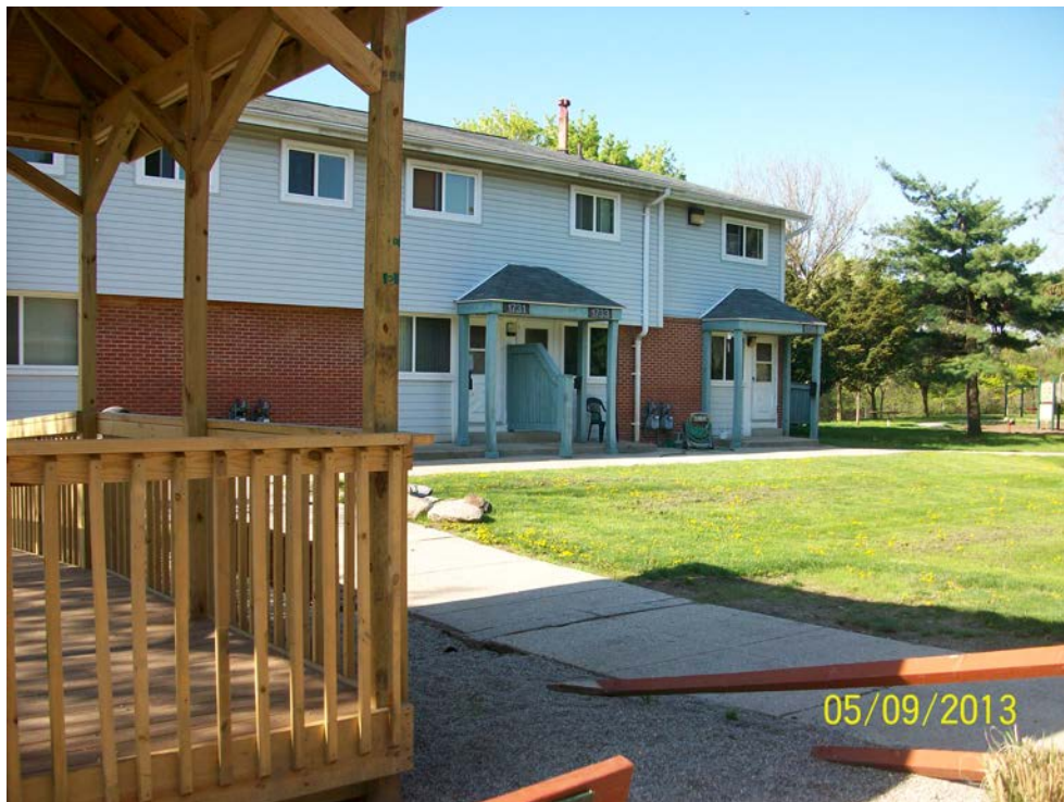
Photograph 4: Typical building front and front doors to the apartment units.
