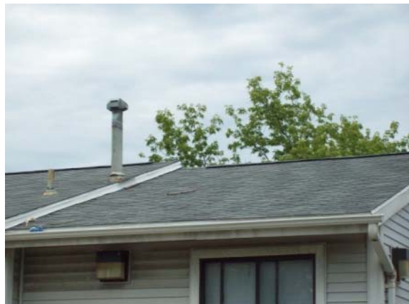
Photo #6: Roof overview
