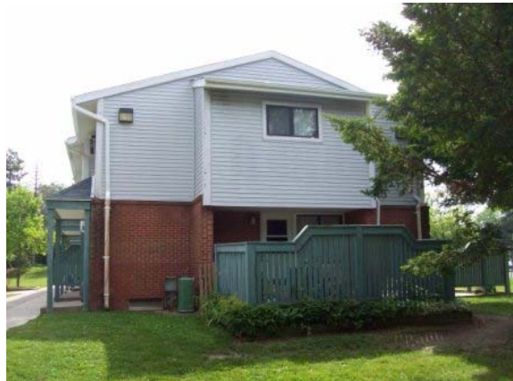
Photo #4: Right side elevation of typical building
