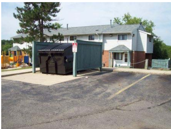
Photo #47: Dumpster pad and enclosure
