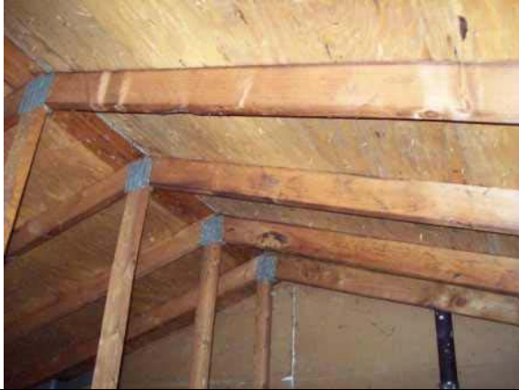
Photo #7: Attic construction
