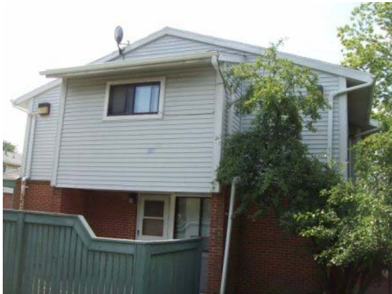
Photo #3: Left side elevation of typical building
