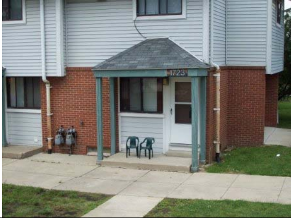
Photo #13: Apartment entry structure
