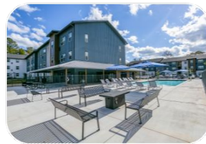
The Annex of Ruston Ruston, LA Student Housing 118 units/324 beds
