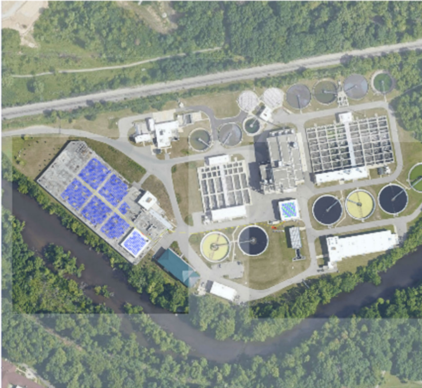
WATER RECOVERY CENTER CITY OF ANN ARBOR, MI PRELIMINARY SOLAR AND STORAGE ARRAY
