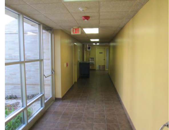
Photo 6: Exit Sign/Fire Alarm/CO Detector
