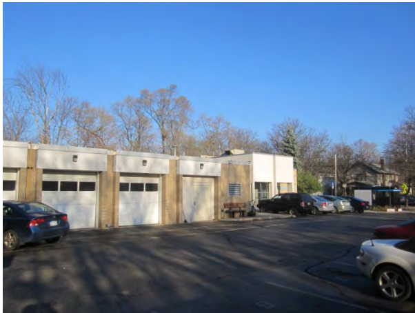
Photo 3: Office Area and Service Door
