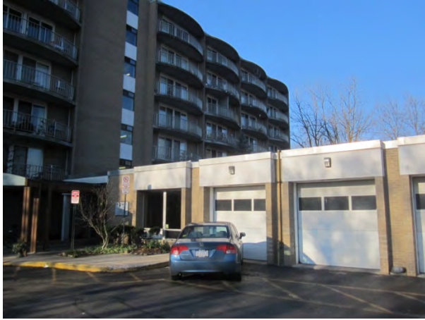
Photo 1: Visitor Entrance and Service Doors
