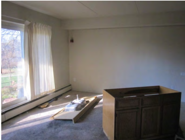
Photo 9: Baseboard finned-tube heating units
