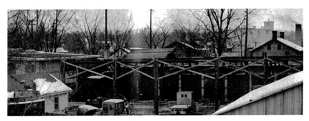
After the high bay framing was in place, major portions of the old concrete garage and concrete machine shop and all remaining structures except for a couple of wood framed buildings were demolished. A new two-story concrete frame "L" shaped building (colored green) with offices on the top floor was constructed along the north and west sides of the high bay space as it was being finished.
