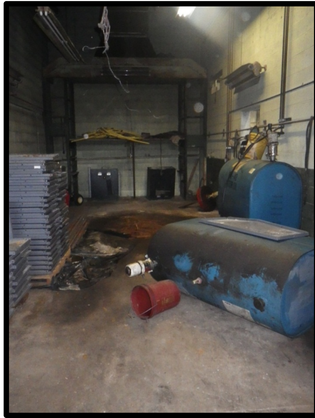
Motor oil tanks in paint booth of maintenance garage
