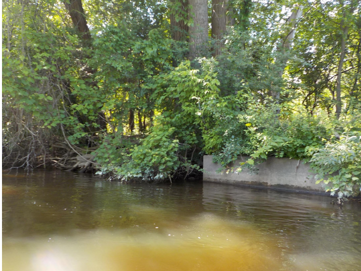
Document Name: DSCN3011.JPG Category: Channel Span Number: Comments: SW quadrant
