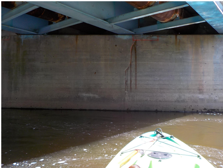
Document Name: DSCN3005.JPG Category: Substructure Span Number: Comments: East abutment
