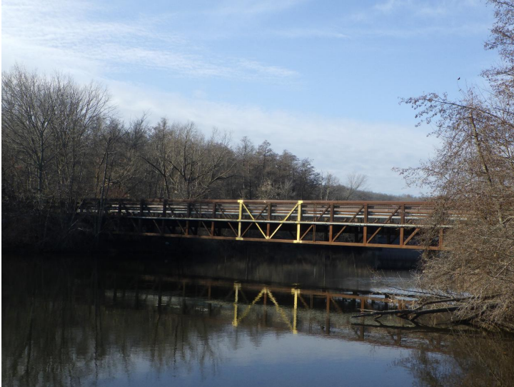
Document Name: R0012530.JPG Category: Elevation Span Number: 1 Comments: East elevation of bridge
