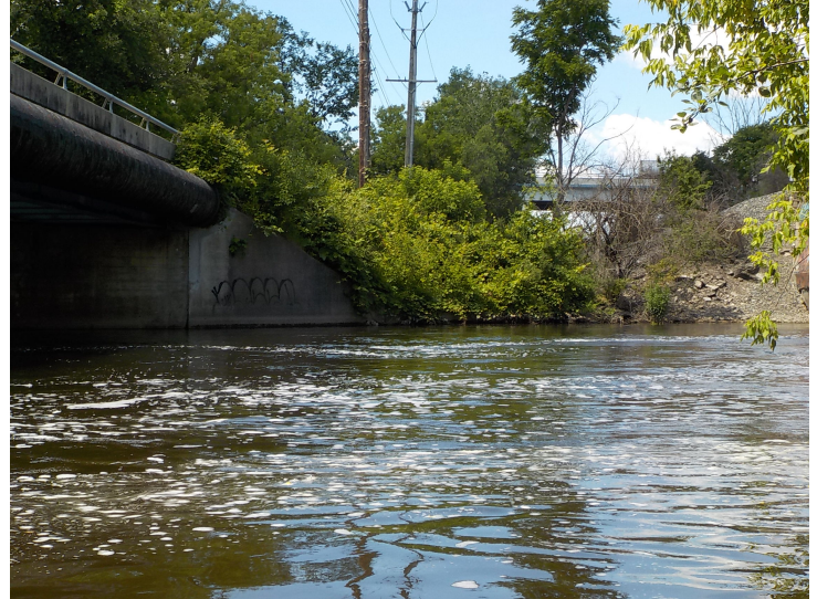
Document Name: DSCN3012.JPG Category: Channel Span Number: Comments: NW quadrant
