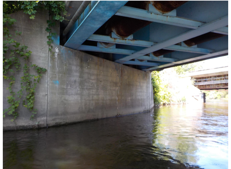
Document Name: DSCN3010.JPG Category: Substructure Span Number: Comments: West abutment
