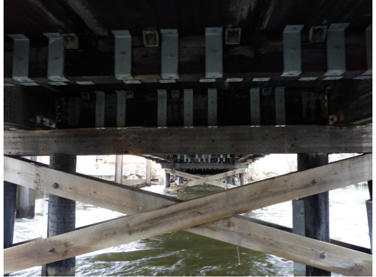
Document Name: R0011809.JPG Category: Substructure Span Number: Comments: Typical pier
