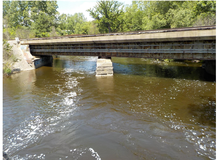
Document Name: DSCN3015.JPG Category: Channel Span Number: Comments: Looking upstream/north
