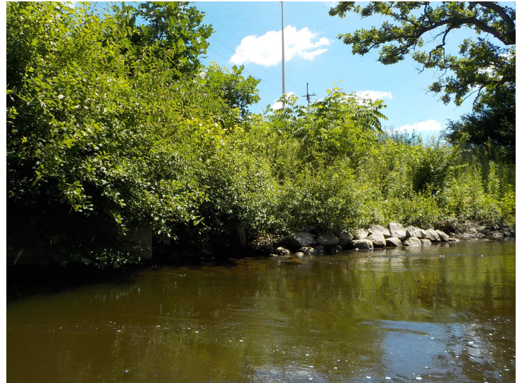
Document Name: DSCN3007.JPG Category: Channel Span Number: Comments: SE quadrant
