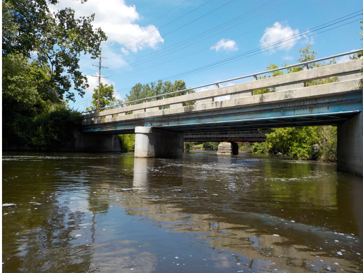
Document Name: DSCN3008.JPG Category: Elevation Span Number: Comments: South elevation
