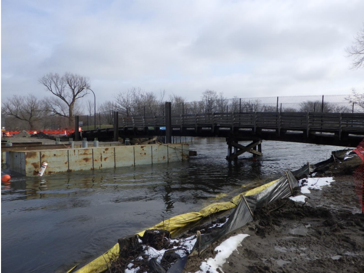
Document Name: R0011785.JPG Category: Elevation Span Number: Comments: West elevation of bridge
