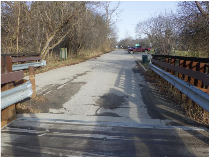
Document Name: R0012527.JPG Category: Approach Span Number: Comments: North approach
