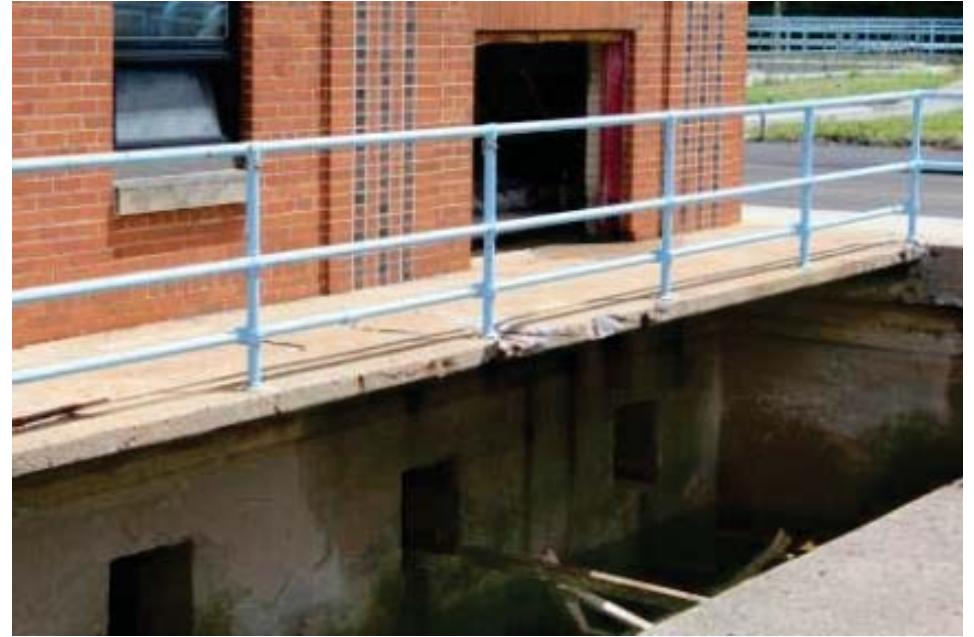
Flocculation Basin No. 3 Stage 1 and Cantilevered Concrete Slab
