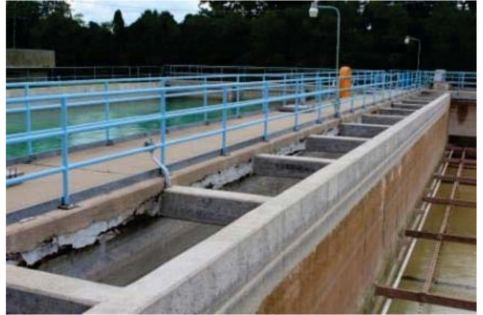
Basin Nos. 1 & 2 Settled Water Effluent Channel and Center Walkway
