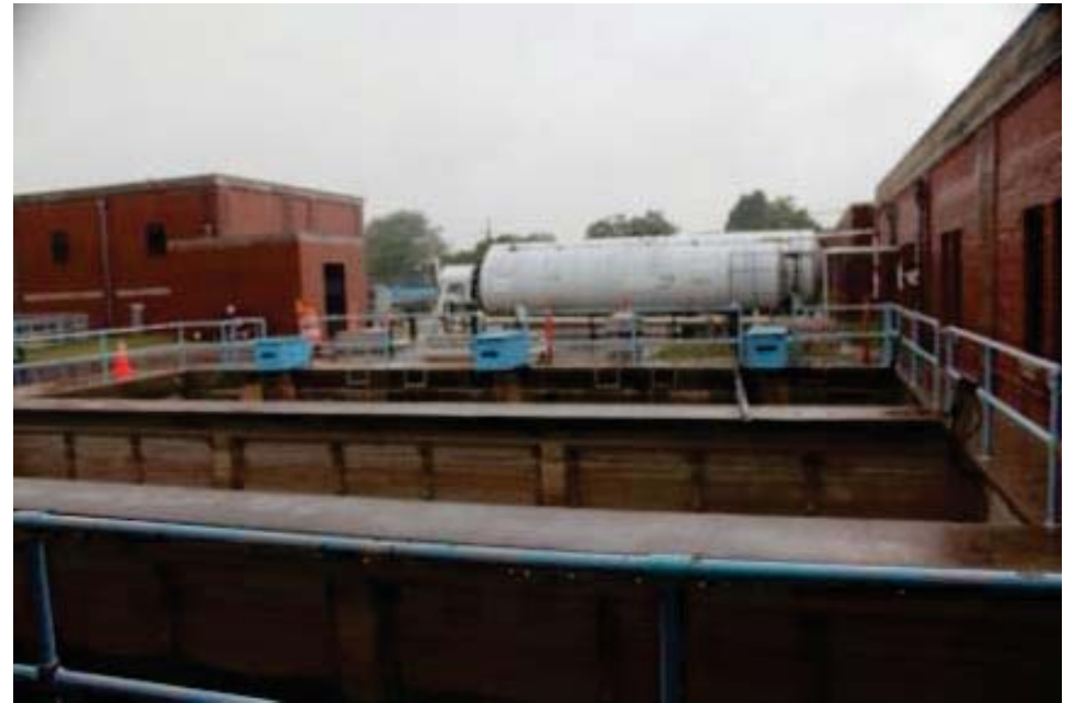
Flocculation Basin No. 3
