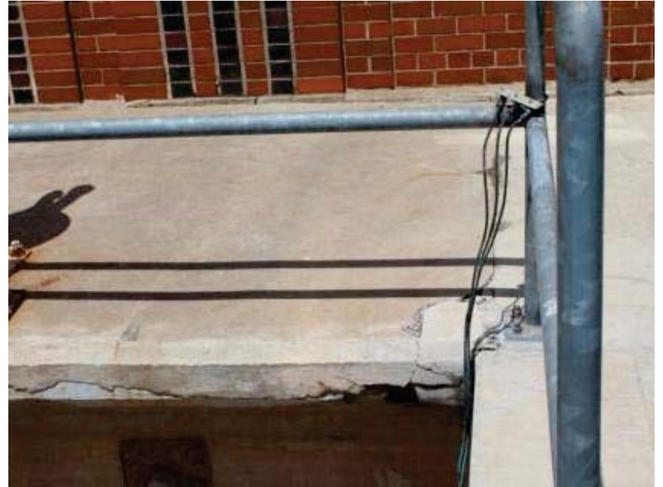
Basin No. 2 Cantilevered Concrete Walkway, Northeast Corner
