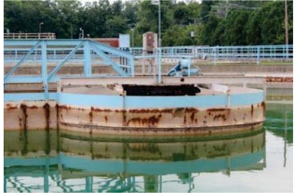
Settling Basin No. 3 Center Column
