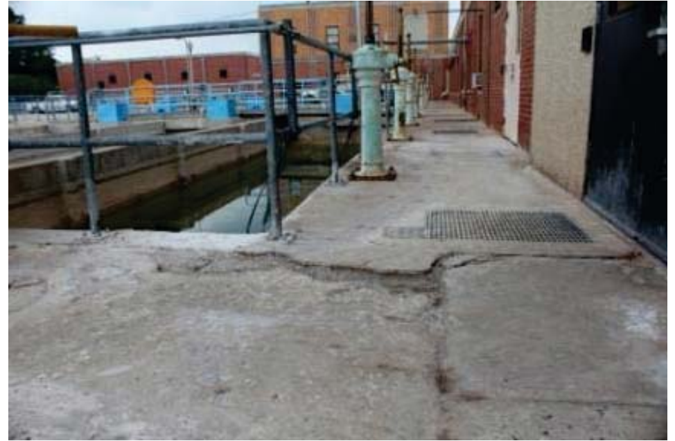
Basin No. 1 perimeter walkway at northeast corner
