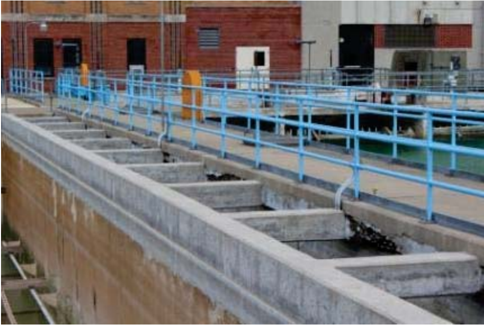
Basin Nos. 1 & 2 Settled Water Effluent Channel and Center Walkway
