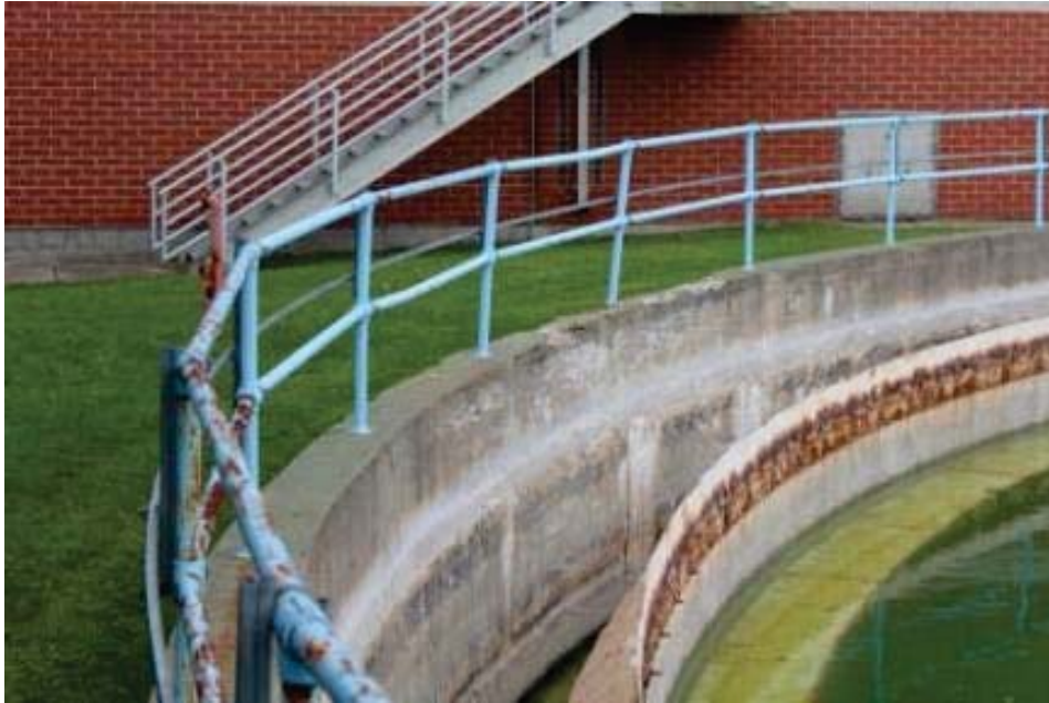
Basin No. 3 Effluent Weir and Effluent Channel
