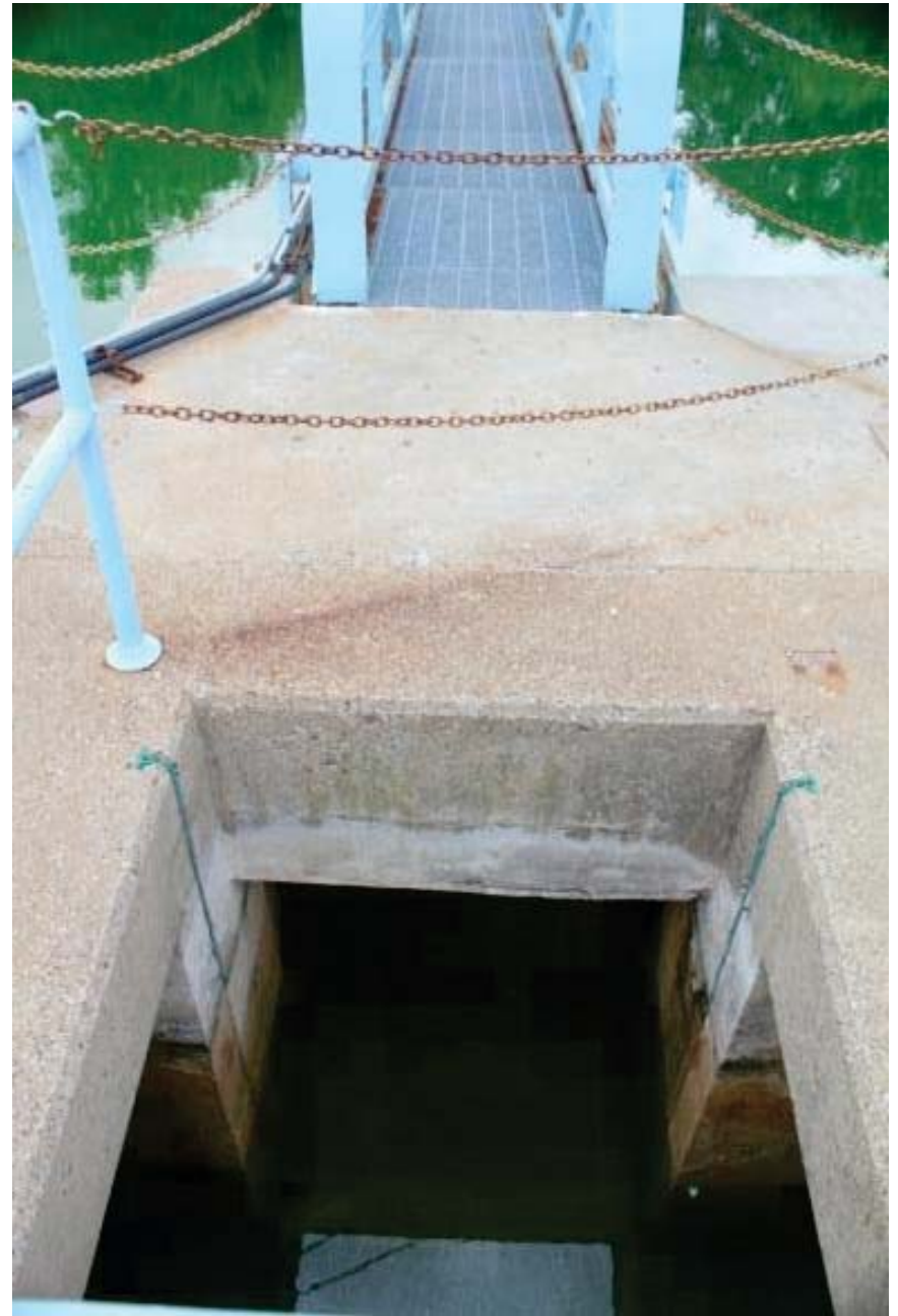
Basin No. 3 North Effluent Structure and Slide Plate Frame
