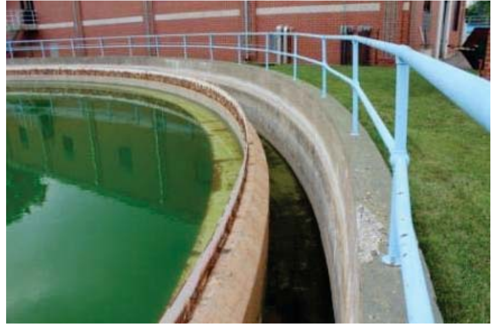
Settling Basin No. 3 Effluent Weir and Effluent Channel
