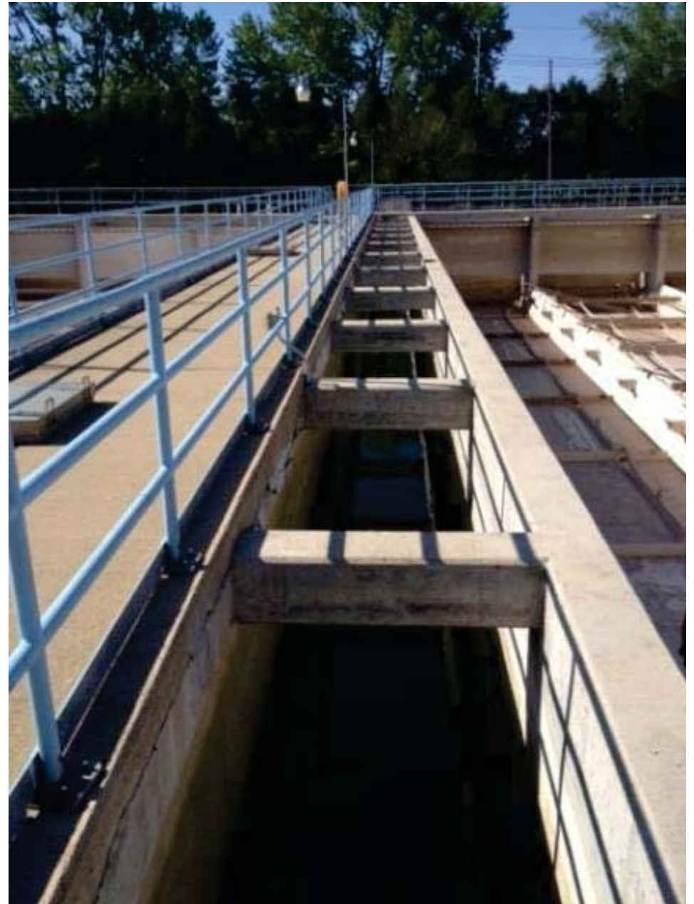
Basin Nos. 1 & 2 Settled Water Effluent Channel
