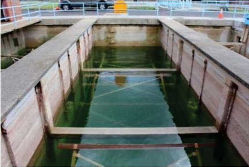
Flocculation Basin No. 3 Stage 2 and Baffle Walls
