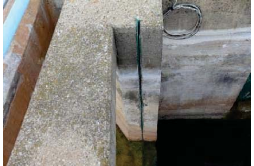
Basin No. 3 North Effluent Structure and Slide Plate Frame
