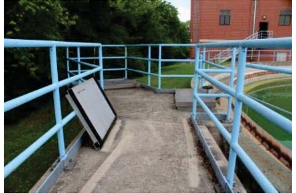
Basin No. 3 Effluent Channel and Stop Logs
