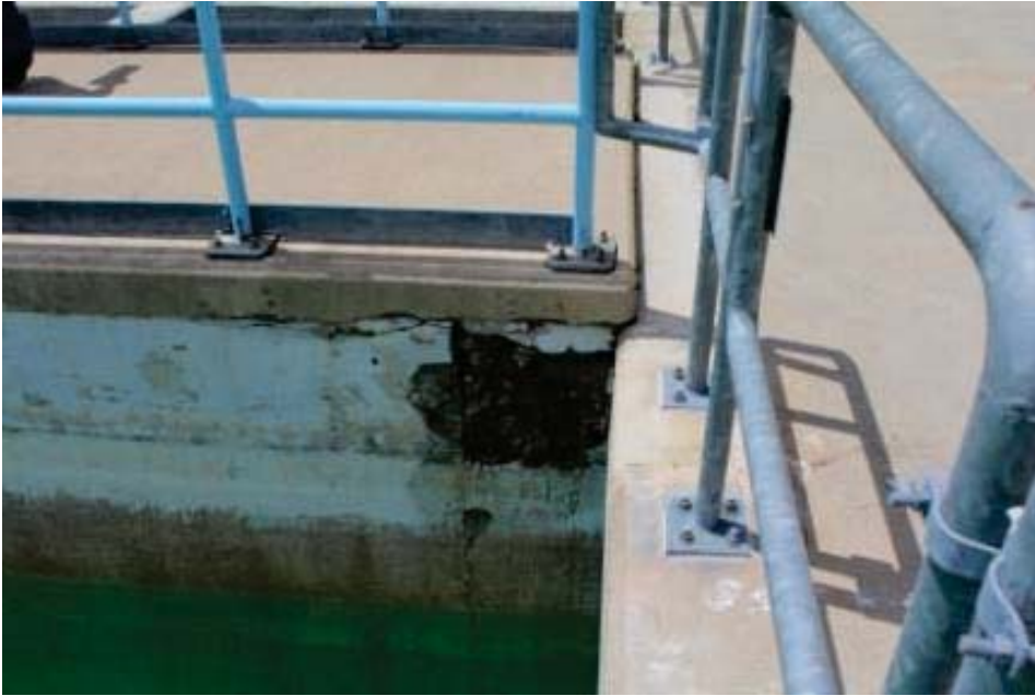
Basin Nos. 1 & 2 Walkway Concrete
