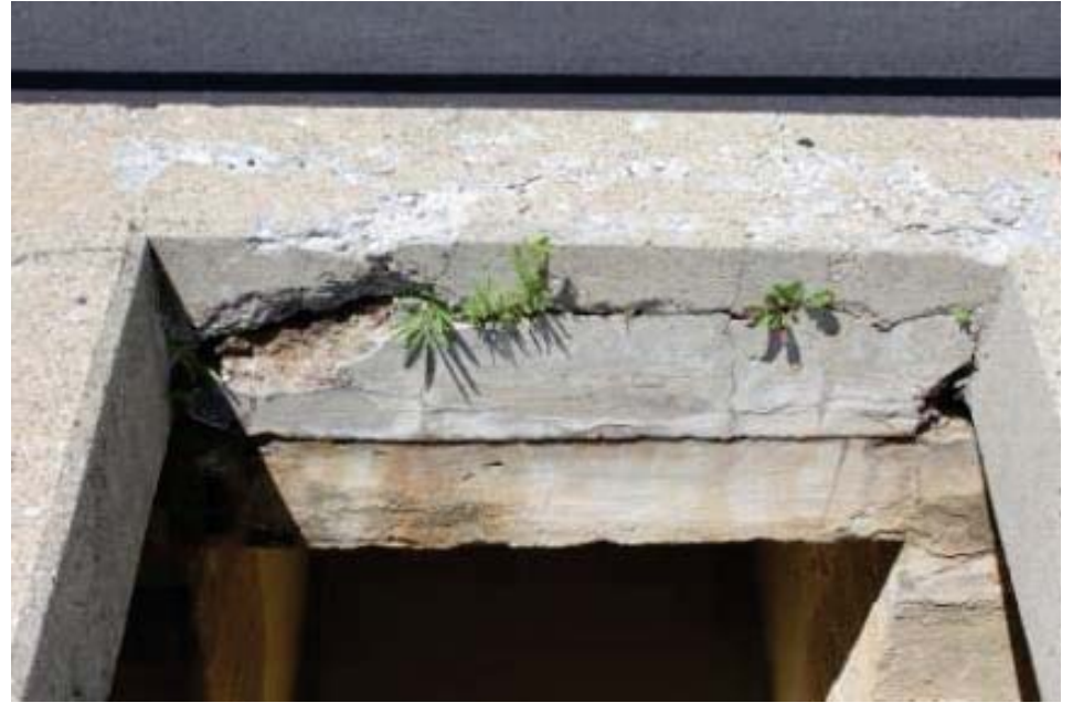
Basin No. 3 North Effluent Structure
