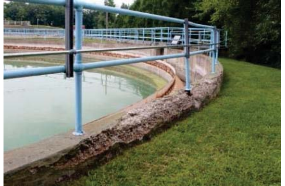
Settling Basin No. 3 Effluent Channel
