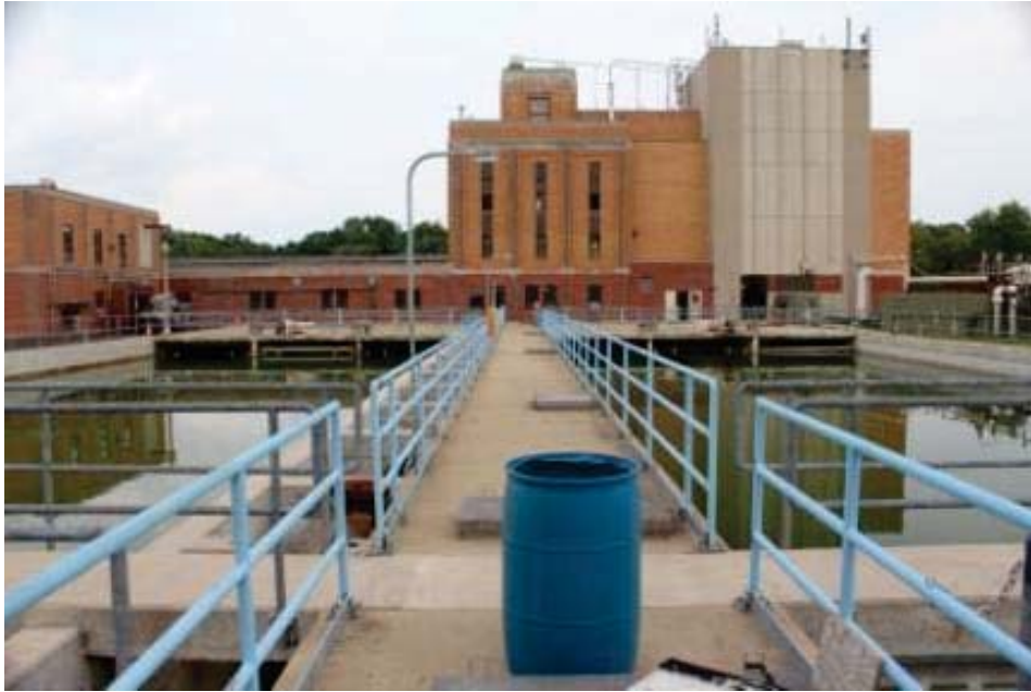
Basin Nos. 1 & 2 Center Walkway
