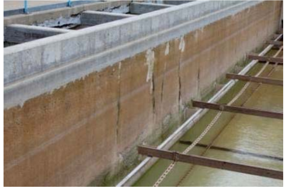
Basin No. 2 Settling Basin Concrete Wall and Center Walkway
