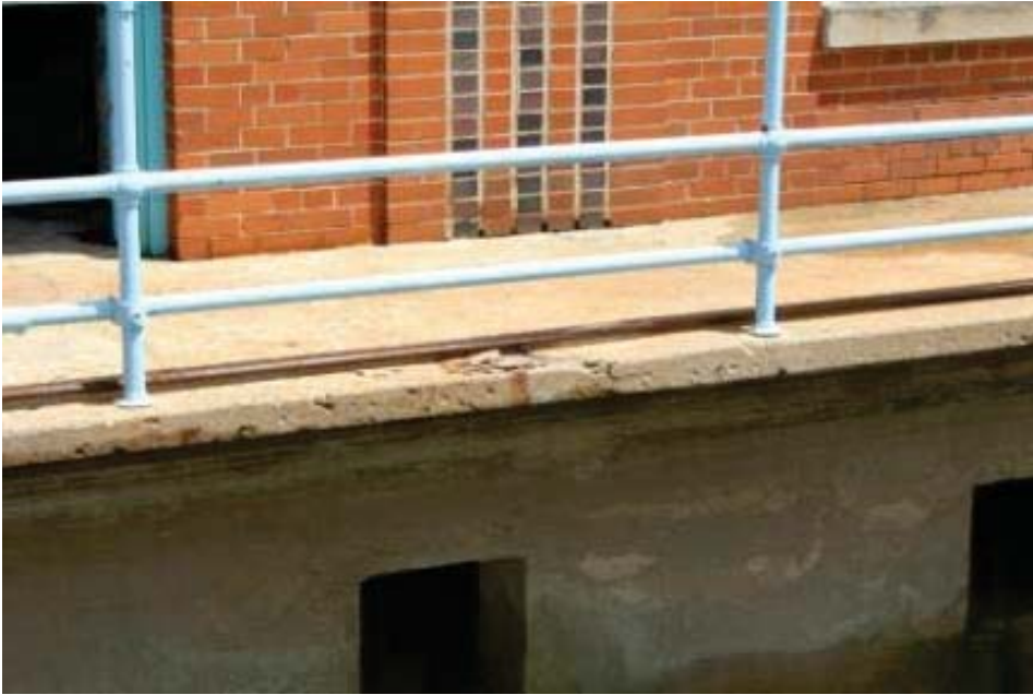
Flocculation Basin No. 3 Stage 1 Cantilevered Concrete Slab
