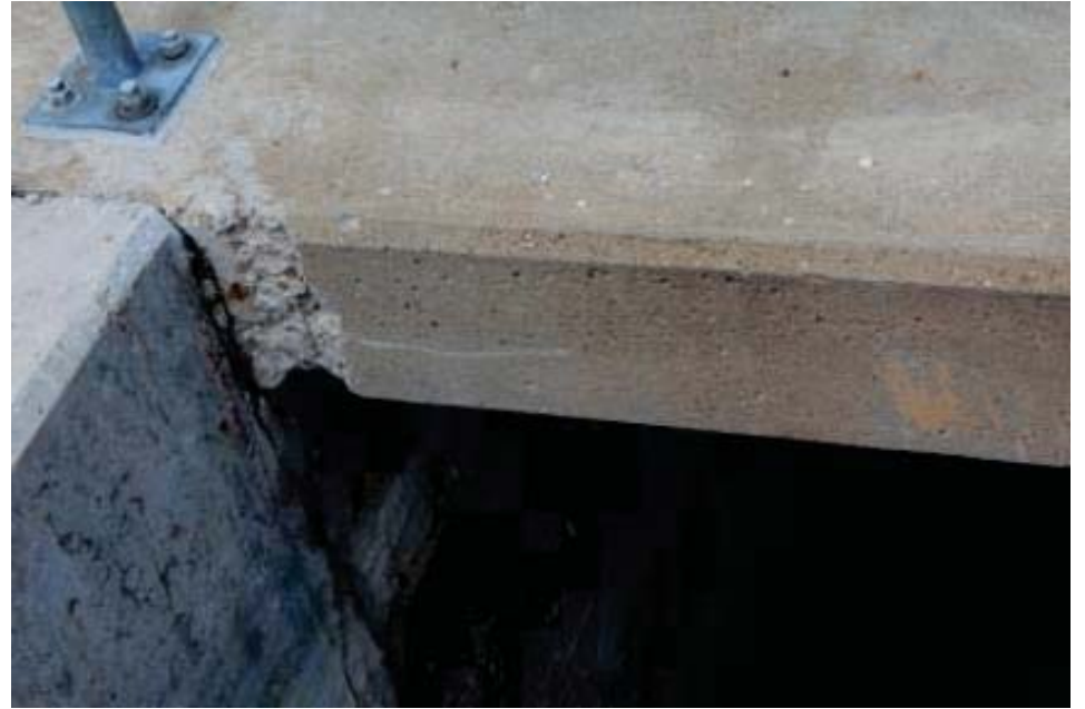
Basin Nos. 1 & 2 Walkway Concrete
