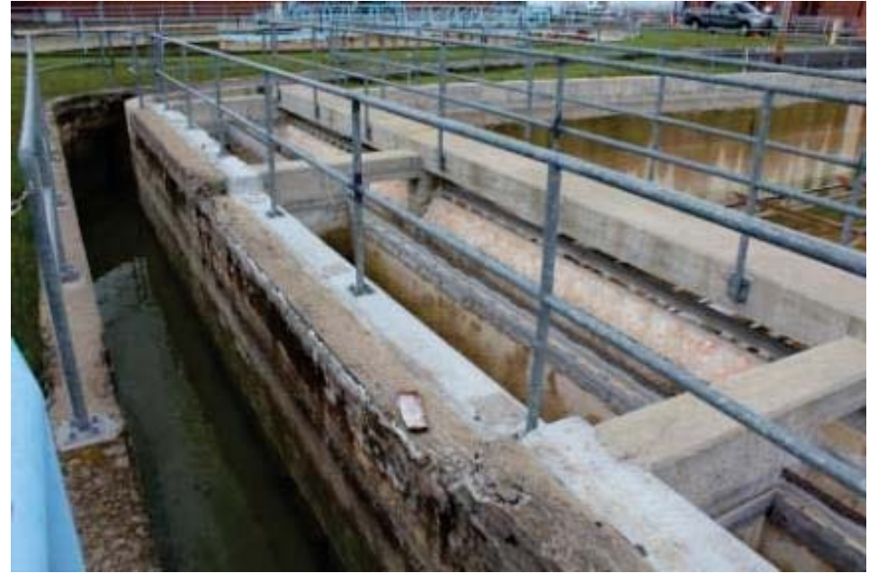
Basin No. 2 Effluent Weirs and Revised Effluent Channel
