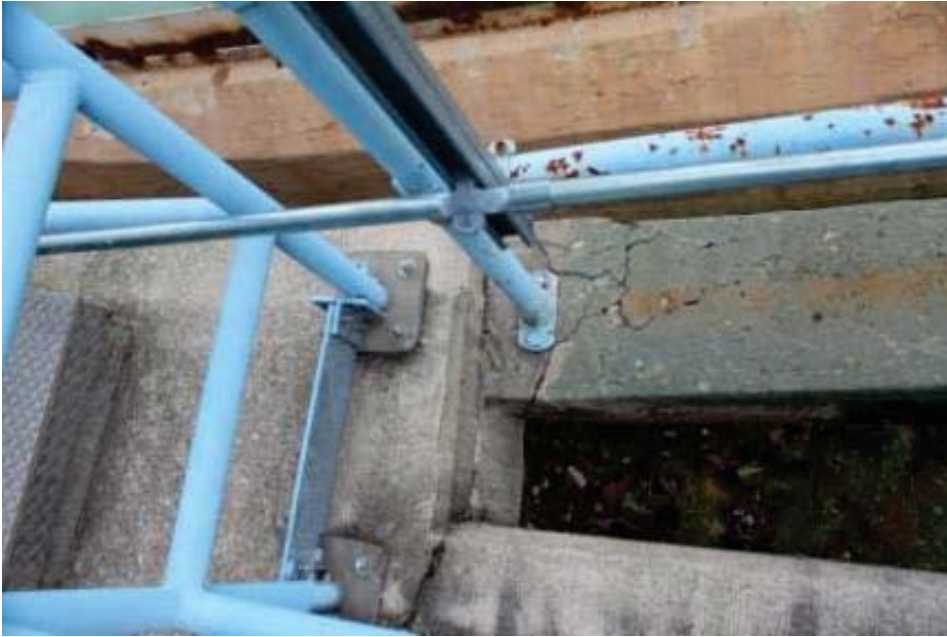
Basin No. 3 South Effluent Structure
