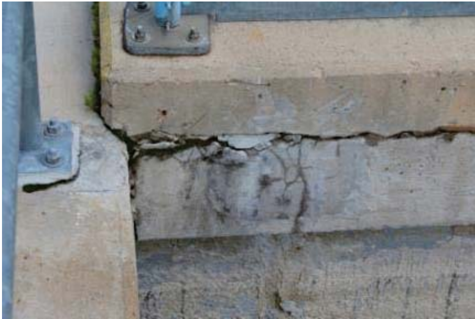
Basin Nos. 1 & 2 Walkway Concrete
