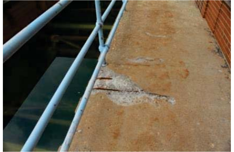
Flocculation Basin No. 3 Stage 1 Cantilevered Concrete Slab
