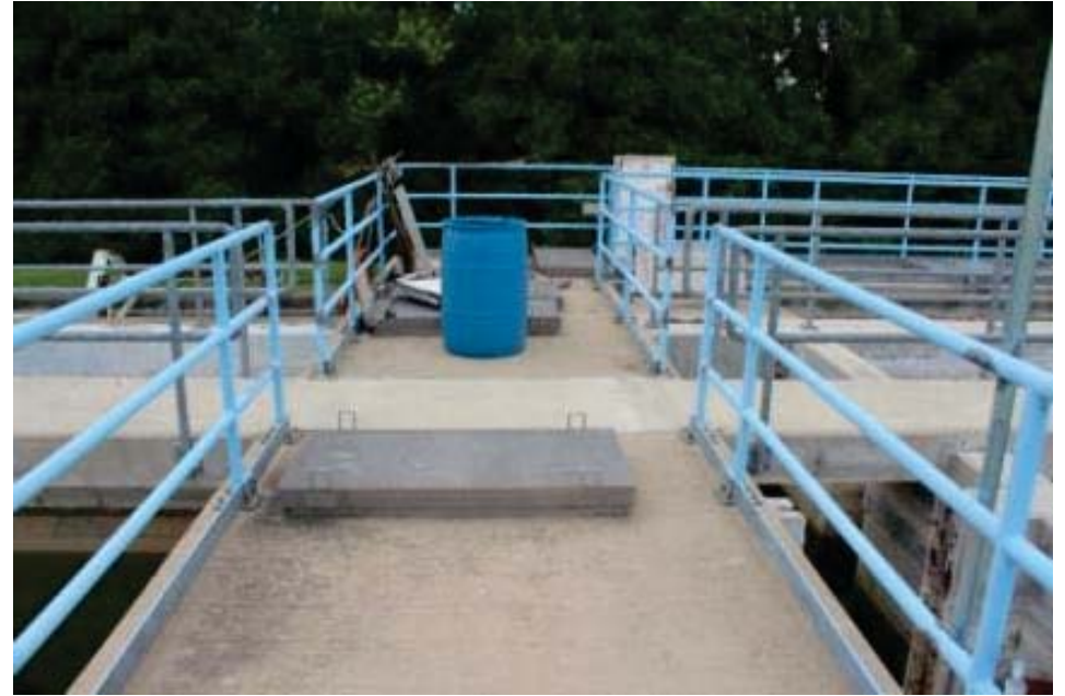
Basin Nos. 1 & 2 Effluent Stop Log Structures
