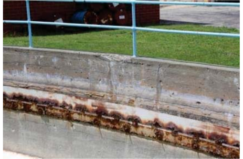
Basin No. 3 Effluent Weir and Effluent Channel
