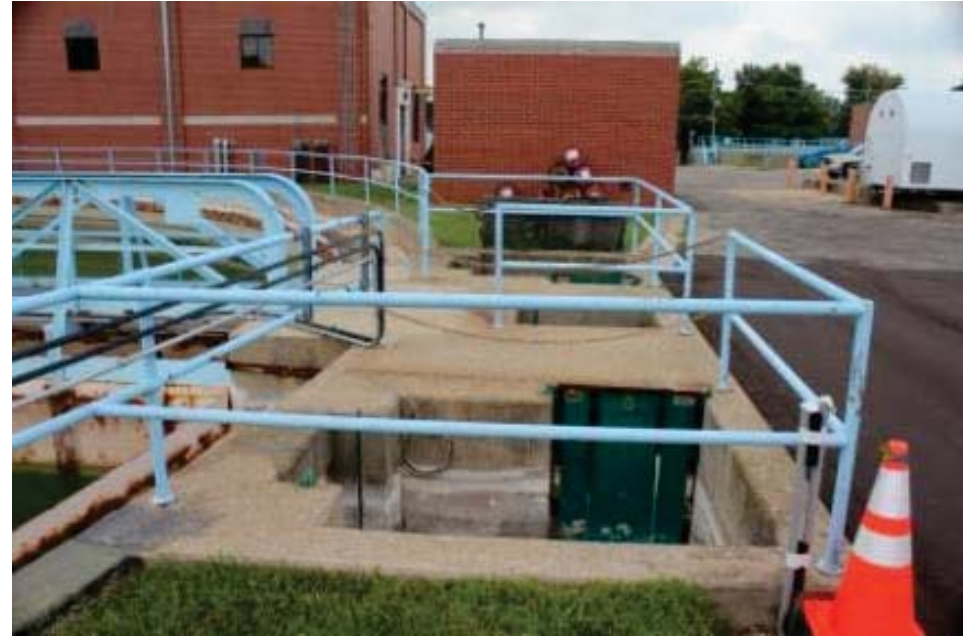
Settling Basin No. 3 Effluent Slide Plates
