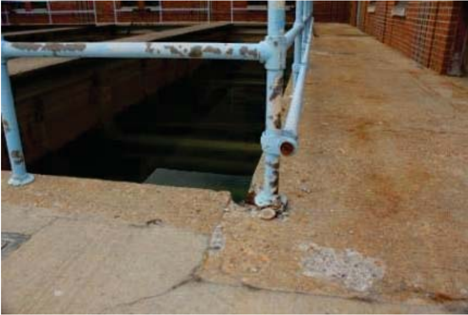
Flocculation Basin No. 3 Stage 1 Cantilevered Concrete Slab
