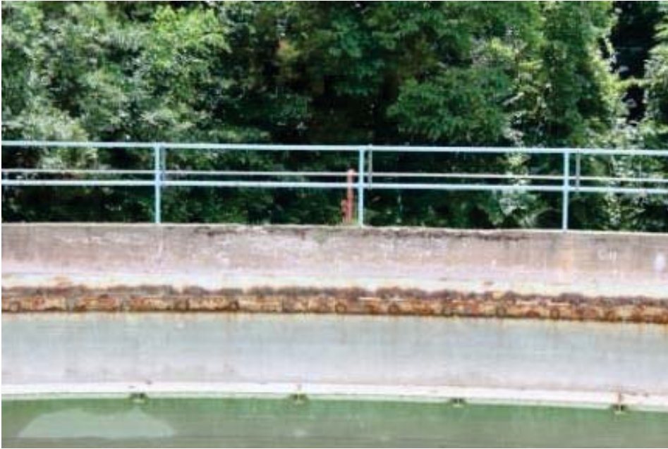
Basin No. 3 Effluent Weir and Effluent Channel
