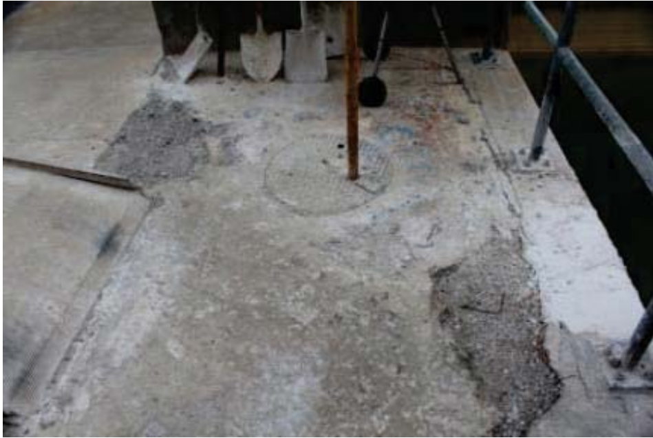
Concrete deck, northeast corner of Basin 1 near Well Influent Chamber
