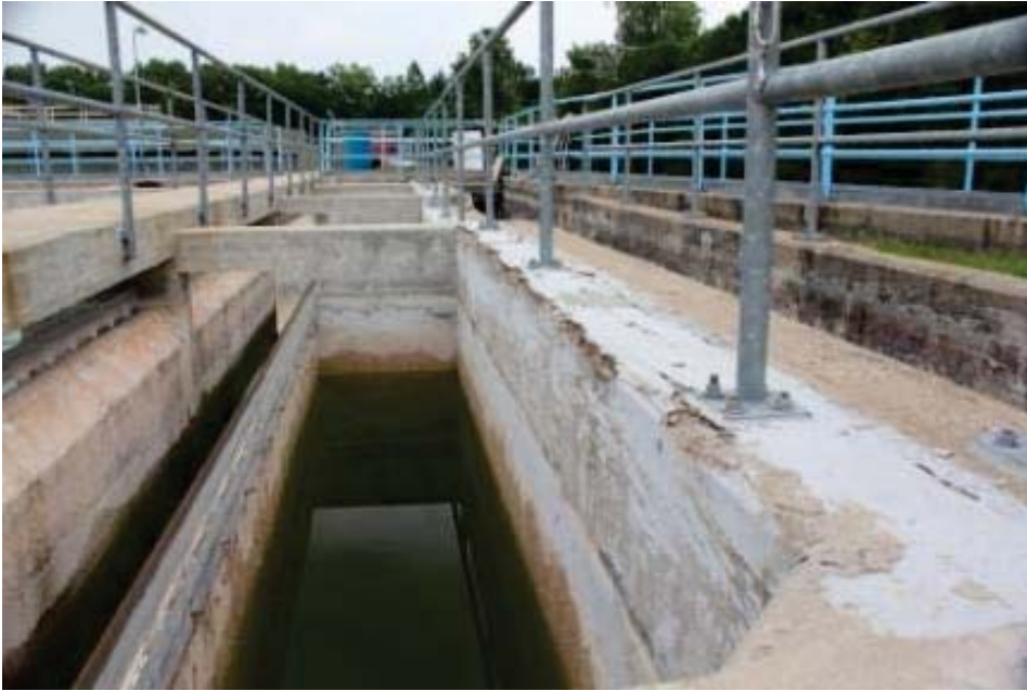
Basin No. 2 Effluent Weirs and Revised Effluent Channel
