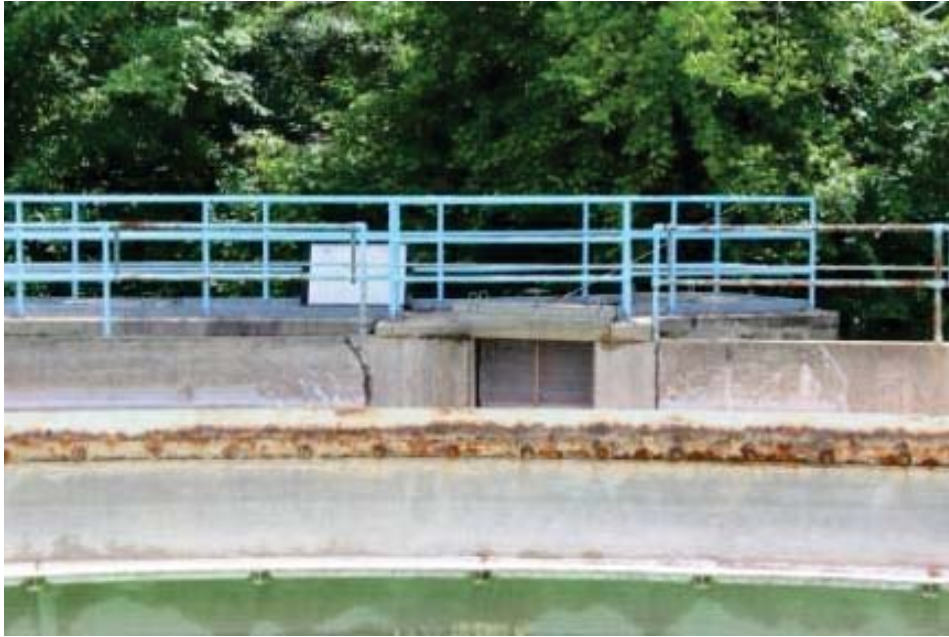
Basin No. 3 South Effluent Structure
