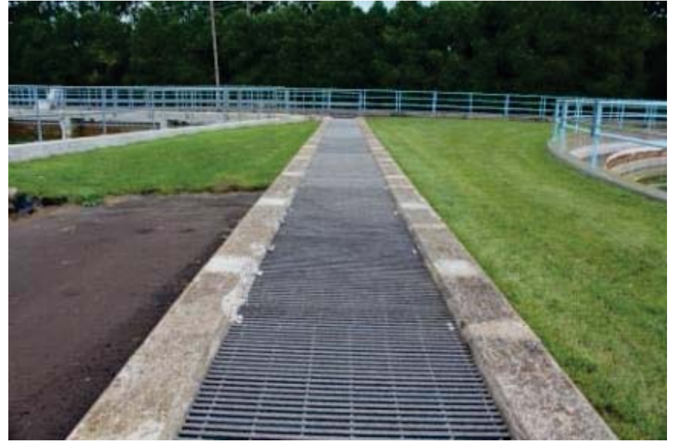
Basin Nos. 1 & 2 Revised Effluent Channel
