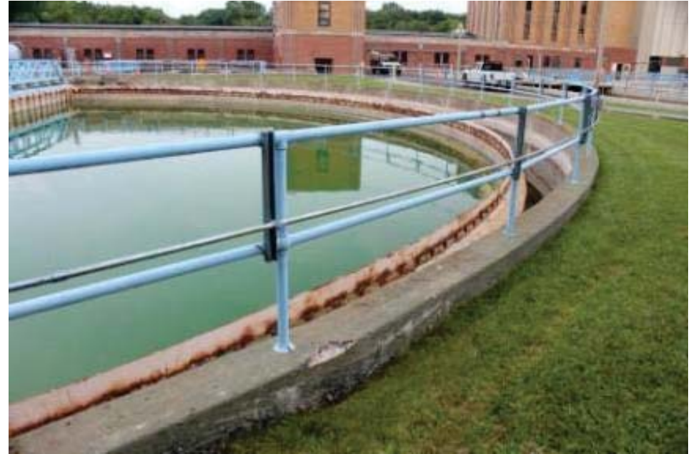
Basin No. 3 Effluent Weir and Effluent Channel
