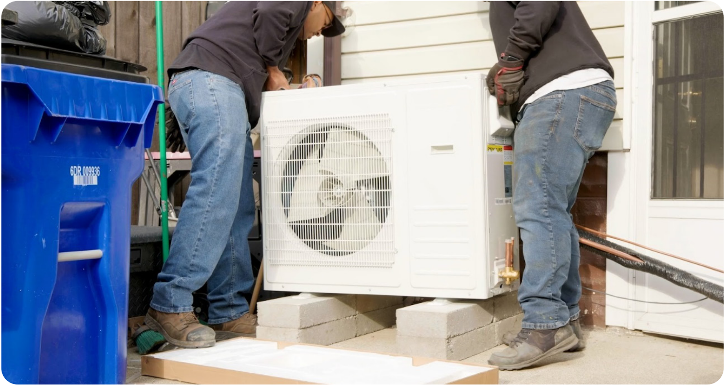
Installation of a heat pump.
