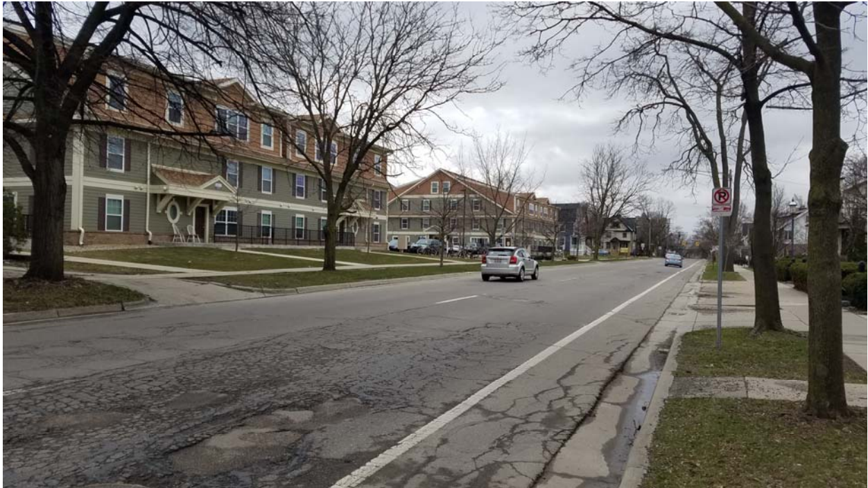
Looking south at Fifth Avenue
