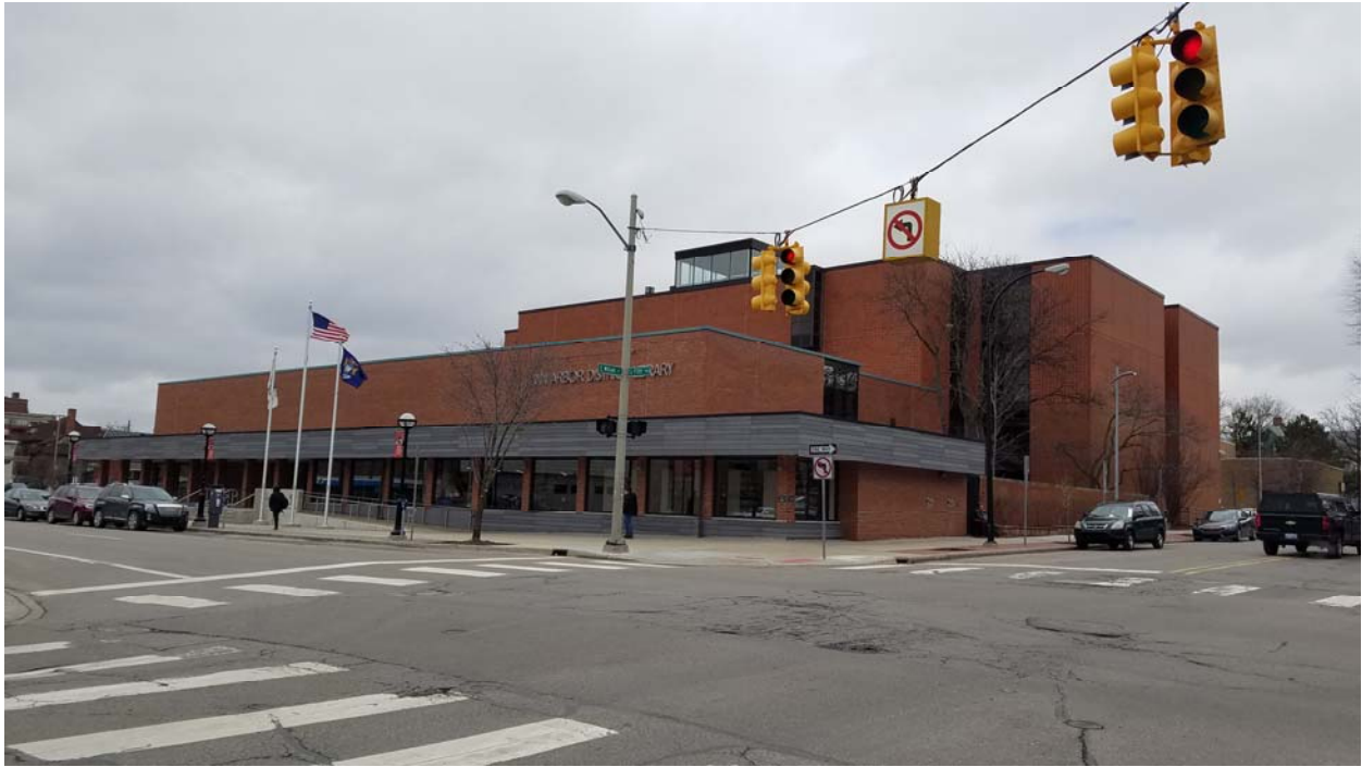
Ann Arbor Public Library across Fifth Avenue from the subject site
