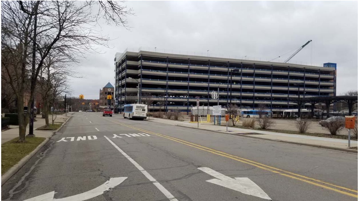
Looking west at William Street
