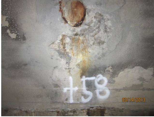
Photo 28 Station 700+58: 6" bulk head, good
