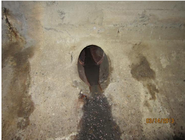
Photo 29 Station 700+65: 12" clay pipe, good
