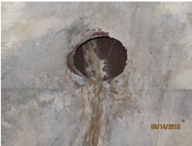
Photo 27 Station 600+30: 4" clay pipe, good condition
