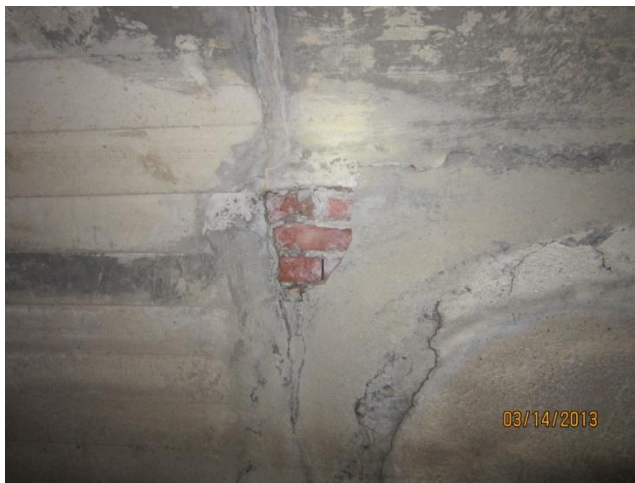
Photo 21 Station 500+11: bulk head
