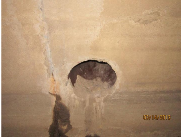
Photo 10 Station 200+82: 12" clay pipe, good
