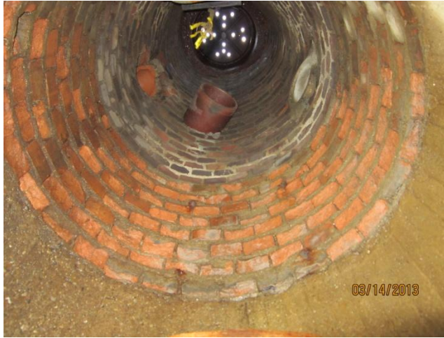
Photo 13 Station 200+95: manhole #1, good condition
