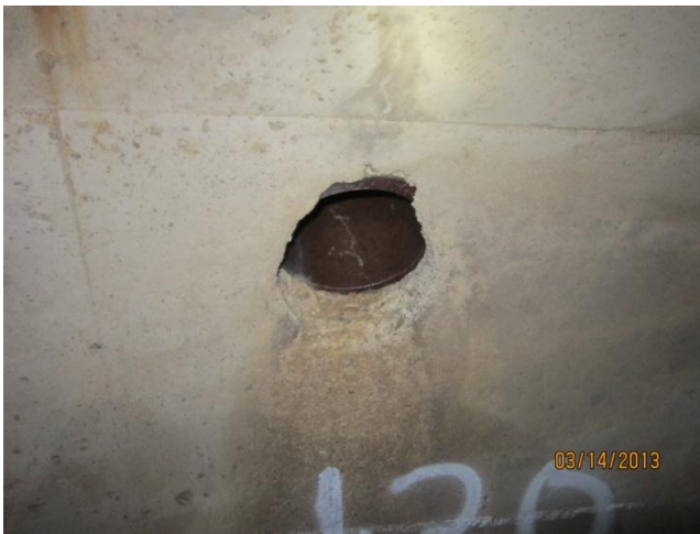
Photo 26 Station 600+30: 4" clay pipe, good
