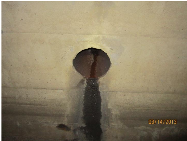
Photo 23 Station 500+22: 12" clay pipe, good
