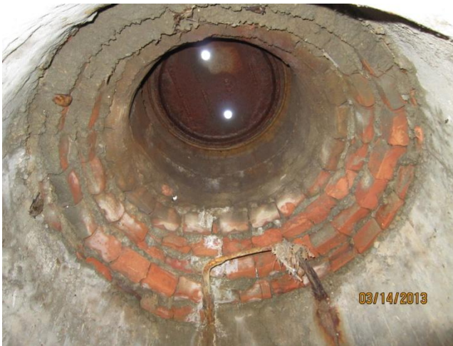
Photo 32 Station 800+20: manhole #2, good condition
