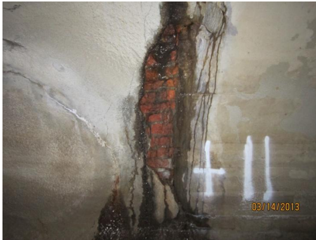
Photo 20 Station 500+11: bulk head, mortar skim
