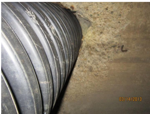
Photo 12 Station 200+95: 12" HDPE pipe, good
