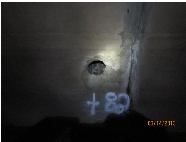
Photo 9 Station 200+82: 6" clay pipe, good condition
