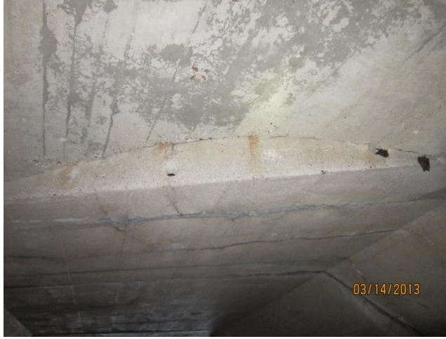
Photo 7 Station 100+90: pipe transition, good
