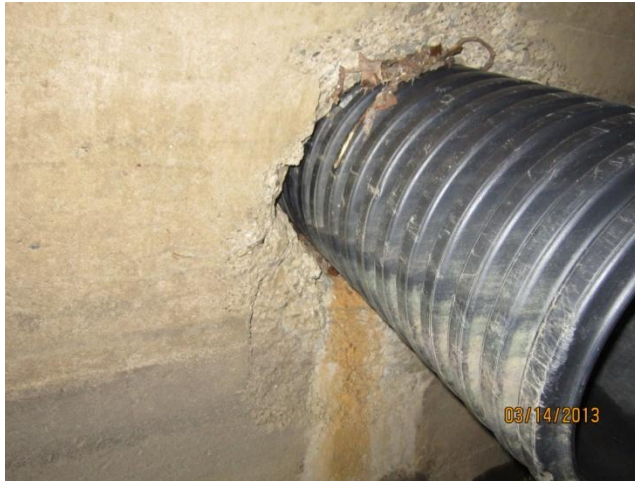
Photo 11 Station 200+95: 12" HDPE pipe, good
