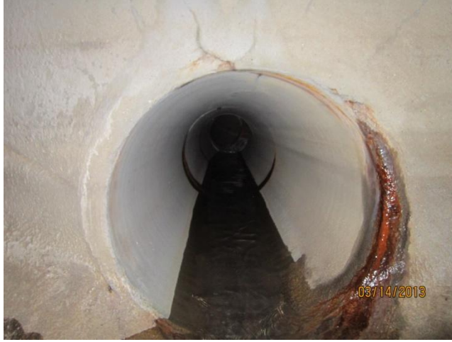
Photo 22 Station 500+20: 36" concrete pipe, good
