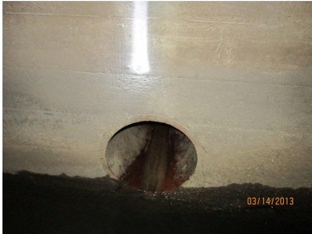
Photo 8 Station 200+00: 12" clay pipe, good condition
