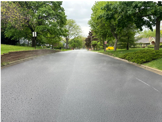
Hawthorn Road Street Resurfacing Project
