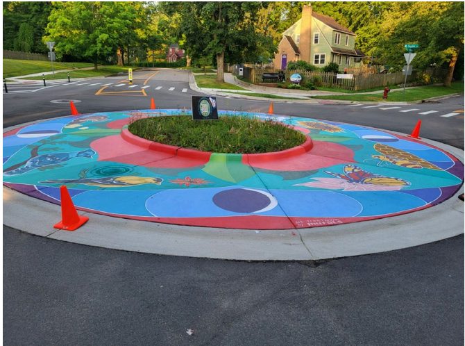
Eberwhite Roundabout Installation
