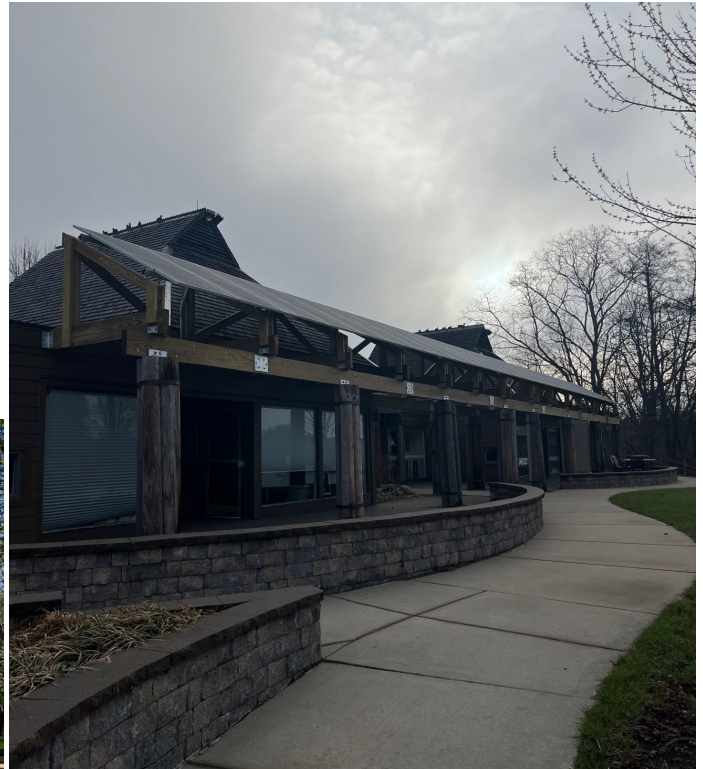
Gallup Livery Solar Panel and Pergola Installation
