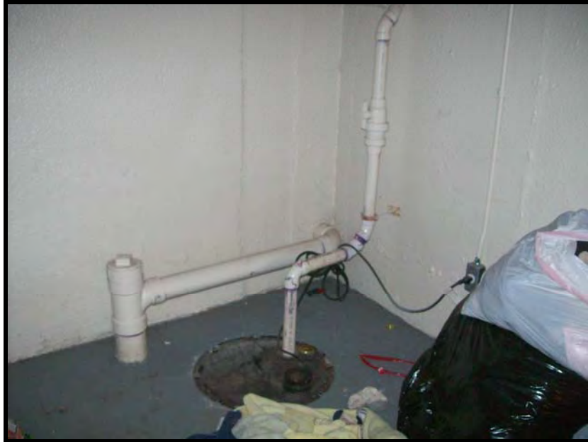
PHOTOGRAPH NO. 6: TYPICAL VIEW OF SUMP LOCATED WITHIN TENANT BUILDING
