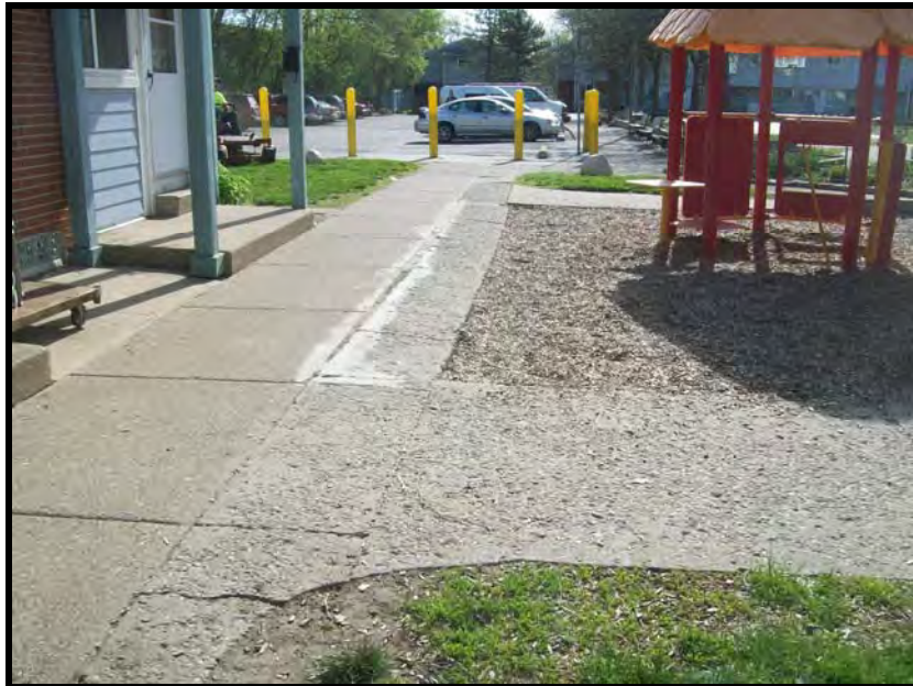
PHOTOGRAPH NO. 4: TYPICAL VIEW OF FLATWORK THROUGHOUT SUBJECT PROPERTY
