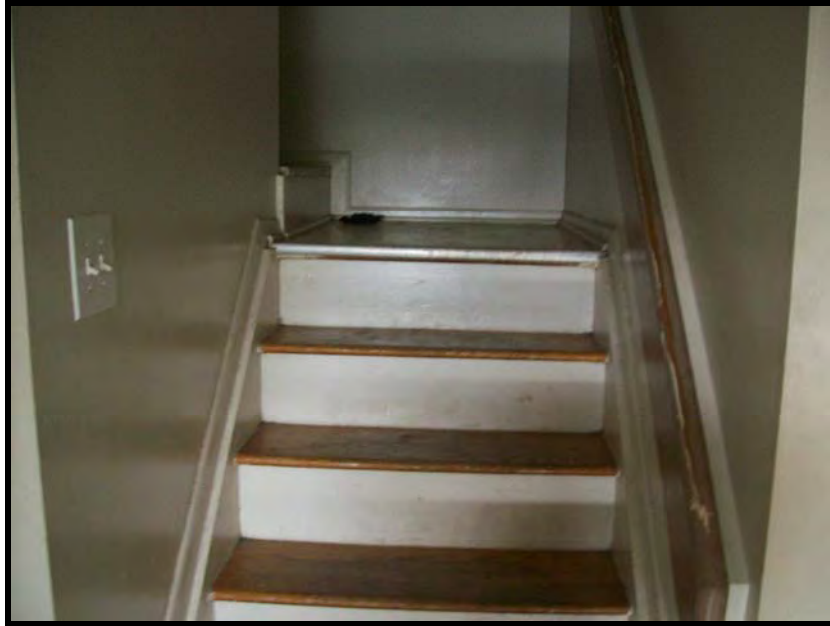
PHOTOGRAPH NO. 17: TYPICAL VIEW OF SECOND STORY TENANT UNIT STAIRS
