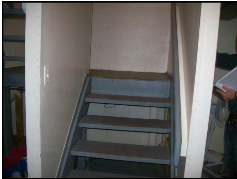
PHOTOGRAPH NO. 8 TYPICAL VIEW OF BASEMENT STAIRS IN TENANT UNITS
