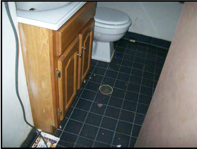
PHOTOGRAPH NO. 15: TYPICAL VIEW OF TENANT UNIT BATHROOMS
