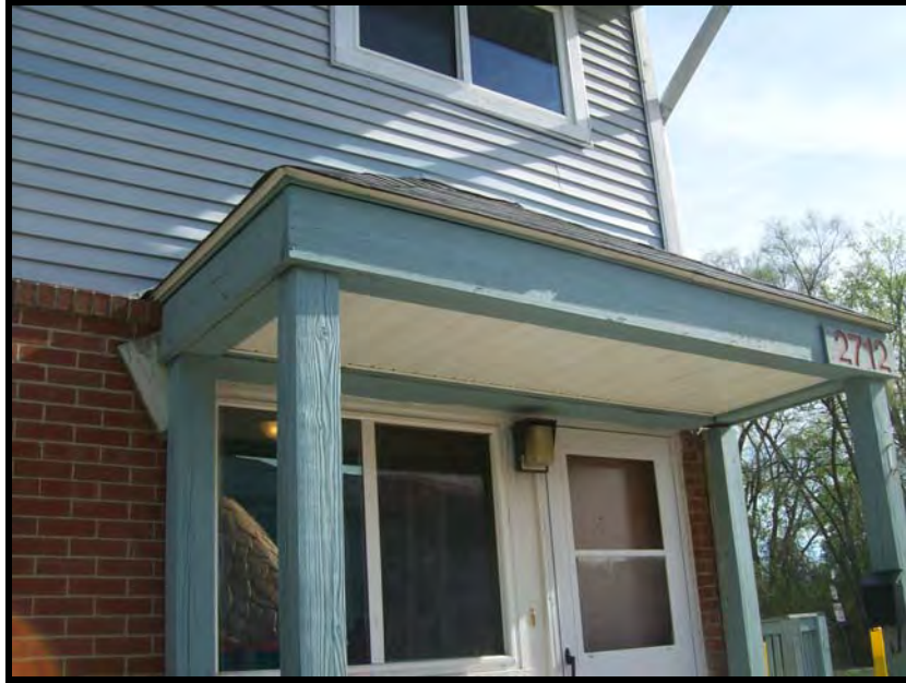
PHOTOGRAPH NO. 3: TYPICAL VIEW OF WOODEN PORCHES ASSOCIATED WITH TENANT UNITS
