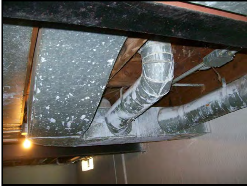
PHOTOGRAPH NO. 12: TYPICAL VIEW OF DUCTWORK AND IN TENANT UNIT BASEMENT
