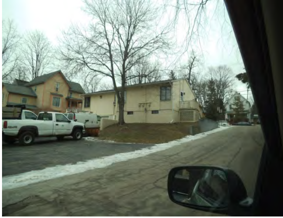
Photo 1: Exterior view of the complex back
