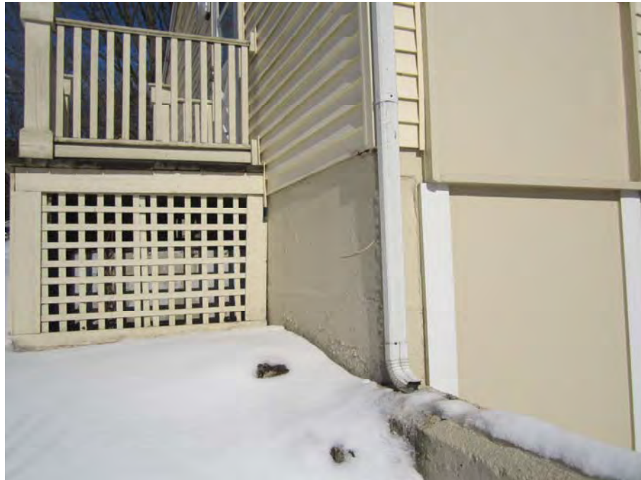
PHOTOGRAPH NO. 18: VIEW OF ALUMINUM DOWNSPOUT
