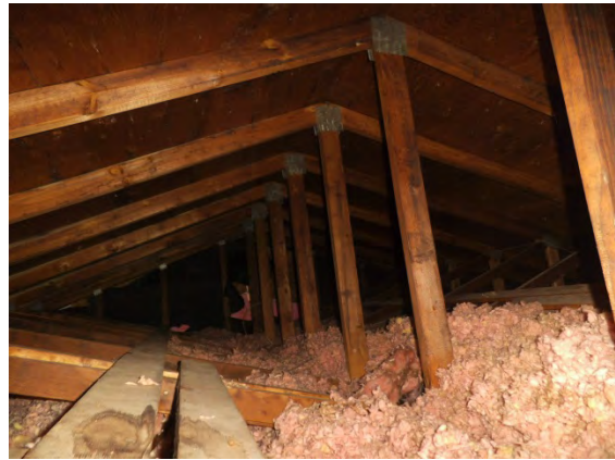
Photo 16: Roof frame in attic space
