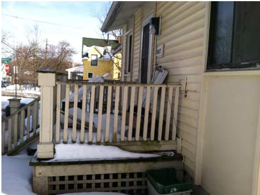
PHOTOGRAPH NO. 6: TYPICAL SIDE VIEW OF WOOD PORCH
