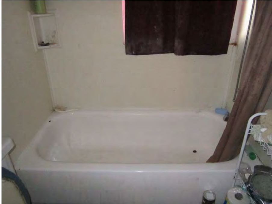
PHOTOGRAPH NO. 11: TYPICAL VIEW OF BATHTUB IN TENANT UNIT BATHROOM
