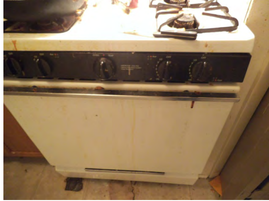
Photo 8: Gas range and oven in kitchen
