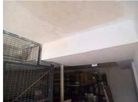
Unconditioned Maintenance Garage - ceiling
