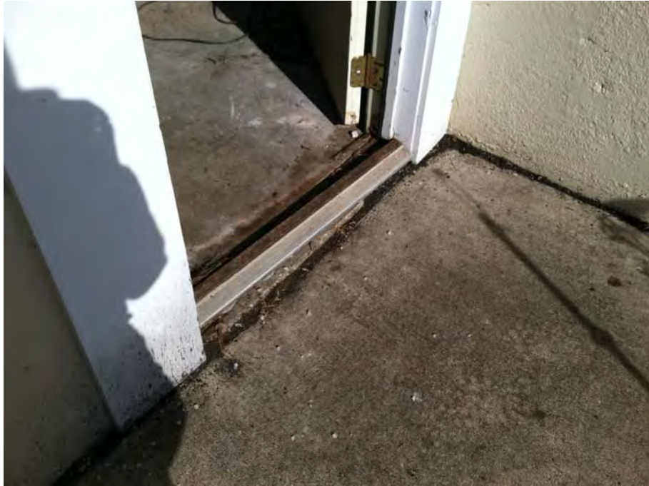
PHOTOGRAPH NO. 17: VIEW OF ENTRANCEWAY TO GARAGE/BASEMENT AREA
