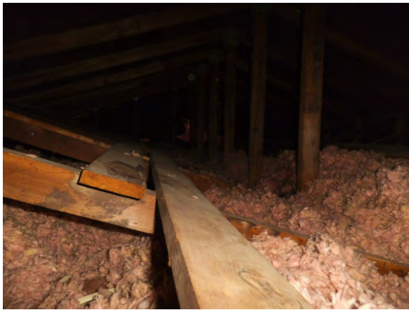
Photo 15: Fiberglass blown insulation in attic
