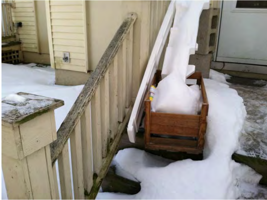
PHOTOGRAPH NO. 7: VIEW OF WOOD PORCH STAIRWELL AND RAILING
