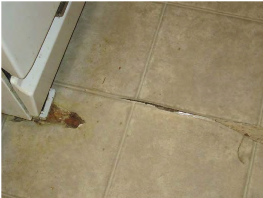
PHOTOGRAPH NO. 10: TENANT UNIT FLOORING IN KITCHEN (805)
