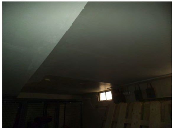
Photo 18: Basement window in storage room
