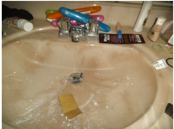
Photo 14: Bathroom faucet with aerator
