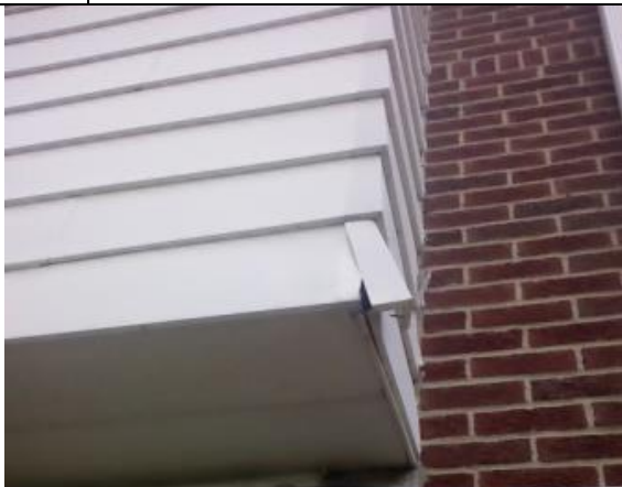
Photo #33: Corner siding piece pulled away. Provides potential entry point for pests.
