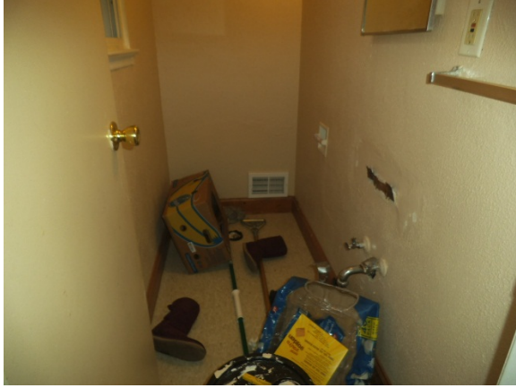
Photo 13: Unfinished bathroom in complex unit
