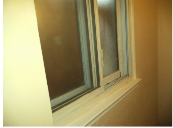
Photo 14: Typical horizontal sliding window frame
