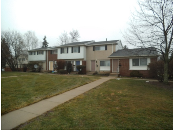
Photo 1: Exterior view of the complex
