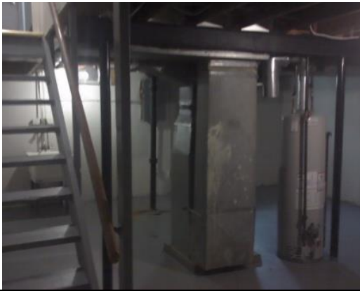
Photo #19: Typical two bedroom unit, basement
