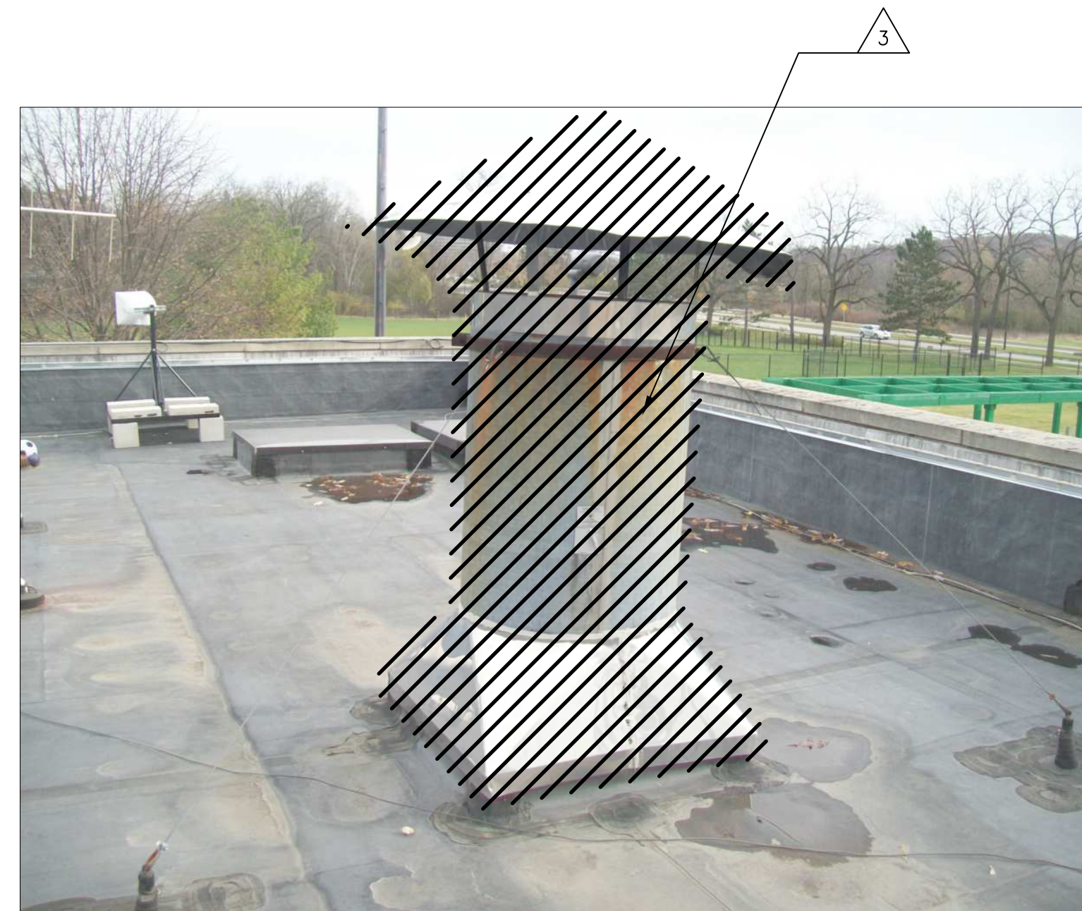
PHOTO No.4 - BOILER STACK
