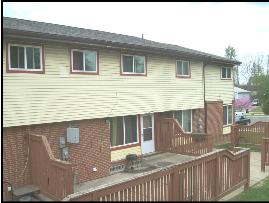
PHOTOGRAPH NO. 3: TYPICAL VIEW OF WOODEN PRIVACY FENCES
