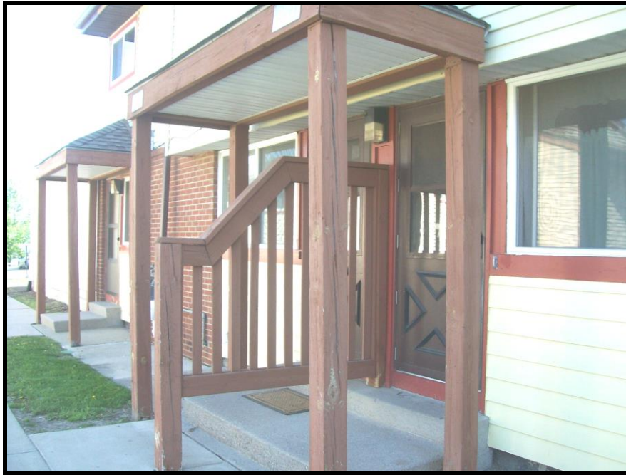
PHOTOGRAPH NO. 7: TYPICAL VIEW OF PORCHES ASSOCIATED WITH TENANT UNITS
