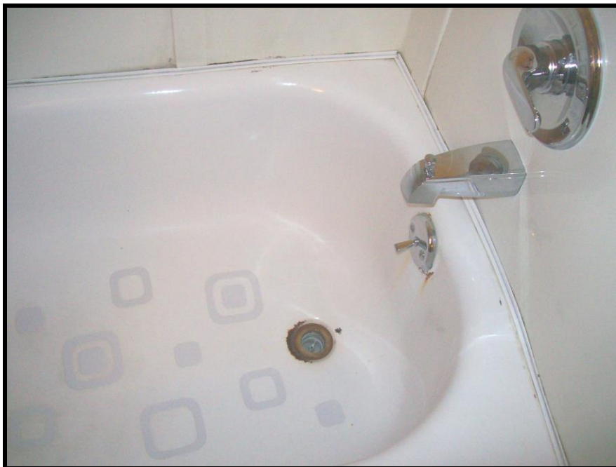
PHOTOGRAPH NO. 16: TYPICAL VIEW OF BATHTUB AND ASSOCIATED VINYL ENCLOSURE
