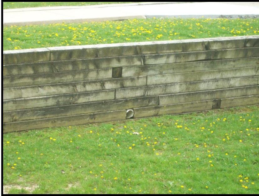
PHOTOGRAPH NO. 5: TYPICAL VIEW OF WOODEN RETAINING WALL
