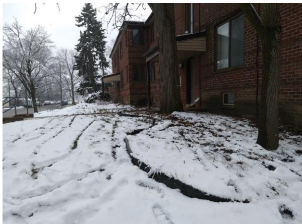
Photo from East side of building investigated
