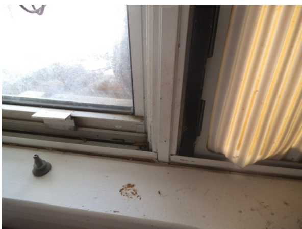
Photo 11: Interior window frame of typical window
