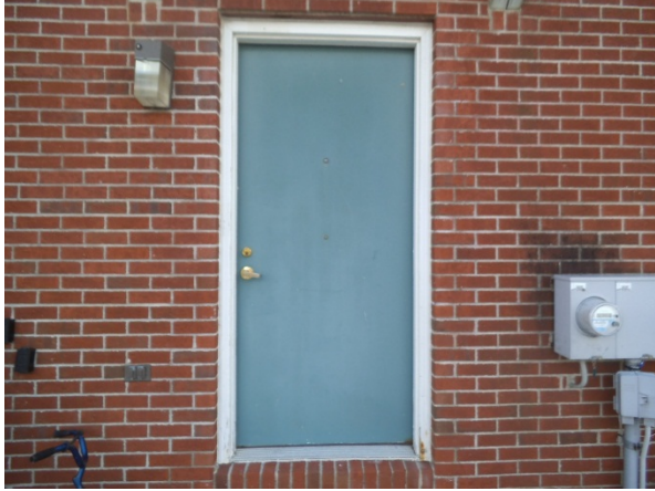
Photo 7: Typical side door and exterior lighting
