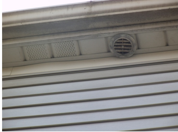
Photo 8: Soffit vents above second floor of building
