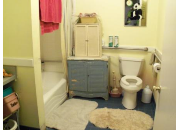
Photo #8: Bathroom, Unit 1020 Typical 3 bedroom
