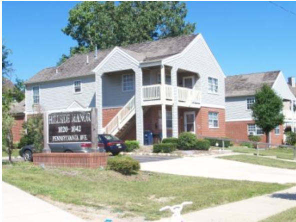
Photo #1: Street elevation
