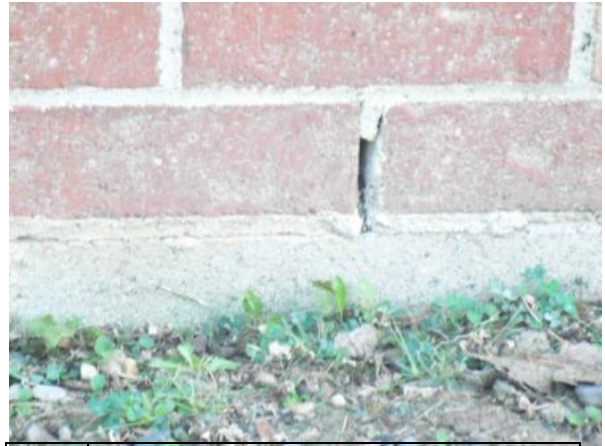
Photo #26: Weep holes should have screen in them to prevent pest entry.
