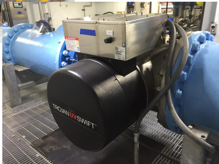
Temporary Ultraviolet Disinfection Project at the Water Treatment Plant
