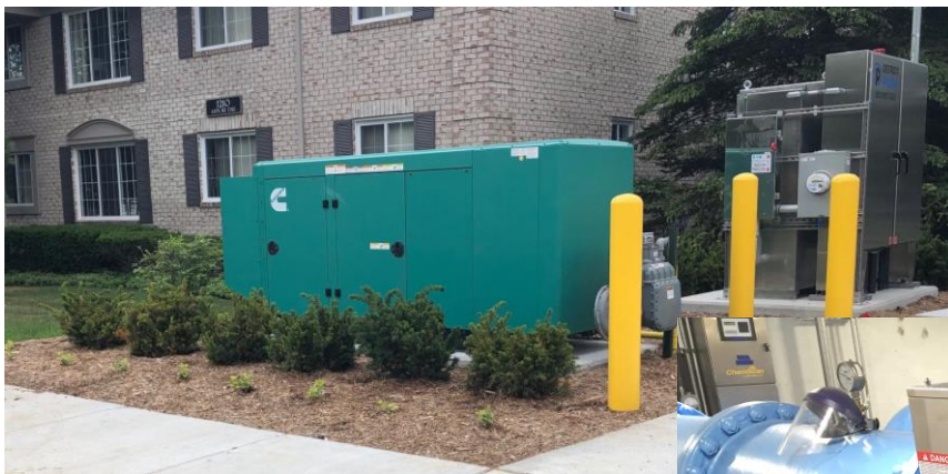
Astor Valve Vault Project
