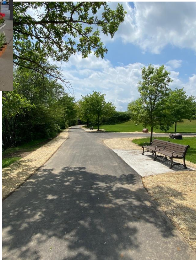
Gallup Park Loop Trail Resurfacing Project
