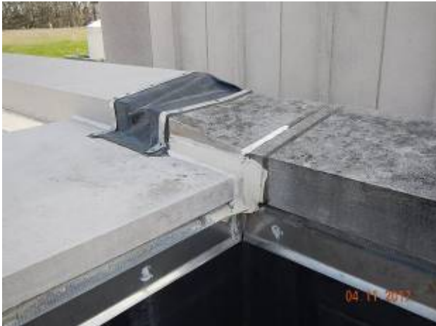
Admin Building – AD-1
