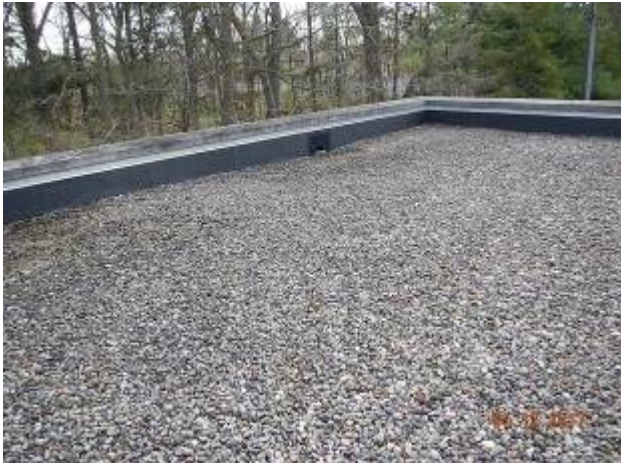
Maintenance Building – M-1
