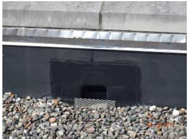
Re-carb Building – RC-1
