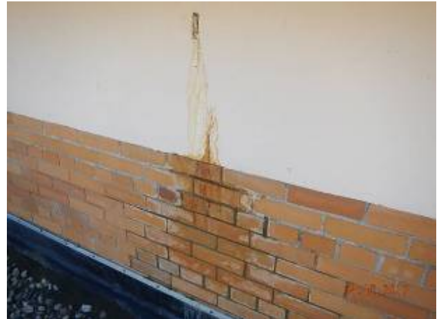
Barton Pumping Station
