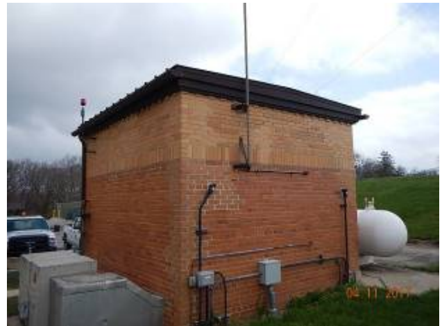
Ammonia Building – A-1
