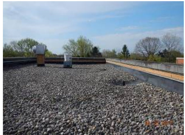
Carbon House – CH-1 Overview of the roof area.
