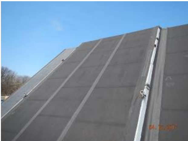
Superior Hydroelectric Pumping Station
