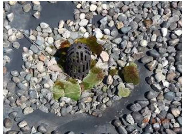
Barton Pumping Station
