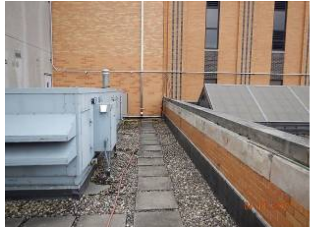
Control Rooms – CR-2 Overview of the roof area.
