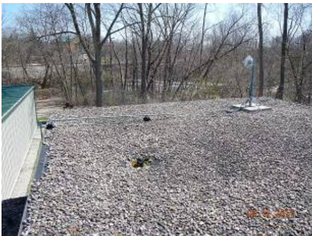
Barton Pumping Station
