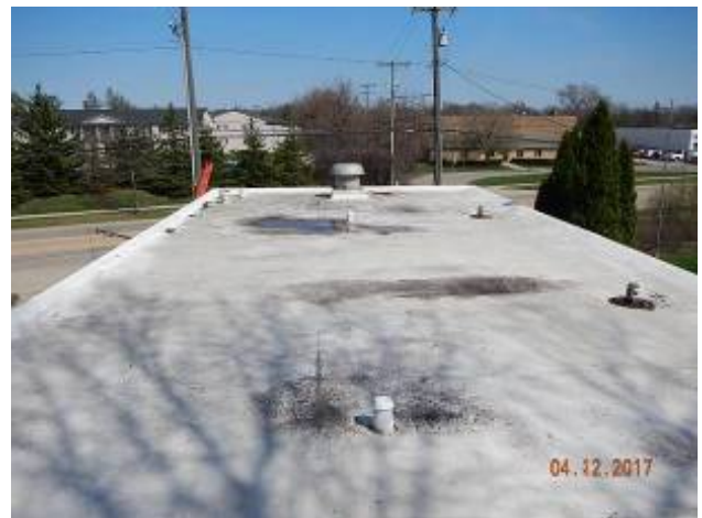
Industrial Pumping Station
