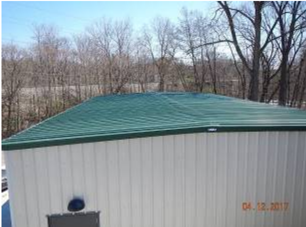
Barton Pumping Station
