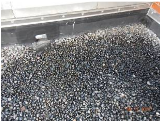
Admin Building – AD-2 Overview of the roof area.
