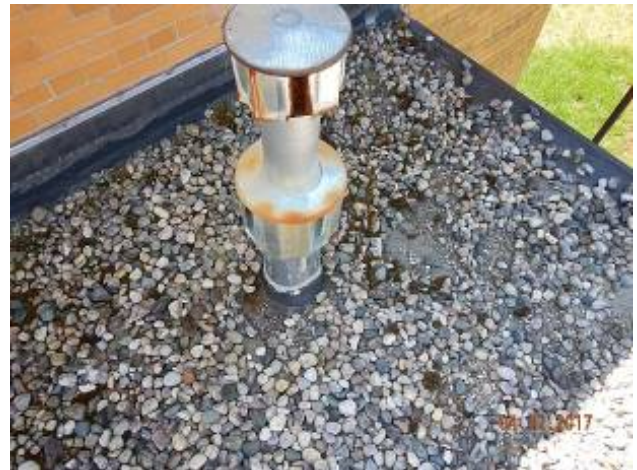
Barton Pumping Station
