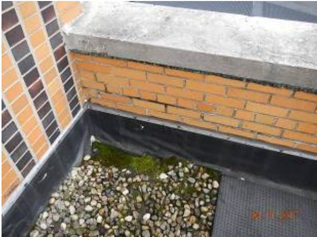
Control Rooms – CR-1
