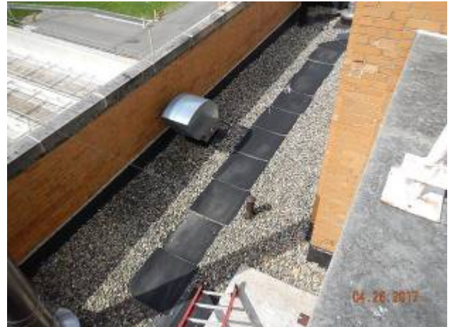
Penthouse – P-1 Overview of the roof area.
