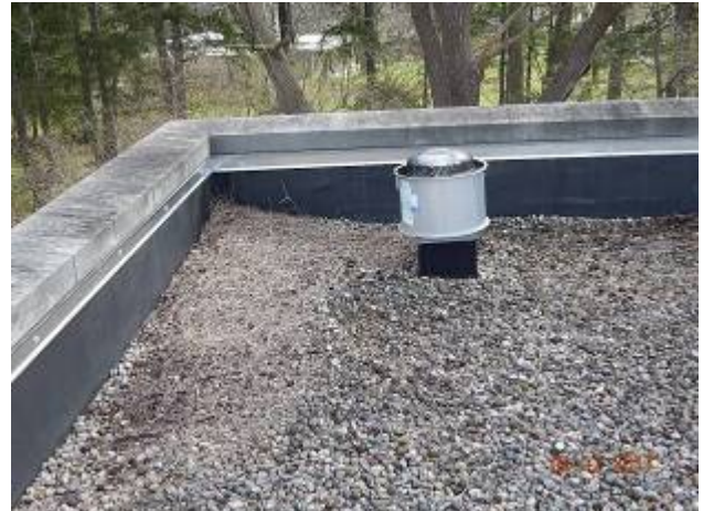
Maintenance Building – M-1
