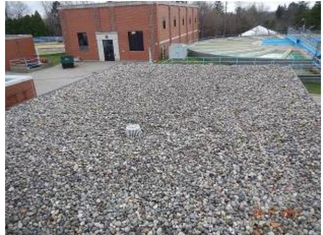
Rapid Mix Building – R-1
