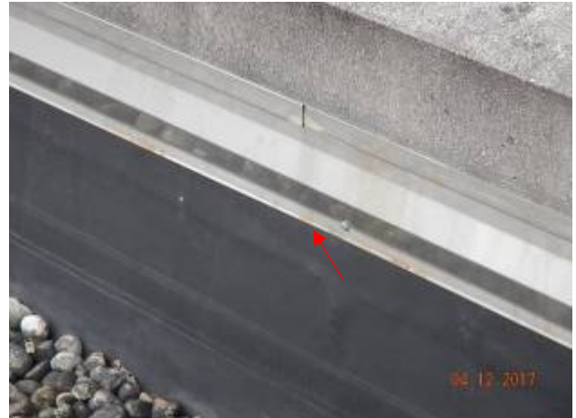
Generator Building – G-1
