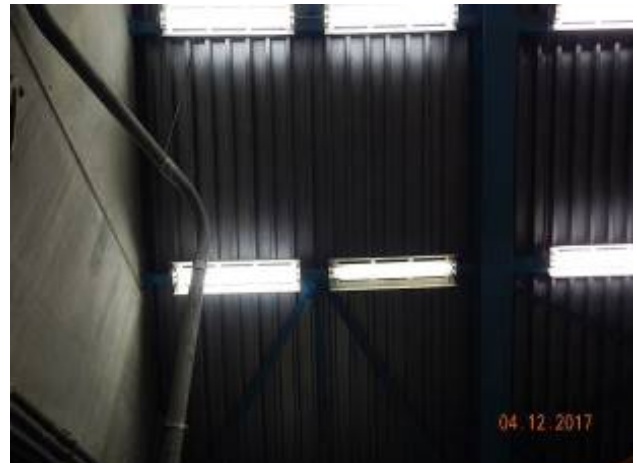
Superior Hydroelectric Pumping Station Interior photo of underside of metal decking.
