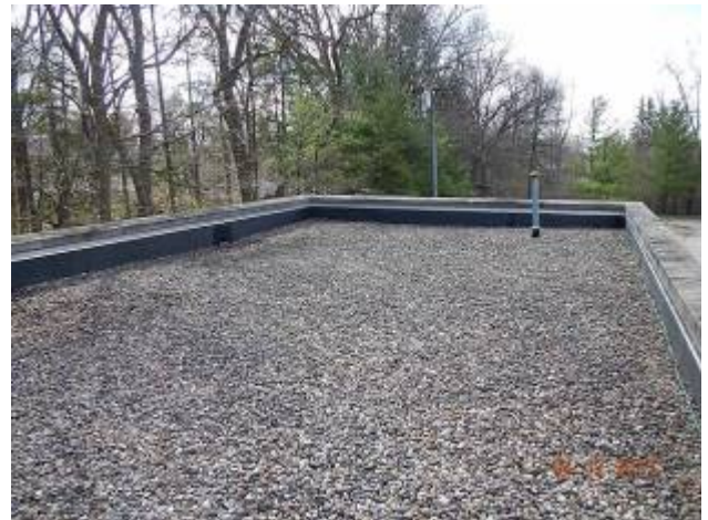
Maintenance Building – M-1
