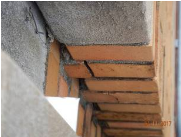
Admin Building – AD-3
