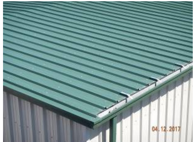
Barton Pumping Station
