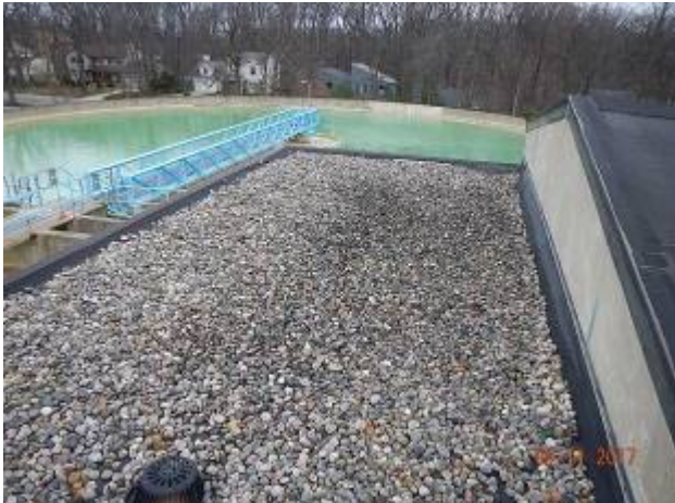
Rapid Mix Building – R-1
