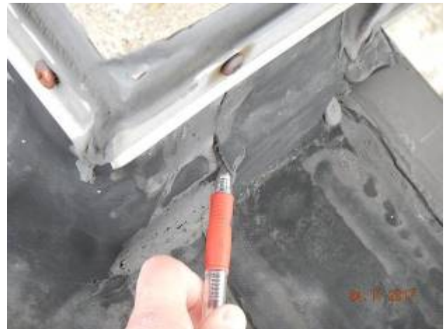
Rapid Mix Building – R-1
