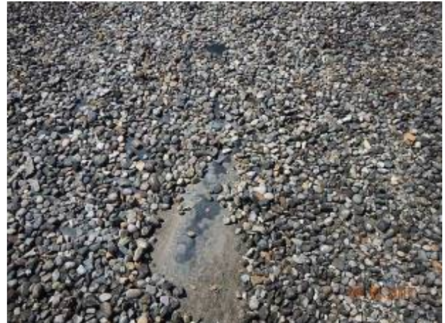
Barton Pumping Station
