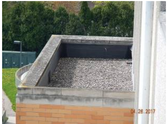
Calciner Building – CA-2 Overview of the roof area.
