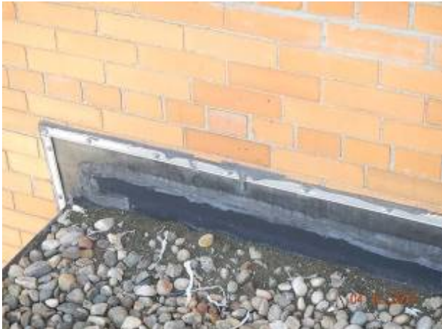
Barton Pumping Station
