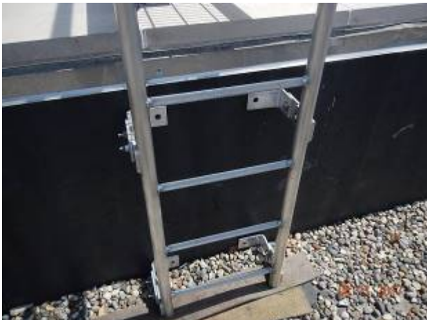
Admin Building – AD-1
