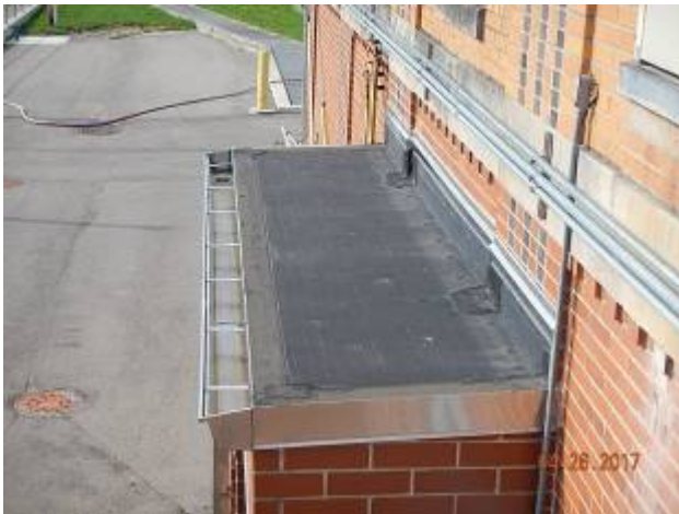
Carbon House – CH-2 Overview of the roof area.
