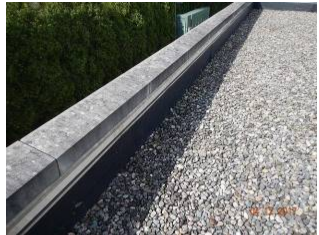
Generator Building – G-1 Overview of the roof area.
