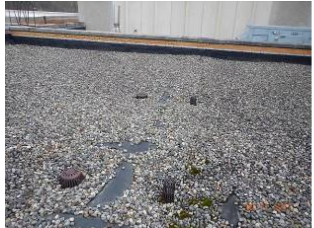
Control Rooms – CR-1
