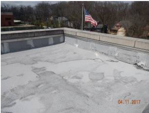
Admin Building – AD-3
