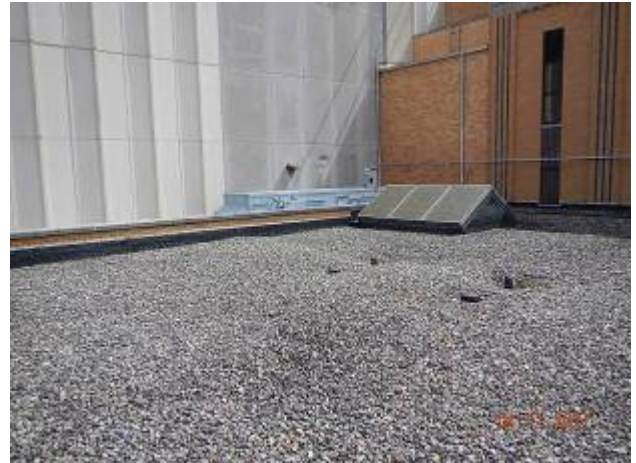
Control Rooms – CR-1 Overview of the roof area.
