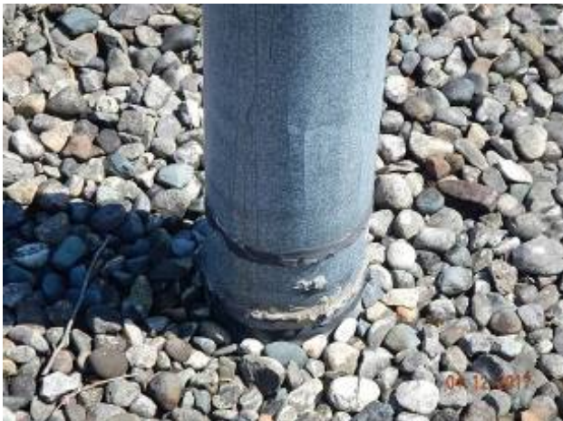
Barton Pumping Station
