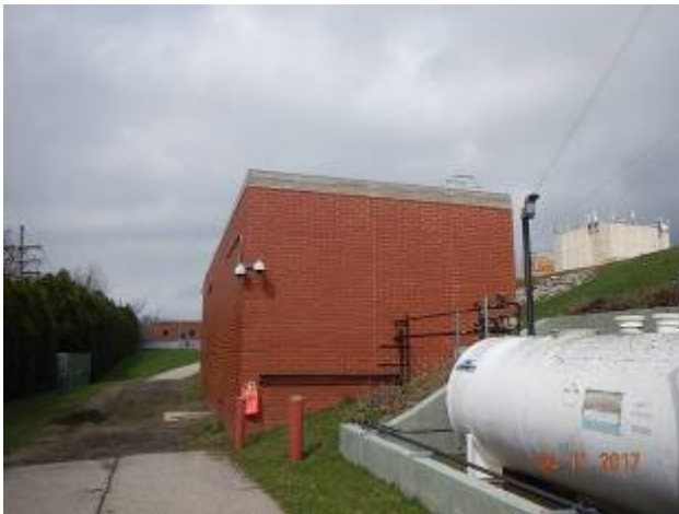
Generator Building – G-1 Overview of the generator building.
