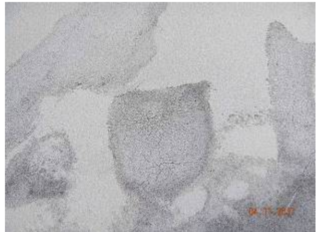
Admin Building – AD-3
