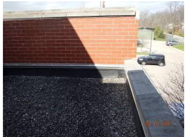
Admin Building – AD-2
