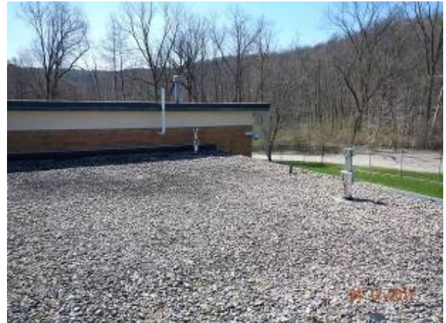
Barton Pumping Station
