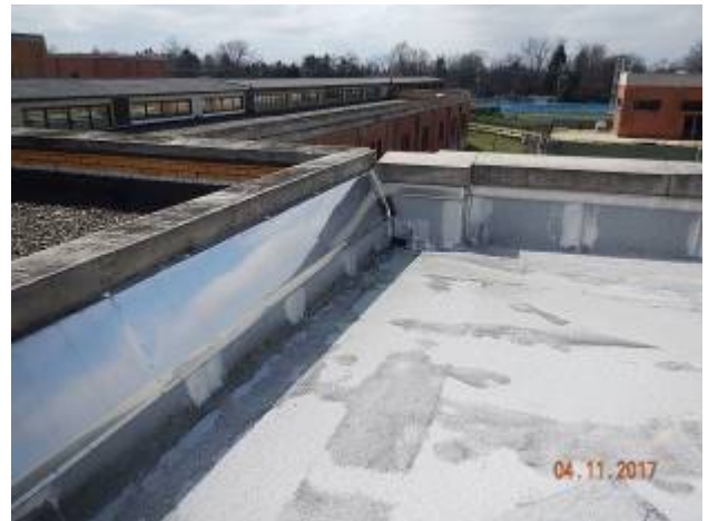
Admin Building – AD-3
