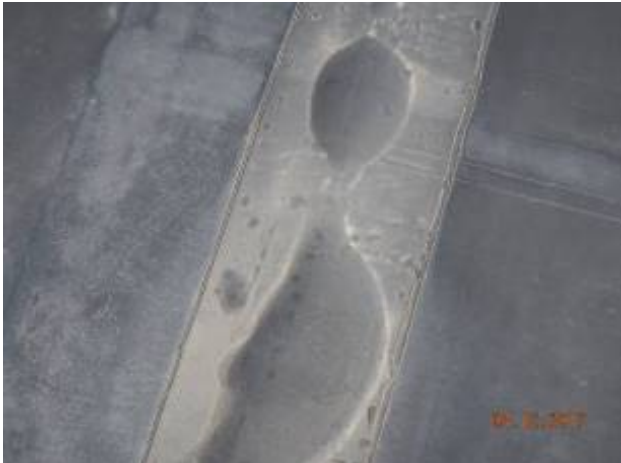
North Campus Pumping Station
