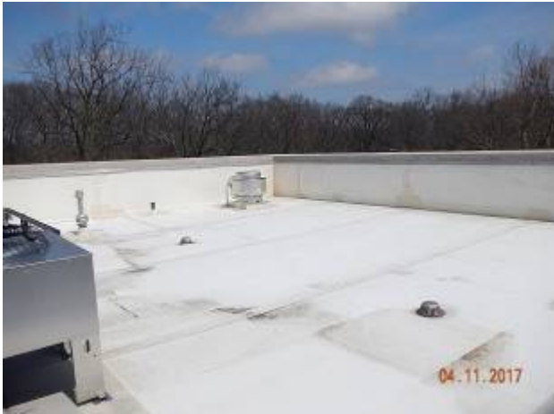
WHS Building – WHS-1 Overview of the roof area.
