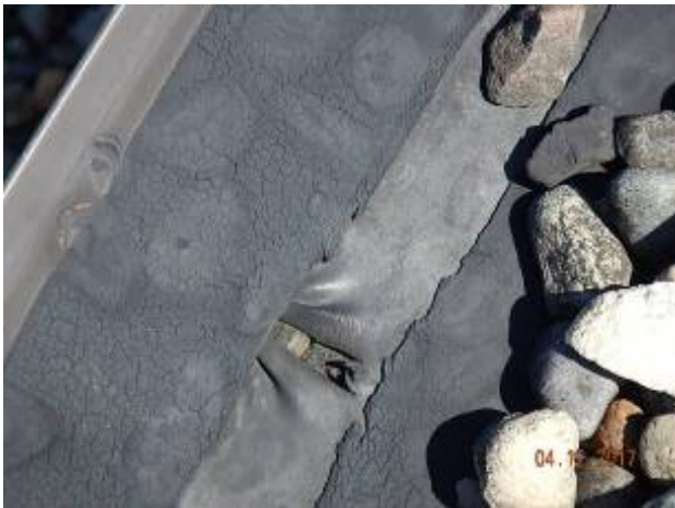
Barton Pumping Station
