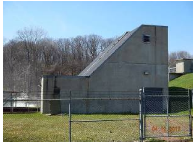
Superior Hydroelectric Pumping Station
