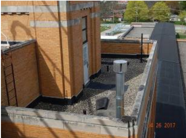
Penthouse – P-1 Overview of the roof area.
