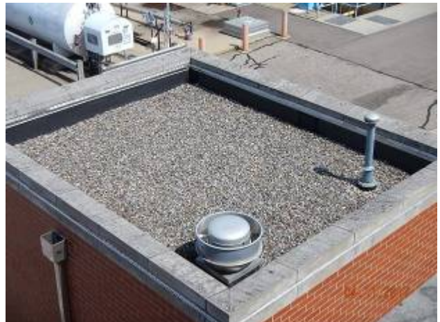
Re-carb Building – RC-1
