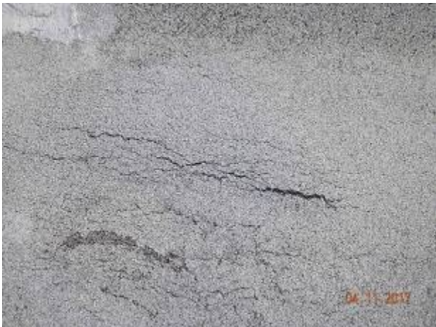
Admin Building – AD-3
