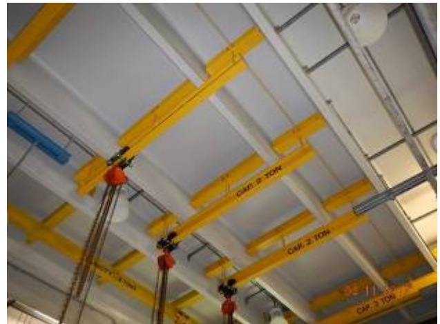
Ozone Building Interior photo of underside of pre-cast concrete decking.
