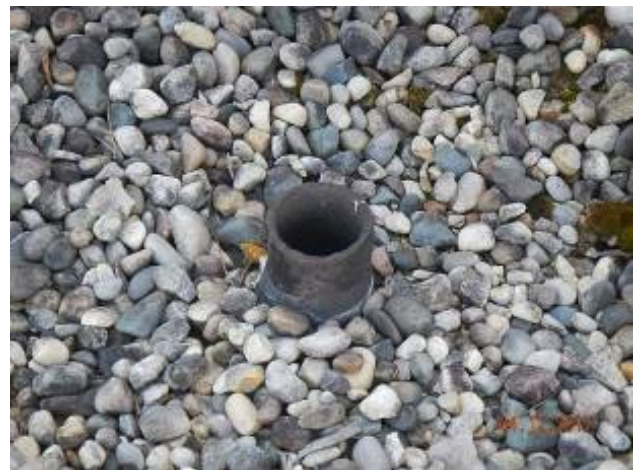
Barton Pumping Station
