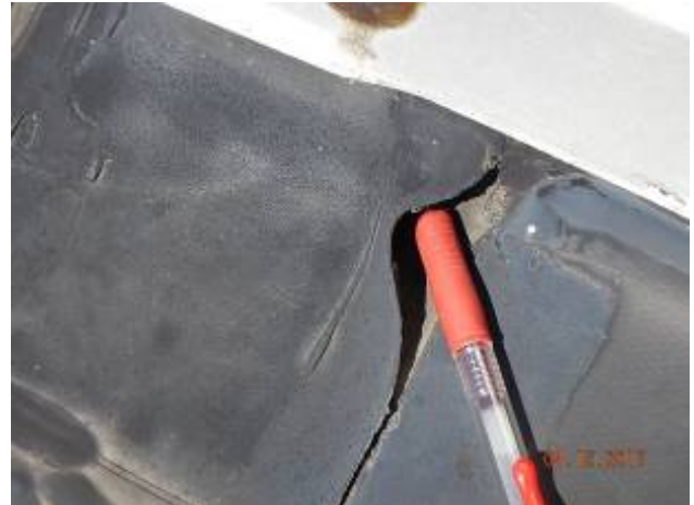
North Campus Pumping Station
