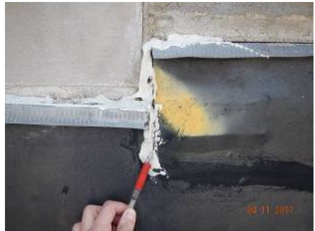
Admin Building – AD-1
