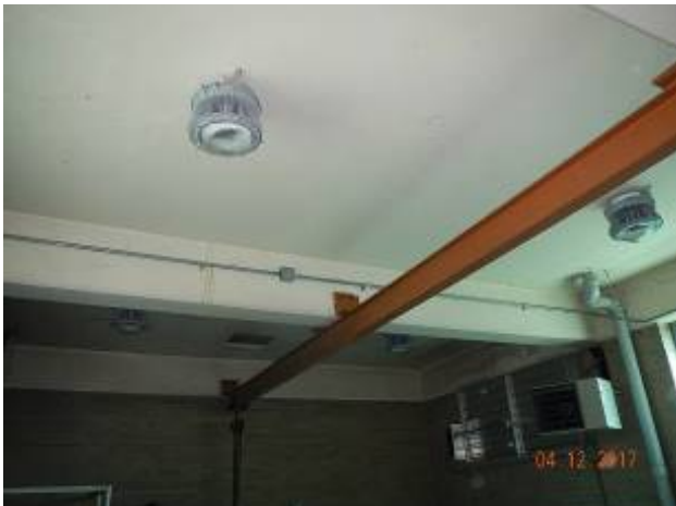
Industrial Pumping Station Overview of underside of concrete decking.
