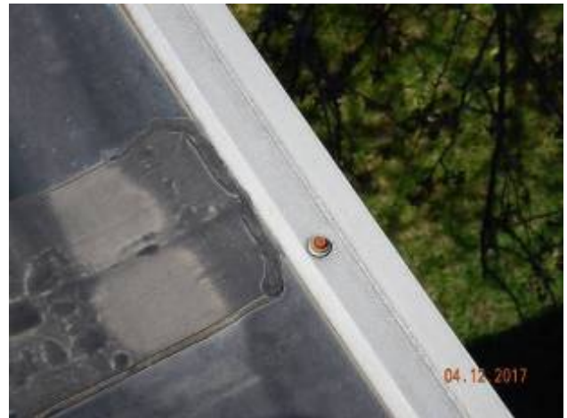
North Campus Pumping Station
