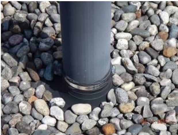
Admin Building – AD-1
