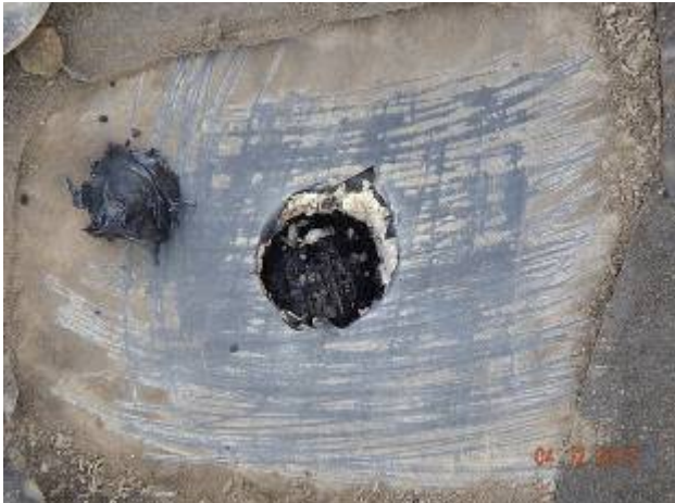
Core Sample – Control Room – CR-1
