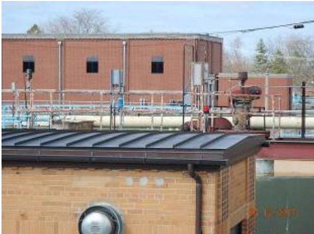
Ammonia Building – A-1 Overview of the roof area.
