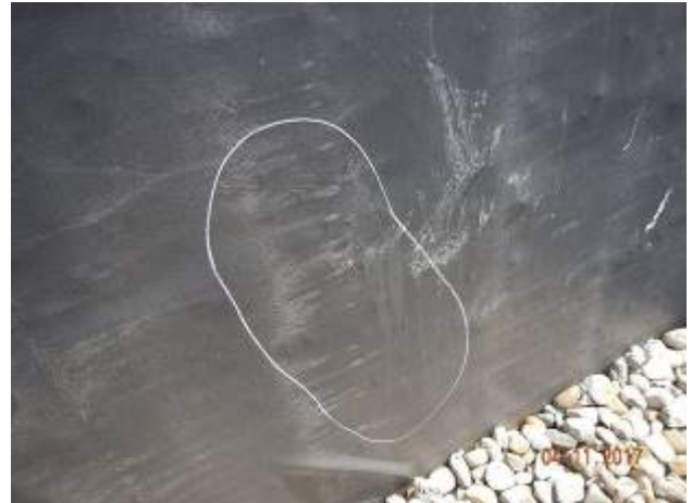
Admin Building – AD-1
