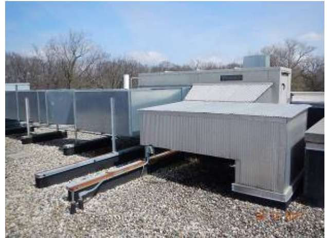
Admin Building – AD-1 Overview of the roof area.
