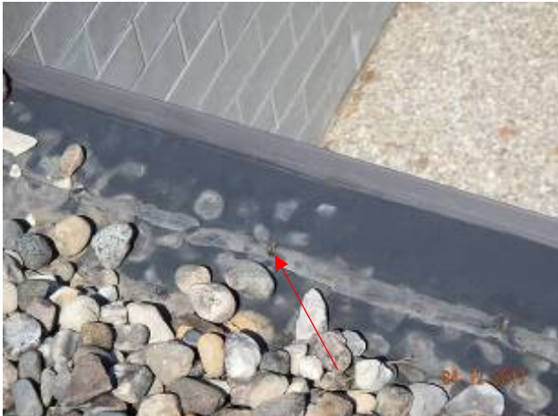
Barton Pumping Station
