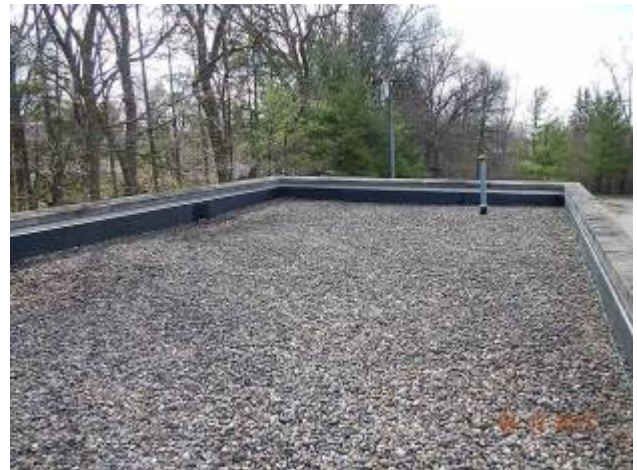
Maintenance Building – M-1
