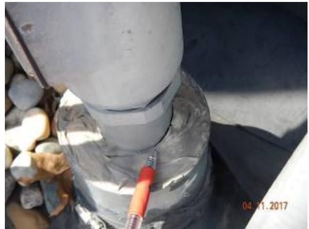
Admin Building – AD-1
