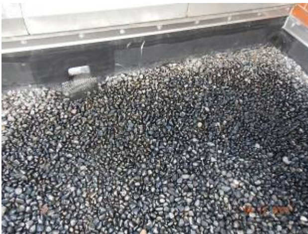
Admin Building – AD-2 Overview of the roof area.
