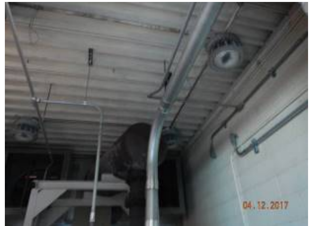
Industrial Pumping Station Overview of underside of metal decking.
