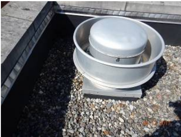
Re-carb Building – RC-1
