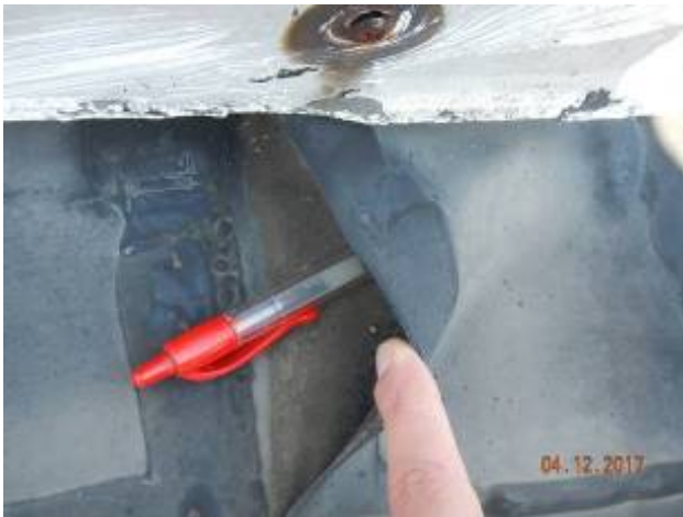
North Campus Pumping Station
