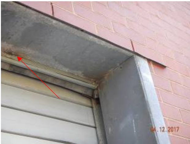
Maintenance Building – M-1
