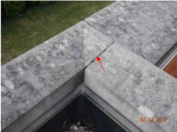
Generator Building – G-1
