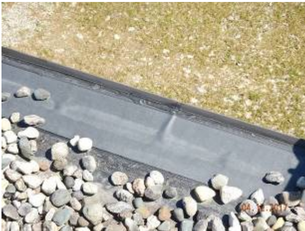
Barton Pumping Station
