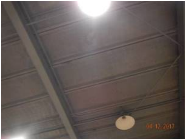
North Campus Pumping Station
