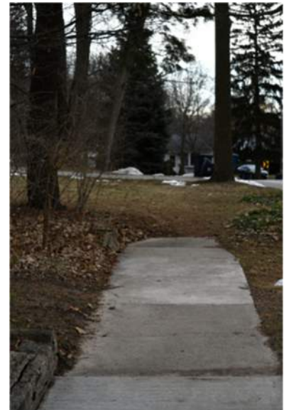
Figure 17: Sidewalks End Without Advance Notice to Users
