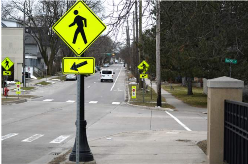
Figure 57: The transition from the Division Street bike lane to the Broadway Street Bridge shared use path is not continuous or marked. The Division Street bike lane ends before Carey Street and there is not an easy entrance for bikes to enter the bridge path.
