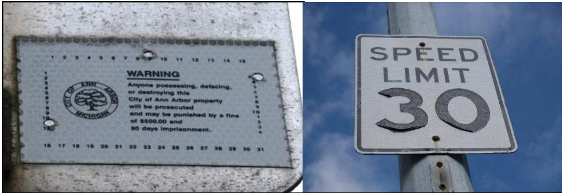
Figure 73: There are older signs throughout the Study Area that lack adequate retro-reflectivity, making them hard to see at night.
