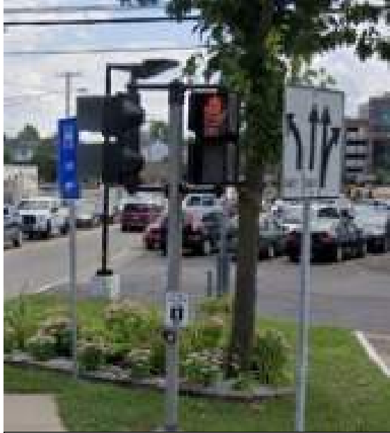
Figure 84: Pedestrian signal heads were noted that lack countdown feature.
