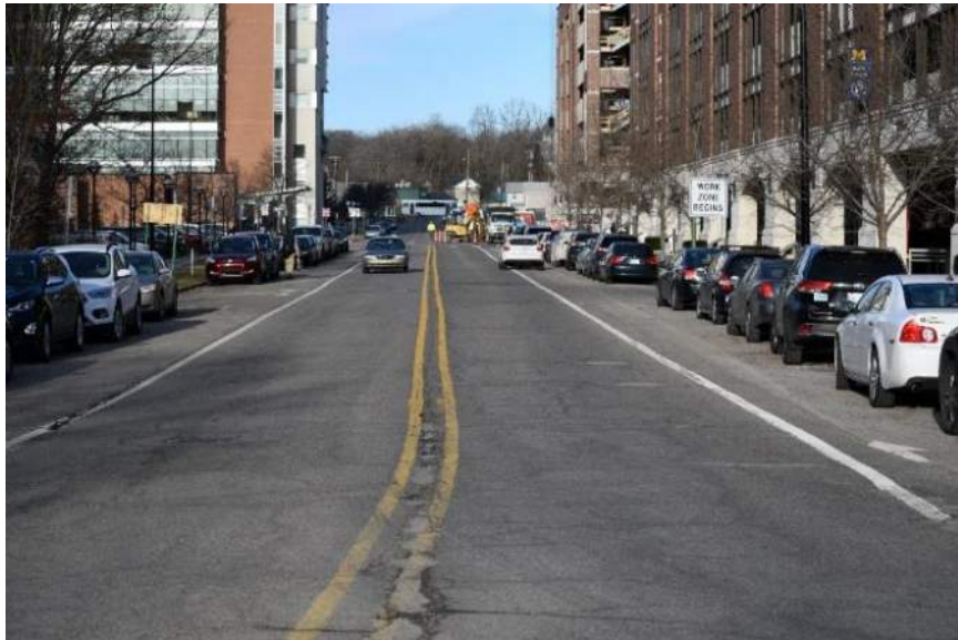
Figure 97: Wall Street – Typical section is 2 vehicle lanes, parking allowed both sides, bike lanes both sides, sidewalk both sides, utilities underground.
