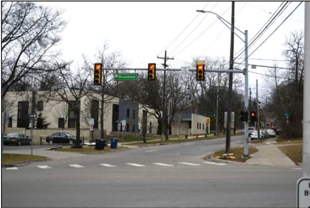
Figure 86: Install box span-wire mounted or mast arm mounted signals to improve visibility and safety.
