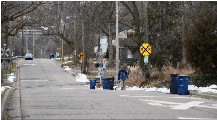
Figure 15: Pedestrian Walking in Roadway Due to Absence of Sidewalk
