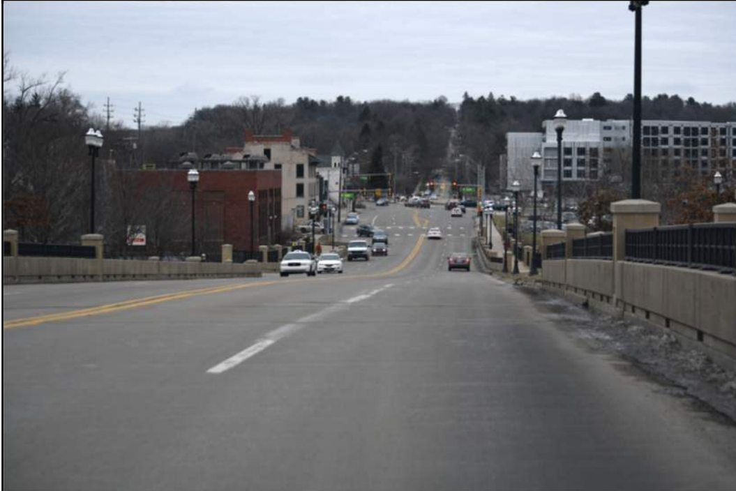
Figure 40: The continuous down-grade for NB Broadway exacerbates the poor observance of the posted speed limit.
