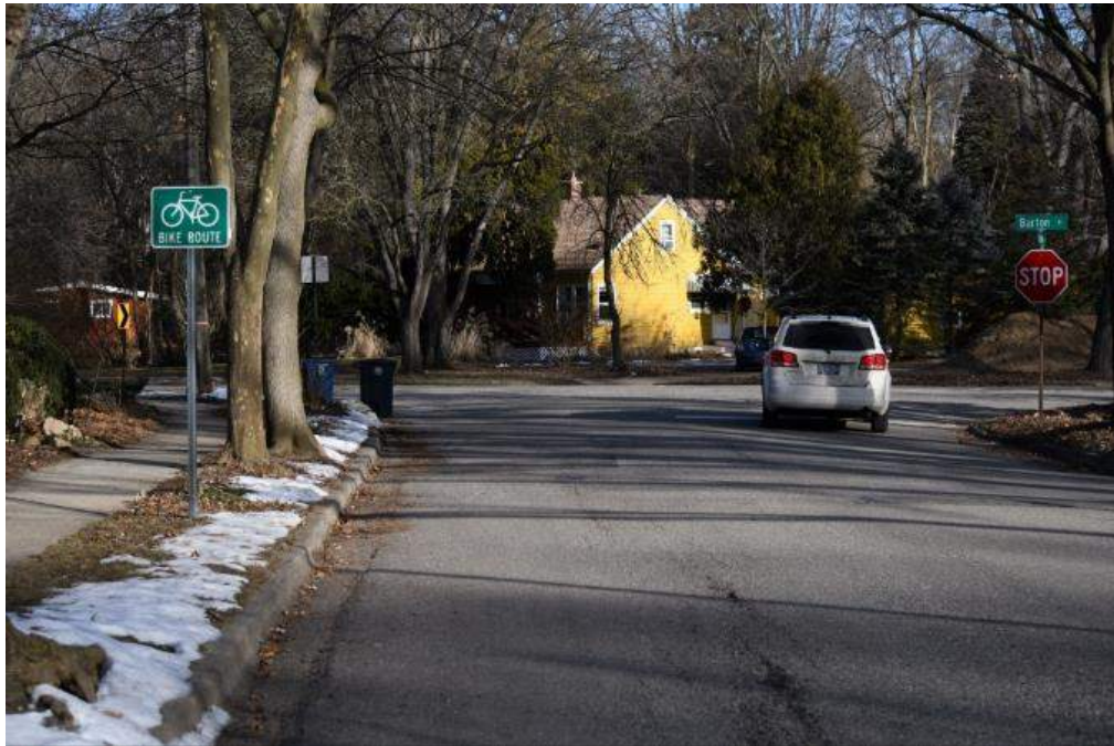
Figure 61: The bike route on Chandler Road does not lead to a bicycle facility and only designates Chandler Road as a safe bicycle street. There are few other signs and the signs are lacking arrows pointing where the bike route continues.
