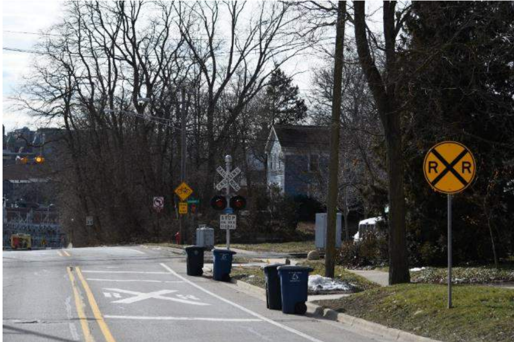
Figure 53: On-street bike lanes lose their utility when blocked by rubbish receptacles or other types of obstructions.
