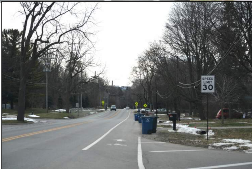
Figure 42: A variety of speed limits are posted along the Pontiac Trail / Pontiac St. The different postings are not commiserate with the roadside environment.
