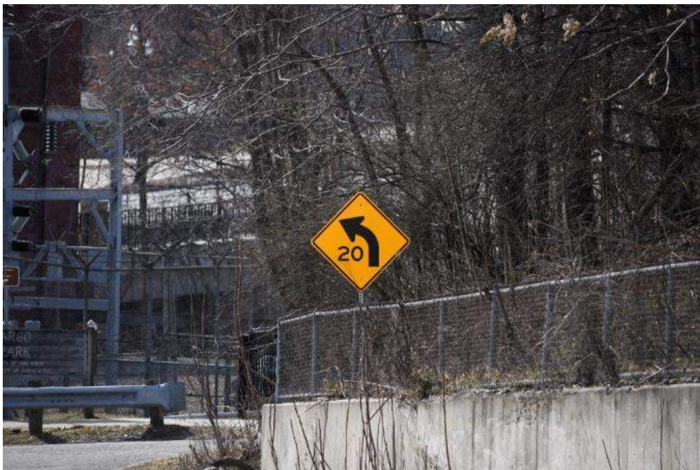
Figure 68: Per MMUTCD, Curve with advisory speed sign (W1-2a) is only to supplement a standard alignment sign with an additional advisory speed plaque (W13-1). In any case, sign is wrong because it combines a curve message with an advisory speed associated with a turn. Curve signs are for speeds 35 mph and above.
