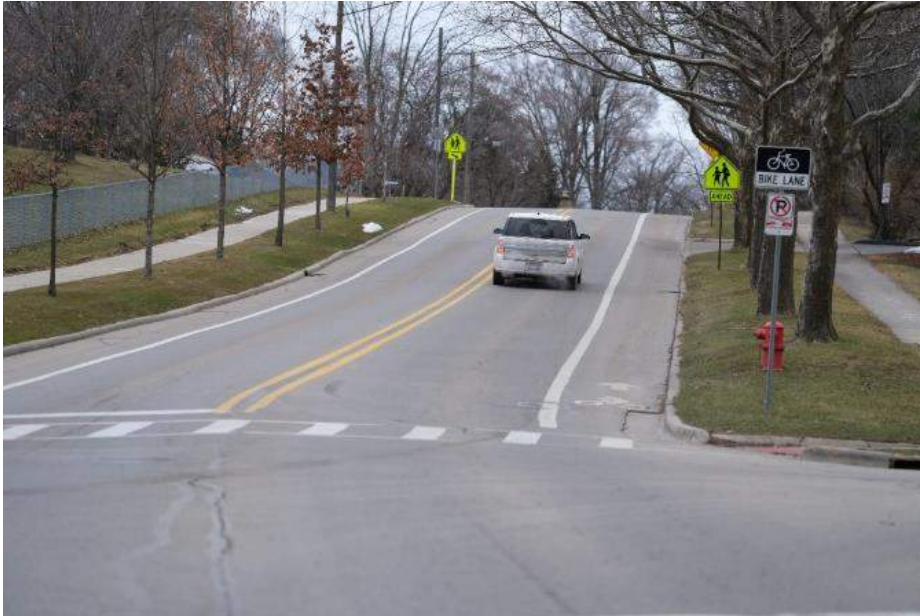
Figure 81: Example of a well maintained pavement markings.
