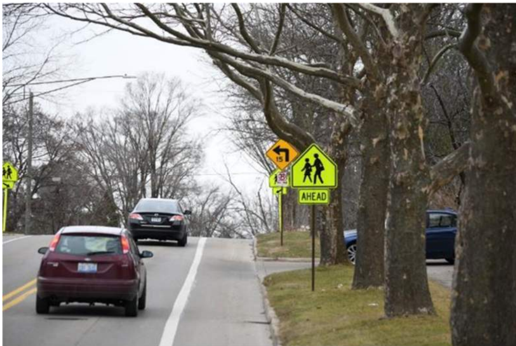
Figure 72: Turn warning sign with advisory speed on Barton Drive, in front of the Northside STEAM school, is poorly located. Should be located just beyond the school pedestrian crossing to not detract from the crossing itself.
