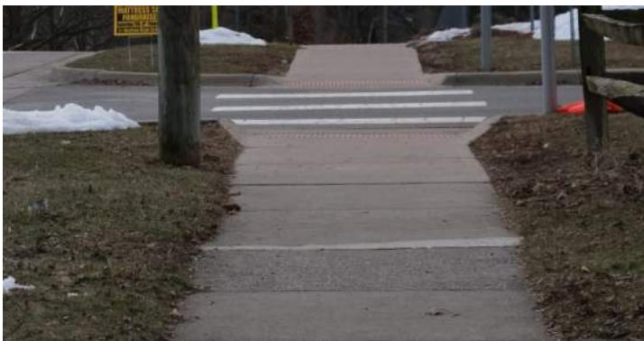
Figure 6: Sidewalks Were Found to be Well Maintained
