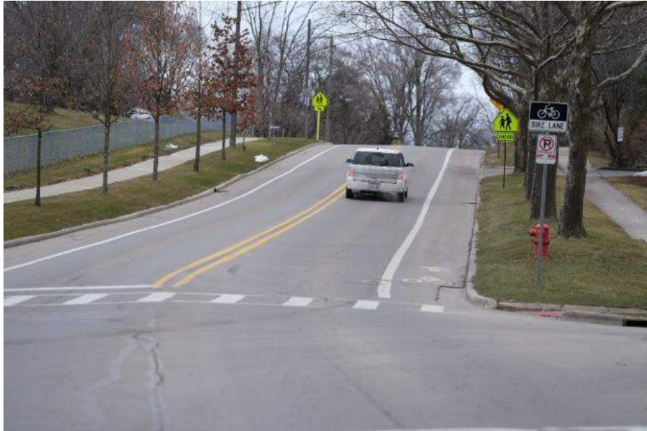
Figure 55: Example of a well dimensioned and signed on-street bike lane.
