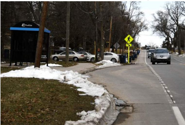
Figure 9: Bus Stop With Shelter At Pull-off Bay
