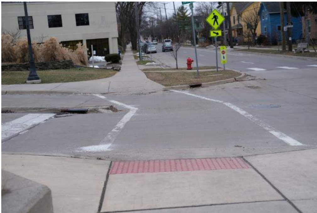
Figure 80: The crosswalk at Detroit Street and Broadway Street/Beakes Street has a deflection mid-crossing, making it non-ADA compliant.
