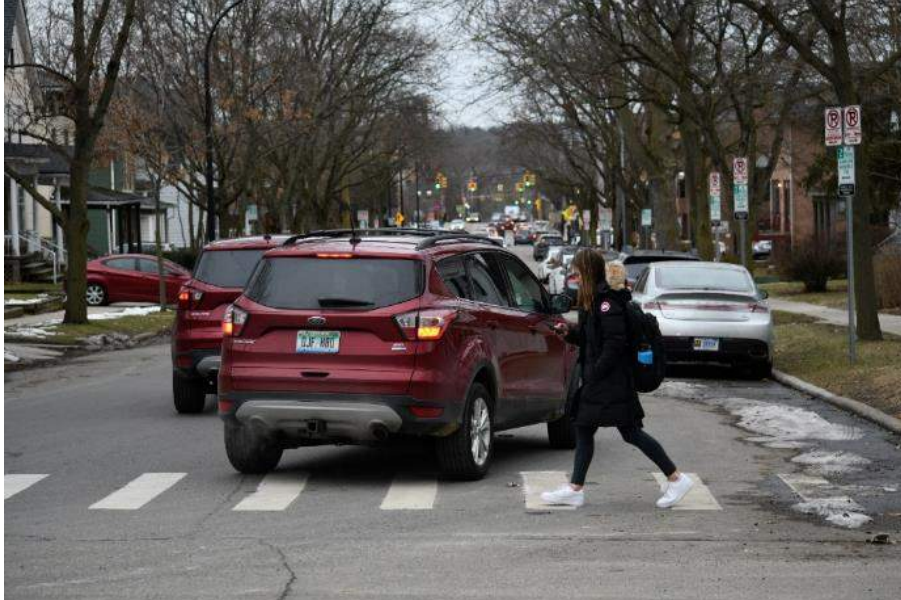
Figure 49: The offset (about 34') between the east and west legs of Catherine St leads to potential conflicts with pedestrians.
