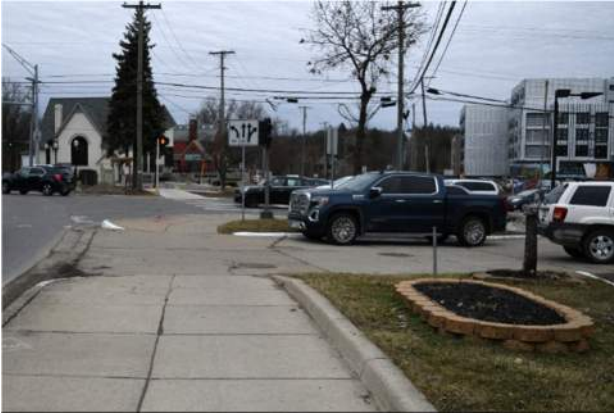
Figure 126: The auto repair shop with access to Broadway Street, Maiden Lane and Wall Street has at least six different curb cuts allowing vehicles to pull in and out of traffic in many places. Some of these driveways are blocked by parked cars throughout the day and should be considered for closure.
