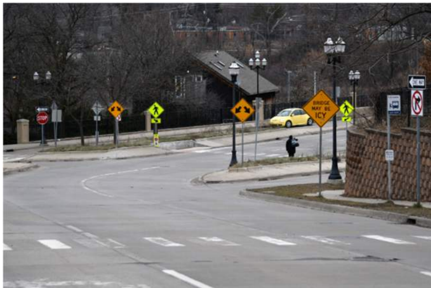
Figure 102: Vehicle speeds are also high as NB Division turns onto Broadway. This, combined with limited sight distance, raises concerns for pedestrians crossing the roadways.
