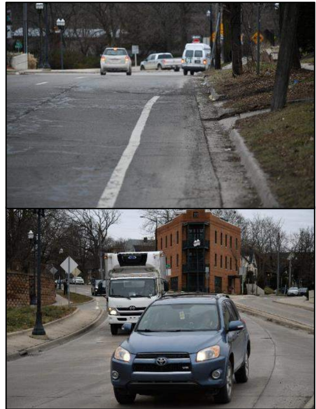
Figure 37: Geometric constraints related to NB Division St joining Broadway St. Dedicated On-street bike lane ends just prior to start of steep down-grade and sharp horizontal curve.
