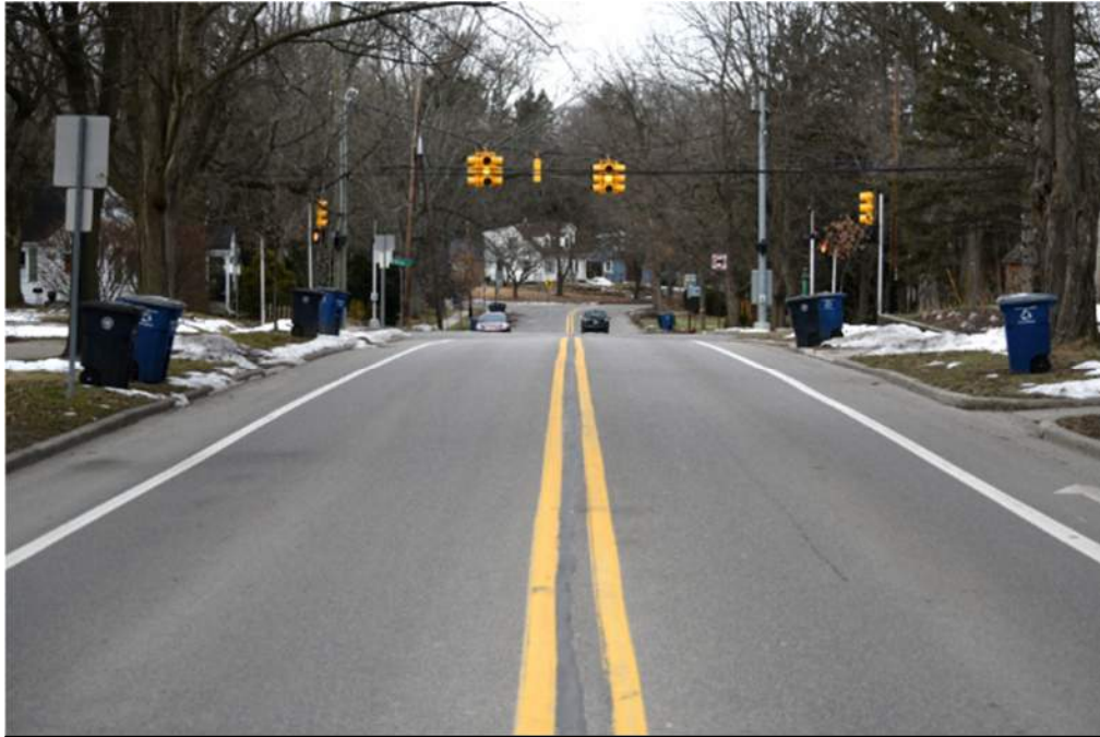
Figure 69: No horizontal alignment warning sign for westbound Barton Drive west of Pontiac Trail.
