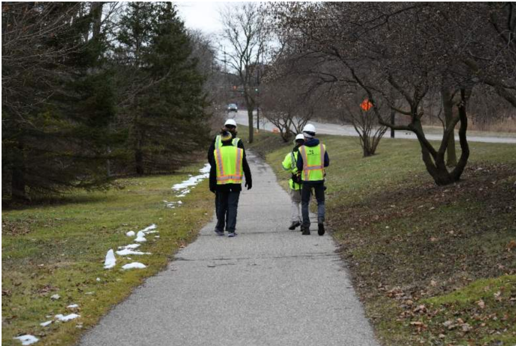
Figure 124: Side path in the depressed section along Plymouth Road does not get much light from streetlights and could use path level lighting.
