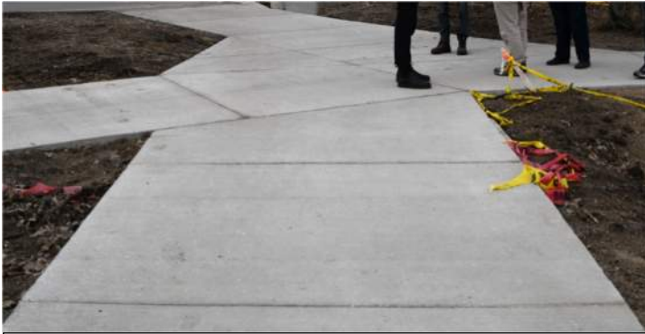
Figure 5: Sidewalk Recently Replaced
