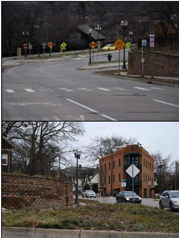
Figure 36: Retaining wall as sight distance obstruction. Top view as seen by drivers NB on Division; bottom view as seen by pedestrians.
