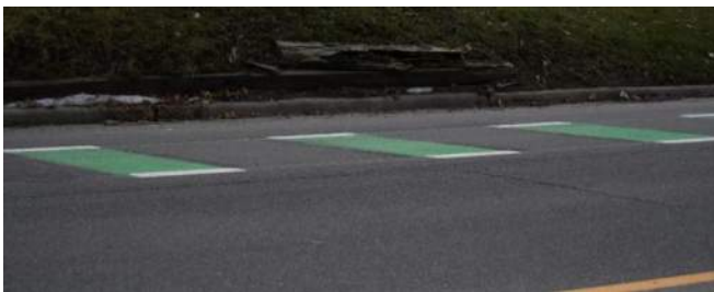
Figure 4: Delineated Bike Lanes Through Turn Lanes
