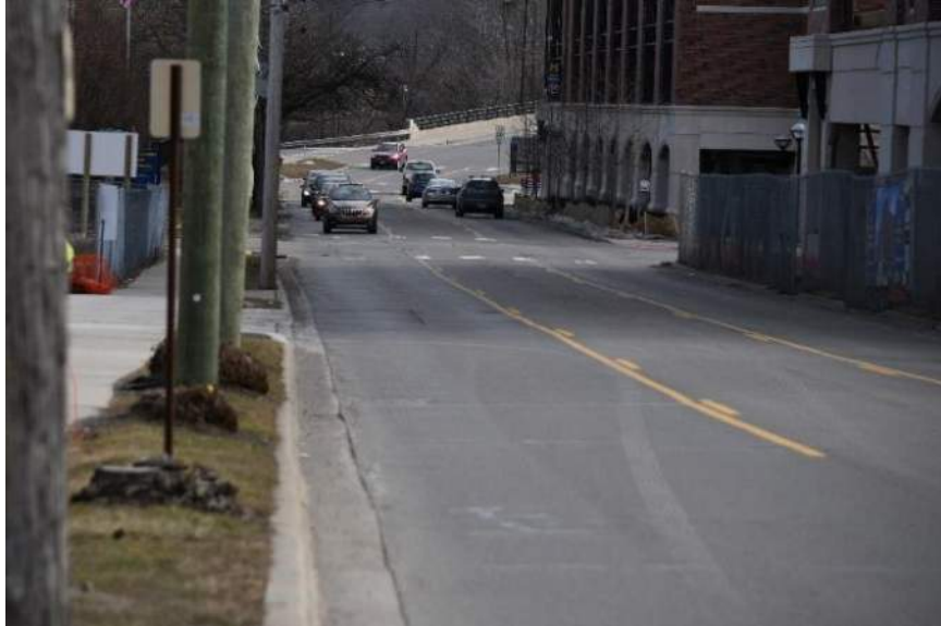
Figure 96: Maiden Lane – Typical section is 3 vehicle lanes, no parking allowed, no bike lanes, sidewalk both sides, overhead utilities along north side.
