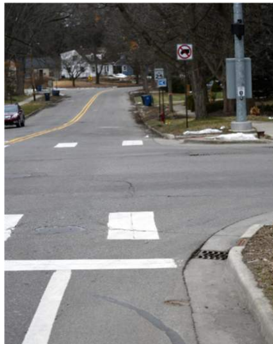
Figure 58: At the intersection of Barton Drive and Pontiac Trail, the bike lanes on Barton Drive west of the intersection do not continue and no guidance is provided for bicyclists.
