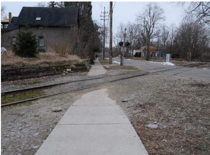
Figure 22: Sidewalk Does Not Continue Through Railroad Crossing
