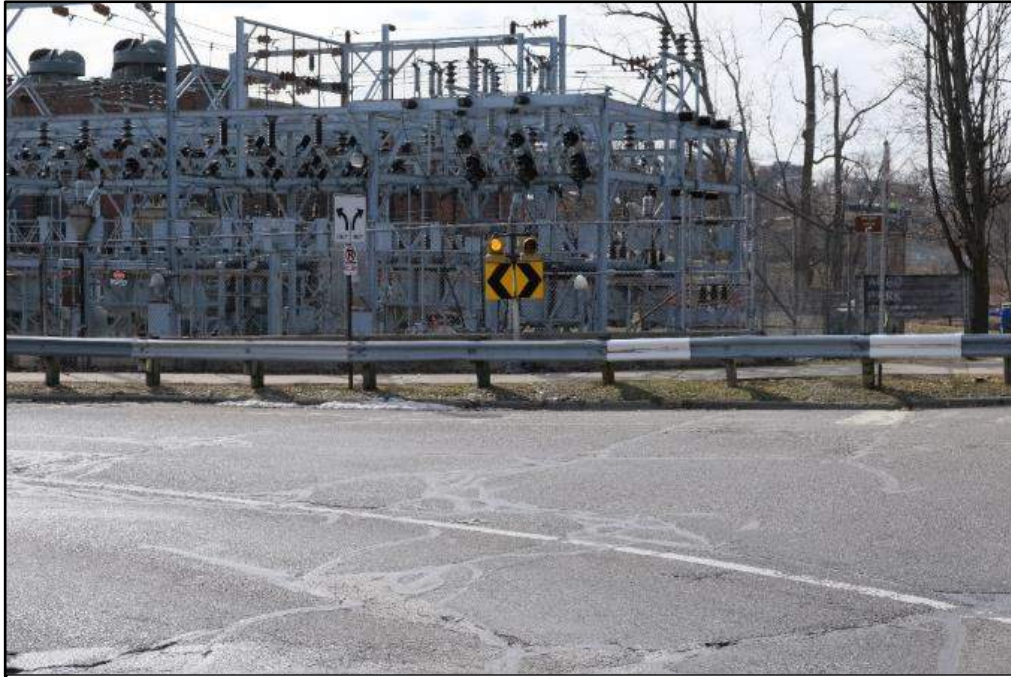
Figure 67: Chevron signs at Swift Street and Pontiac Street are improper. Should be a Two-direction Large Arrow (W1-7).
