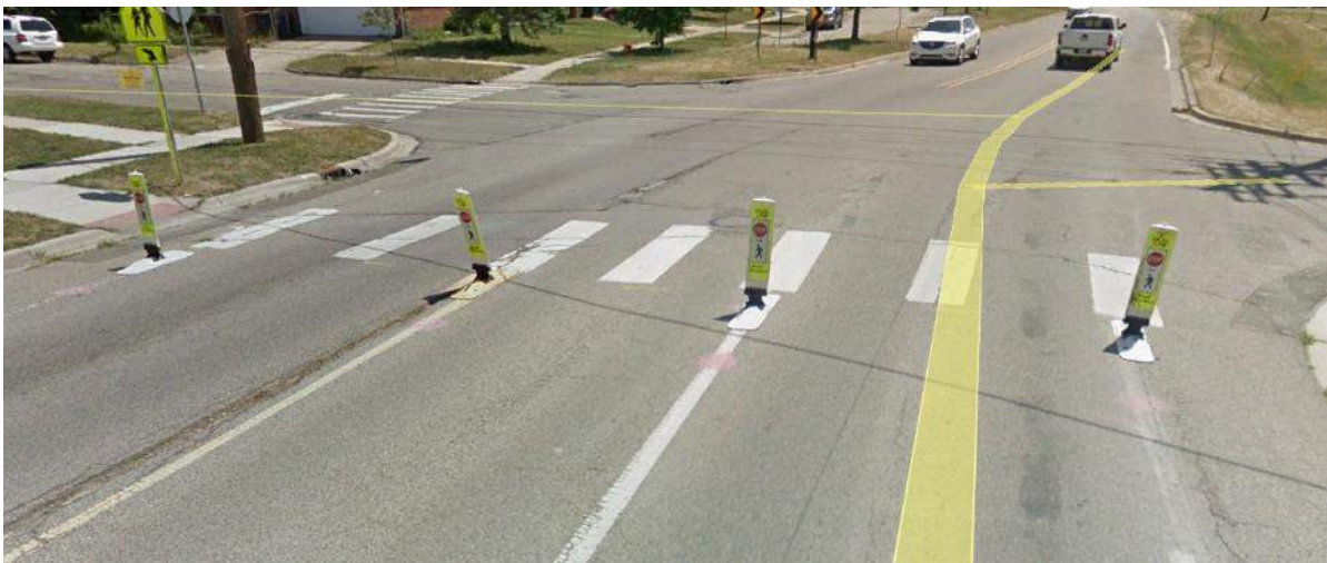
Figure 39: Example of using R1-6 in-road signs on a multi-lane road as a gateway treatment.
