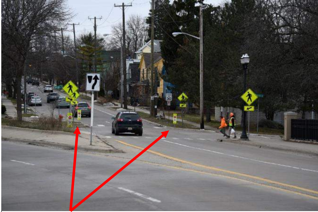
Figure 71: R1-6 signs need to be placed in the road on the lane line or in a pedestrian island per the MMUTCD.
