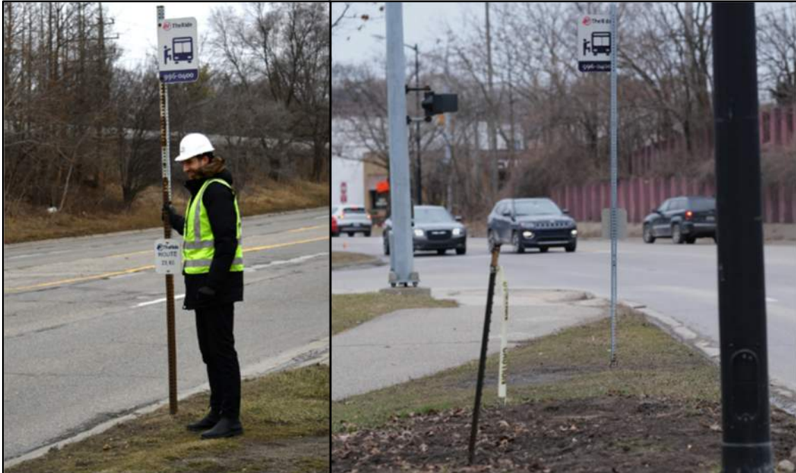
Figure 32: Example of Bus Stop Without a Landing Pad or Connection to Sidewalk/Pathway
