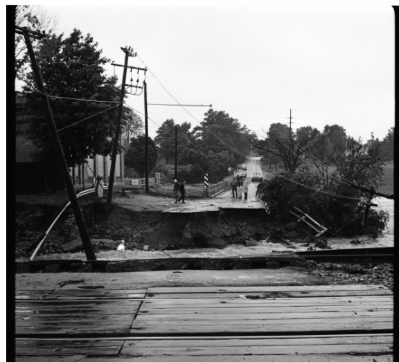
Figure 15: Washed-out bridge from 1968 Allen Creek flood
