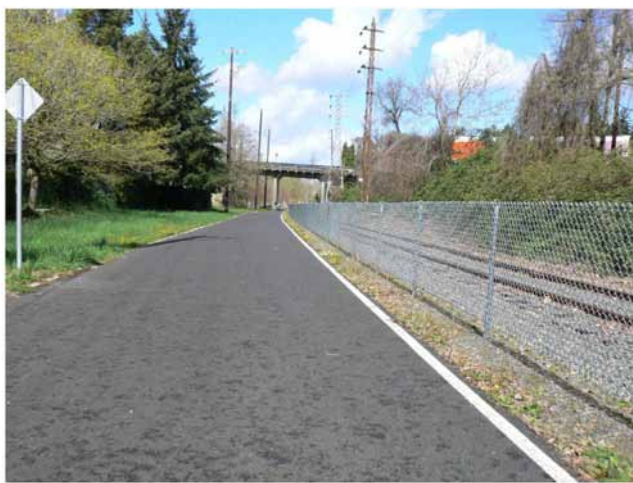
Figure 11: Separation of a greenway from railroad tracks by fence
